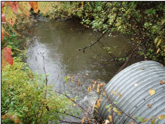
Figure 74. Strawberry Creek culvert outlet. View downstream from outlet.
