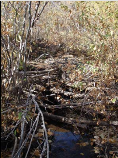
Figure 43. Johnny David Creek culvert inlet. View upstream from culvert inlet.
