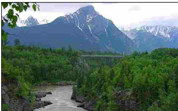
Figure 8. Hagwilget Canyon upstream of bridge.
