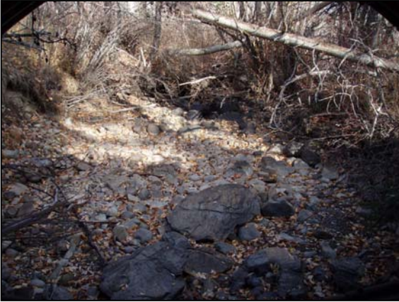
Figure 68. Coffin Creek culvert outlet. View downstream from outlet.
