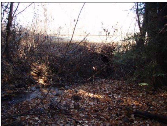
Figure 39. Moan Creek culvert inlet. View downstream to culvert inlet
