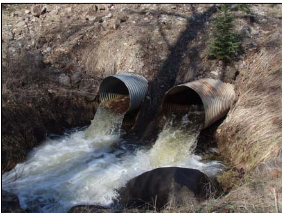
Figure 58. Tyhee Creek culvert outlets. View upstream of outlets in spring, 2007.
