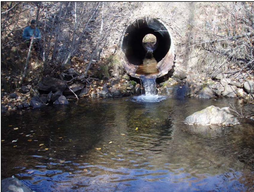
Figure 41. Johnny David Creek culvert outlet. View upstream of culvert outlet.
