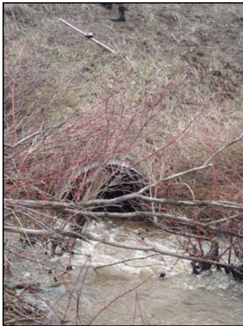
Figure 55. McDowell Creek culvert inlet. View downstream to culvert inlet.
