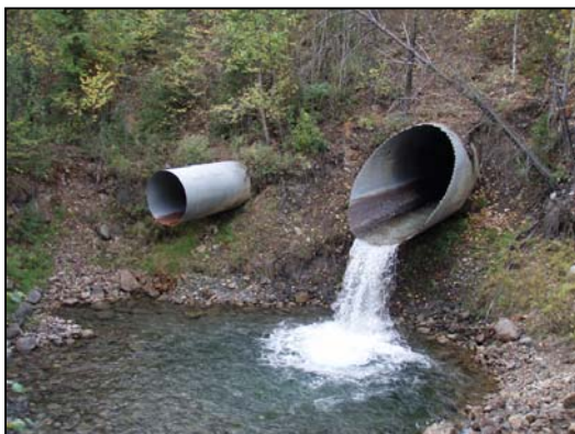
Figure 2. View upstream of Porphyry Creek culvert outlet
