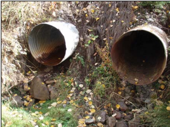
Figure 57. Tyhee Creek culvert outlets. Outlets in late September, 2006.
