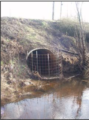
Figure 48. Glass Creek culvert inlet. View downstream to culvert inlet.
