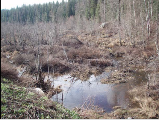
Figure 47. Glass Creek culvert inlet. View upstream from culvert inlet.
