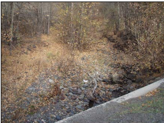
Figure 64. Cesford Creek culvert inlet. View upstream from inlet.
