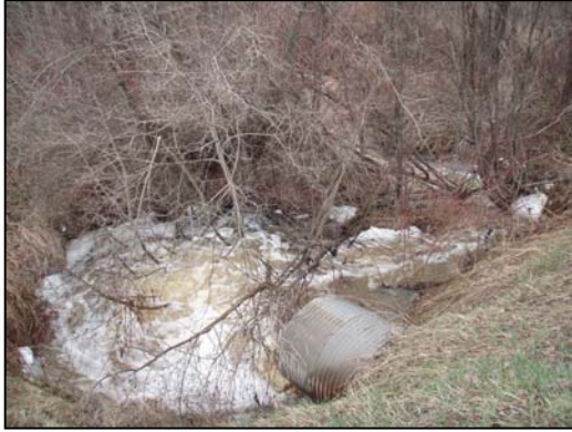
Figure 53. McDowell Creek culvert outlet. View downstream of culvert outlet.
