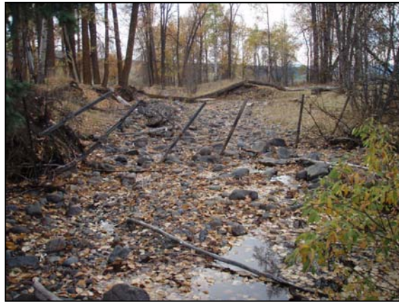
Figure 63. Cesford creek culvert outlet. View downstream from outlet.
