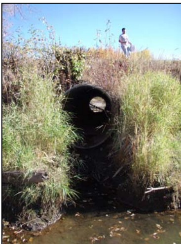
Figure 36. Bulkley Oxbow 1 culvert outlet. View upstream of culvert outlet.
