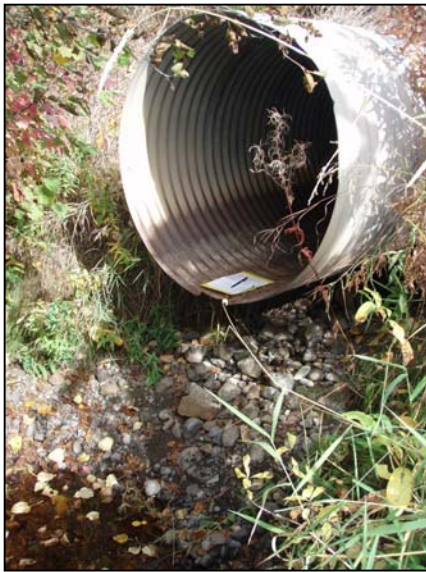
Figure 51. McDowell Creek culvert outlet. Photo shows late summer dry flows.
