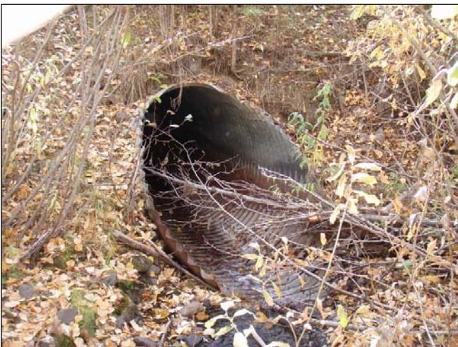
Figure 44. Johnny David Creek culvert inlet. View downstream to culvert inlet.
