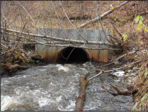
Figure 30. Station Creek culvert inlet. View downstream to inlet.
