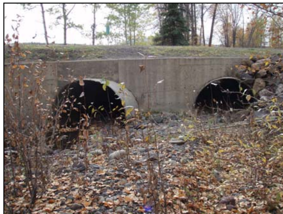
Figure 65. Cesford creek culvert inlet. View downstream to inlet.
