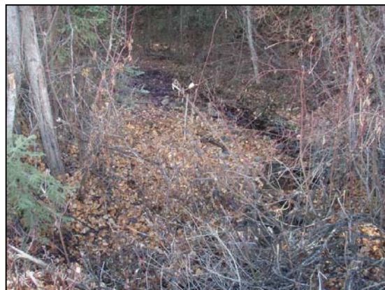
Figure 40. Moan Creek culvert inlet. View upstream from culvert inlet
