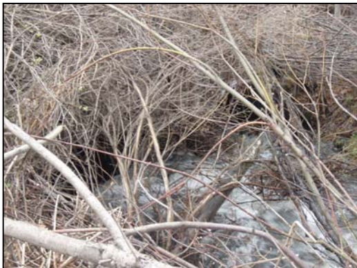
Figure 61. Tyhee Creek culvert inlet. View downstream to inlet.
