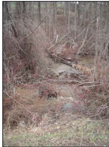
Figure 56. McDowell Creek culvert inlet. Channel upstream of culvert inlet.
