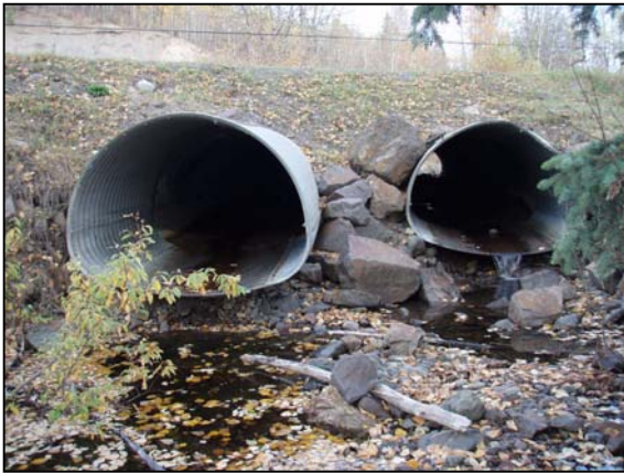
Figure 62. Cesford Creek culvert outlet. View upstream to inlet.
