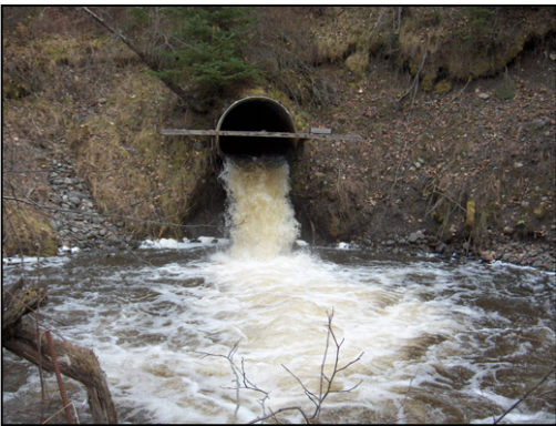
Figure 32. Station Creek culvert outlet. View upstream of outlet.
