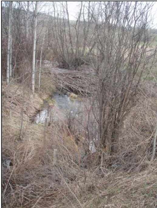
Figure 60. Tyhee Creek culvert inlet. View upstream to inlet.
