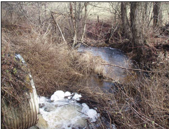
Figure 46. Glass Creek culvert outlet. View downstream from culvert outlet.
