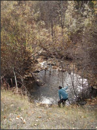
Figure 42. Johnny David Creek culvert outlet. View downstream from culvert outlet.
