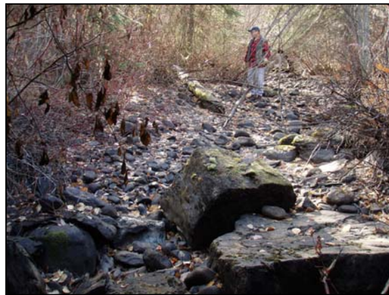
Figure 71. Coffin Creek culvert inlet. View upstream from inlet.
