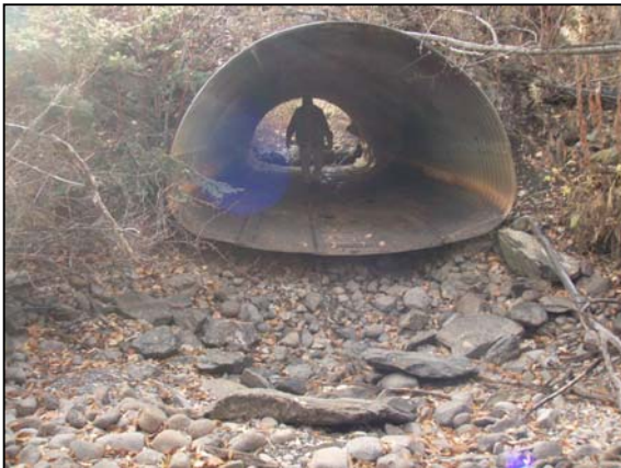
Figure 66. Coffin Creek culvert outlet. View upstream to outlet.
