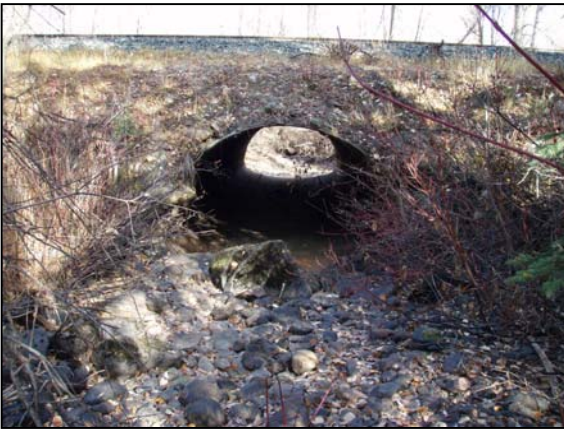
Figure 70. Coffin Creek culvert inlet. View downstream from outlet.
