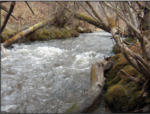
Figure 31. Station Creek culvert inlet. View upstream from inlet.
