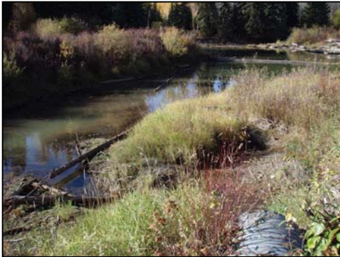
Figure 35. Bulkley Oxbow 1 culvert outlet. View downstream of oxbow channel.
