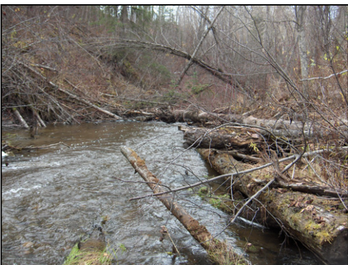
Figure 33. Station Creek culvert outlet. View downstream from outlet.
