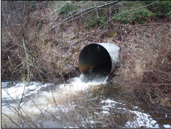
Figure 72. Strawberry Creek culvert outlet. View upstream to outlet in high flows.
