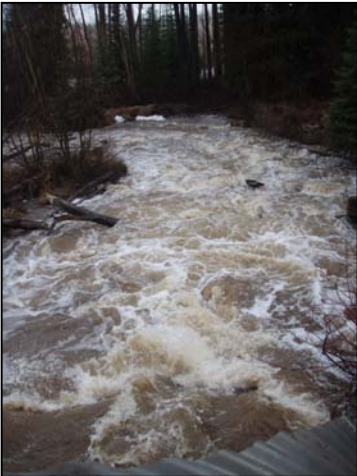
Figure 28. View of Toboggan Creek culvert outlet. Photo shows high flow conditions May 04, 2007.
