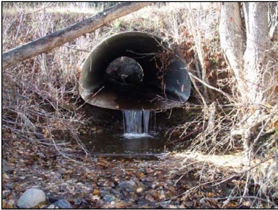
Figure 37. Moan Creek culvert outlet. View upstream of culvert outlet.
