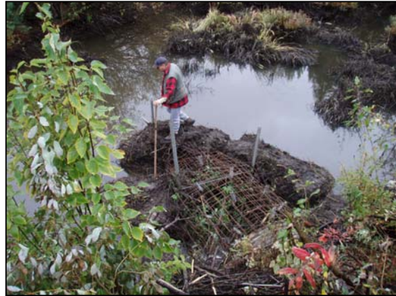
Figure 73. Strawberry Creek culvert inlet.
