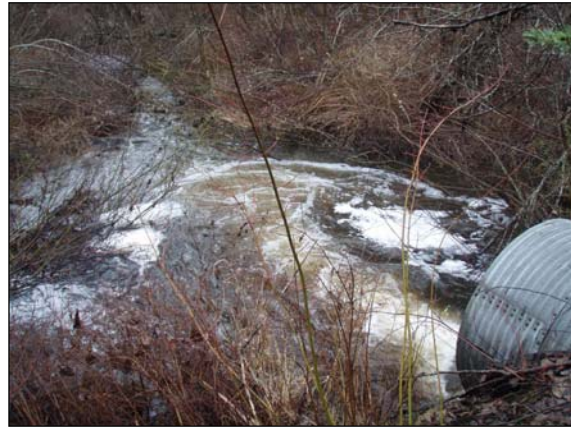
Figure 75. Strawberry Creek culvert outlet. View downstream from culvert in high flows.
