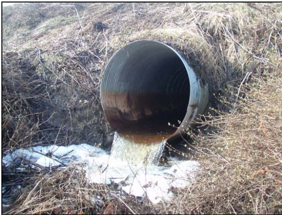
Figure 45. Glass Creek culvert outlet. View upstream of culvert outlet.
