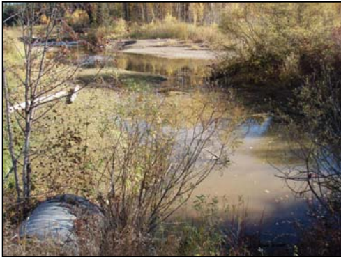
Figure 34. Bulkley Oxbow 1 culvert inlet. View upstream.
