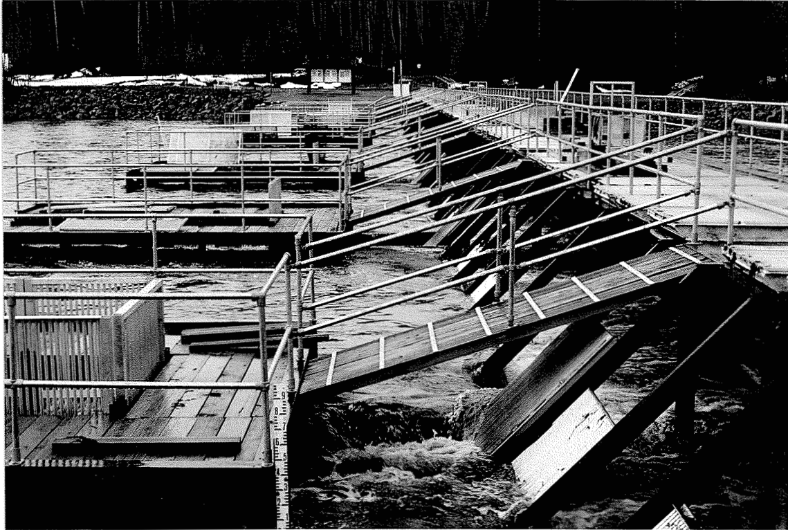
Figure 10. Photograph of fence on May 18 th , when discharge overflowed the new fence panels by approximately 10 cm.
