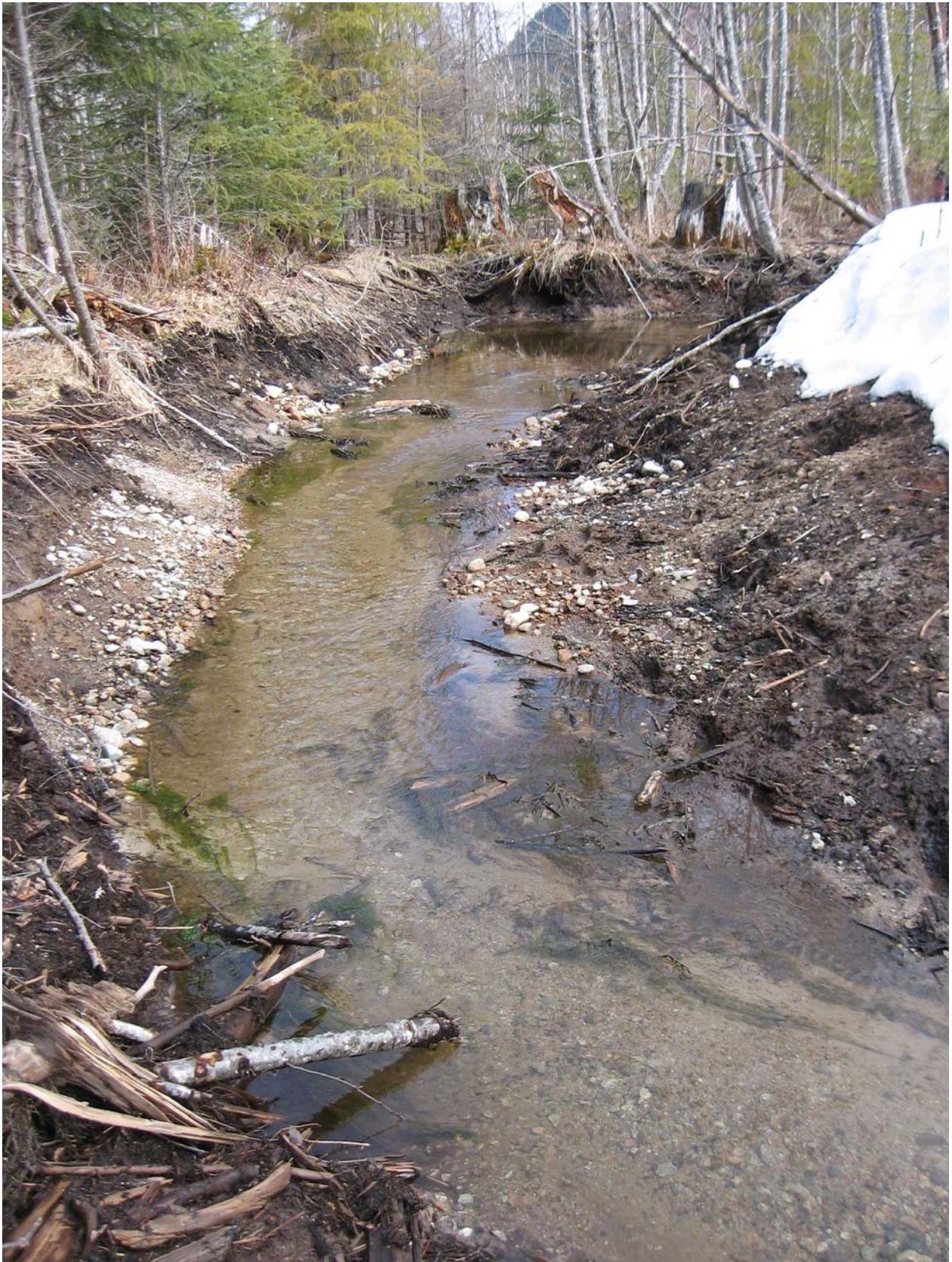
Figure 10. This photo shows natural gravel deposits encountered during channel excavation.
