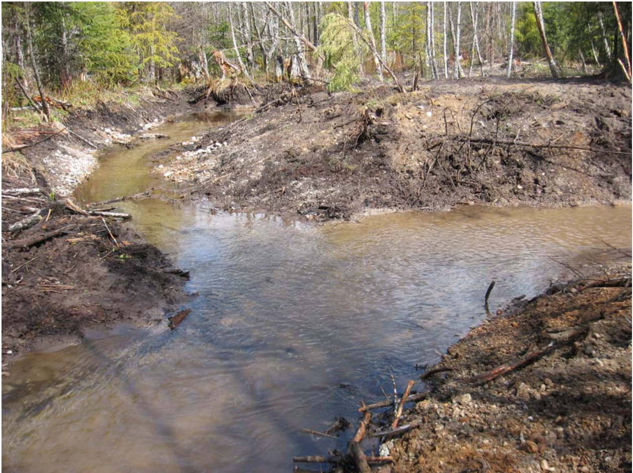
Figure 13. The newly excavated channel (May 2007) flows in the groundwater channel excavated in November 2006, doubling flows.
