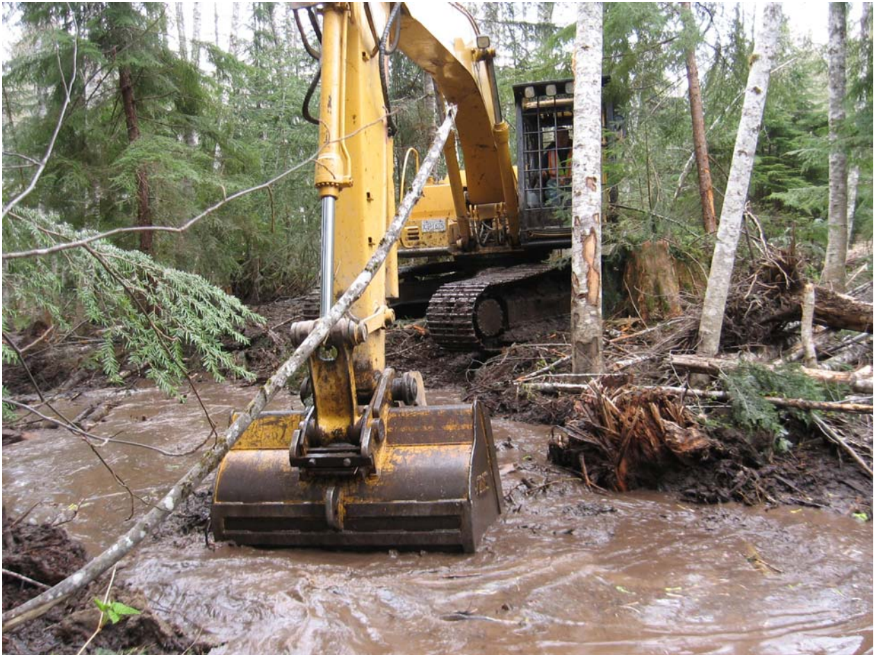
Figure 8. Fine sediment removal in the downstream end of the groundwater channel.
