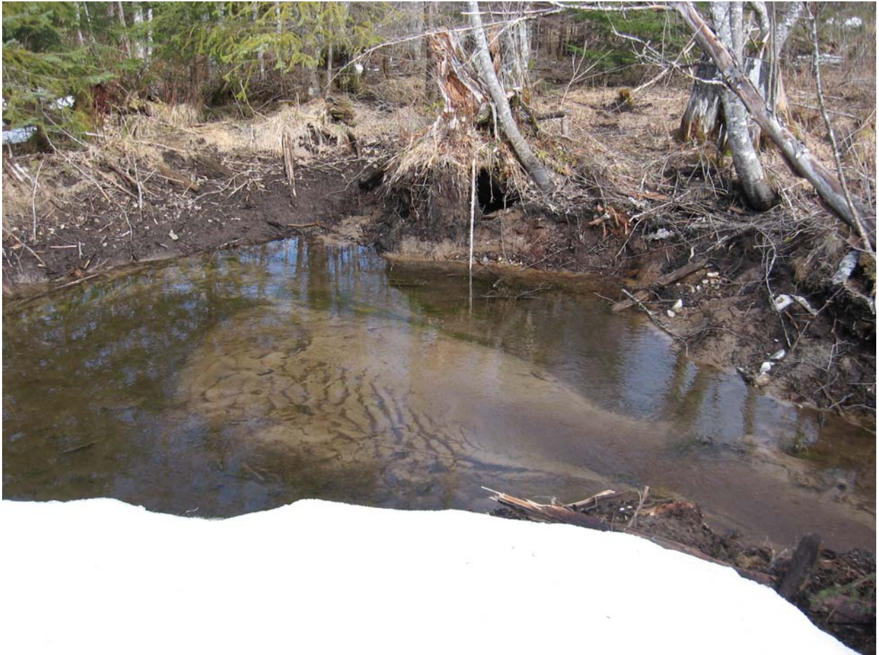
Figure 11. A pool constructed in an area of fine sediment in November, 2007, has infilled with sediment.
