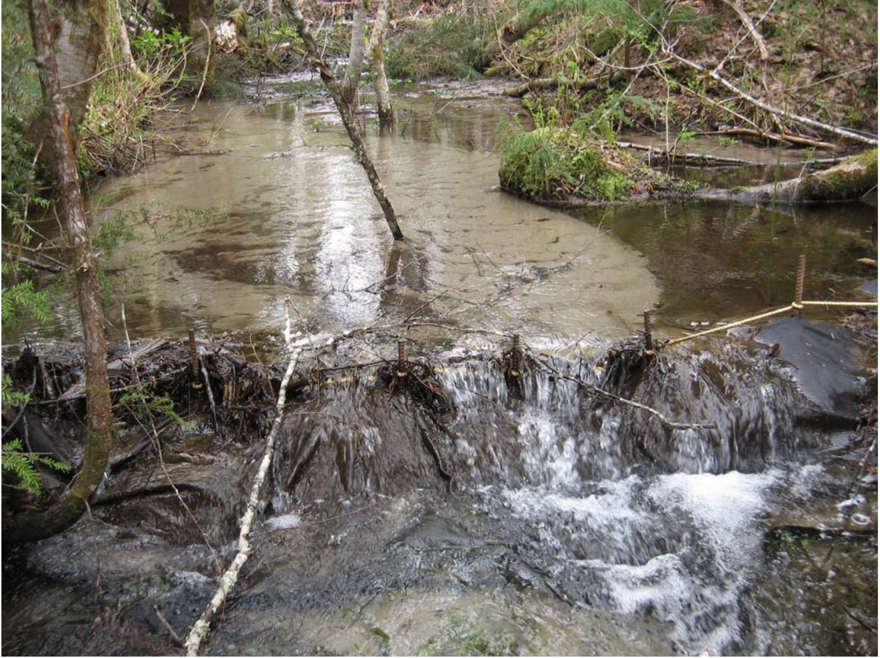
Figure 5. One of three silt fences installed with accumulated sediment Trapped upstream.
