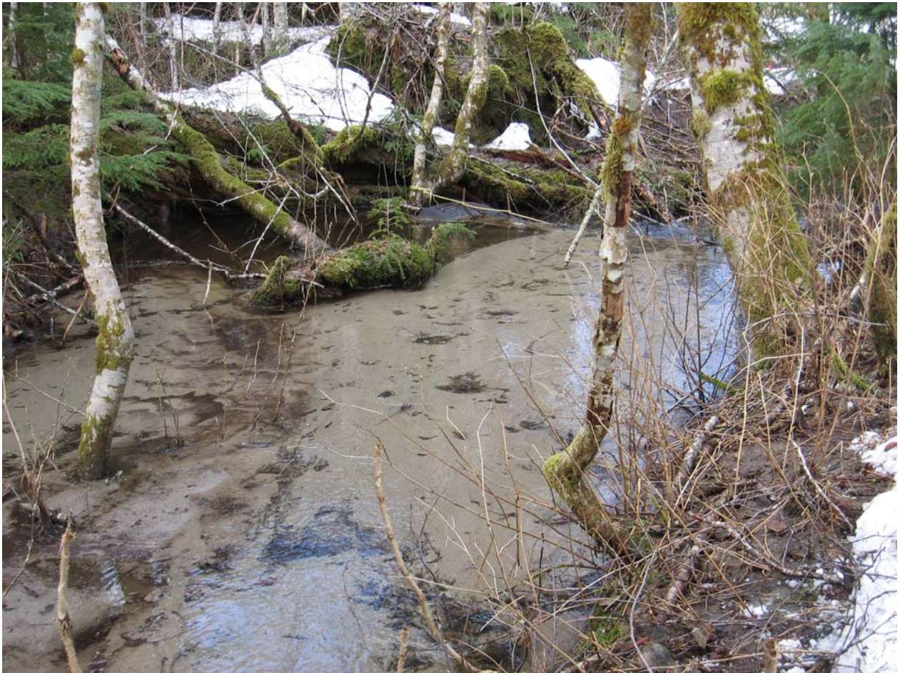
Figure 12. April 2007 site visit. Accumulated sediment upstream from the three sediment fences at the downstream end of the groundwater channel.
