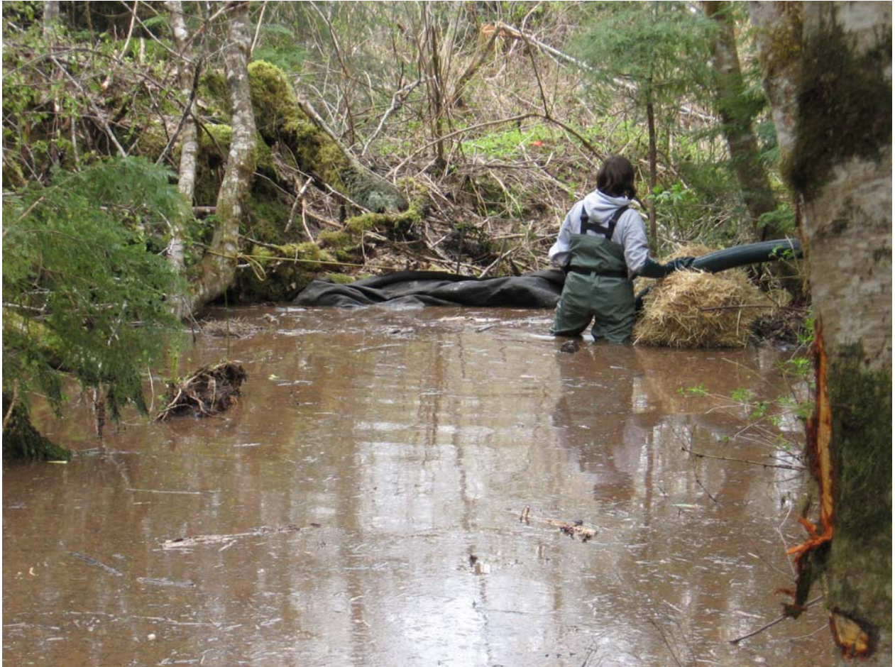
Figure 4. Installation of a silt fence to trap sediment during construction.
