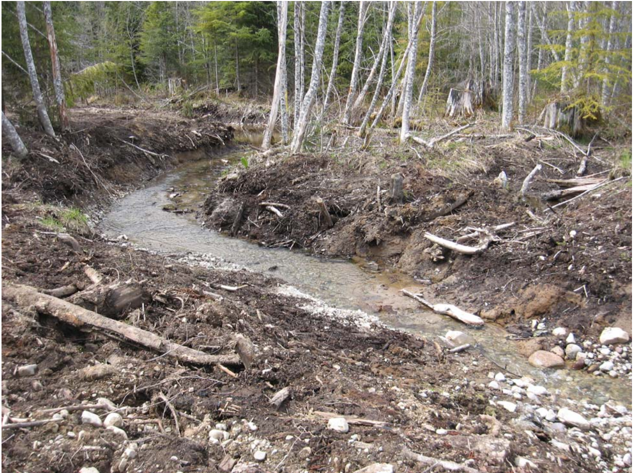
Figure 6. Excavated channel with disturbed banks requiring seeding and planting.
