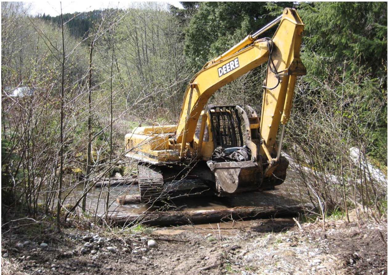
Figure 3. An excavator crosses Scully South on three access logs for May 2007 construction work.
