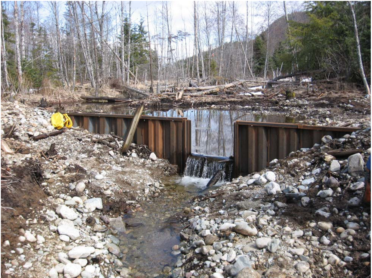
Figure 9. Installed sheet pile dam with two stop logs in place.
