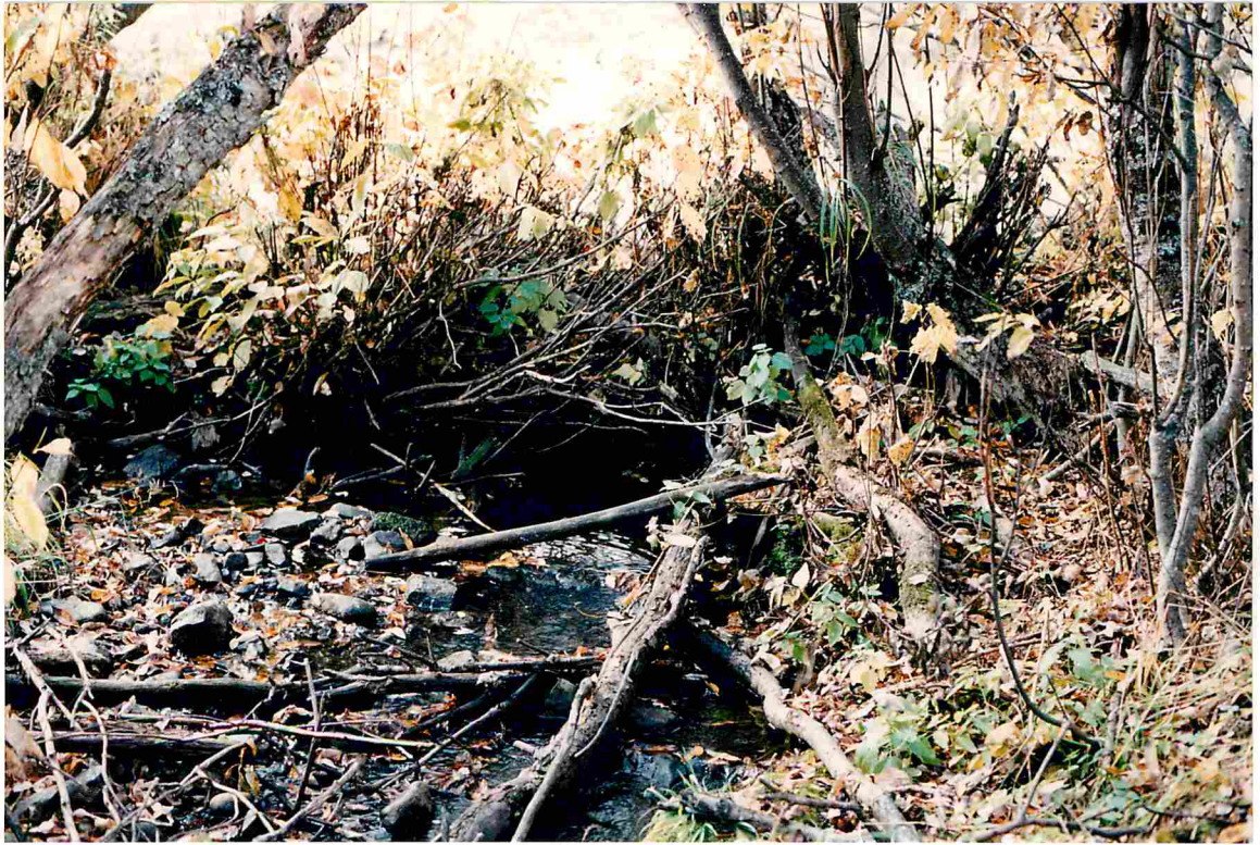
Figure 9. One of three leaks in the beaver dam of outlet stream.
