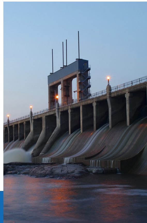
Seven Sisters Generating Station, Winnipeg River, MB
