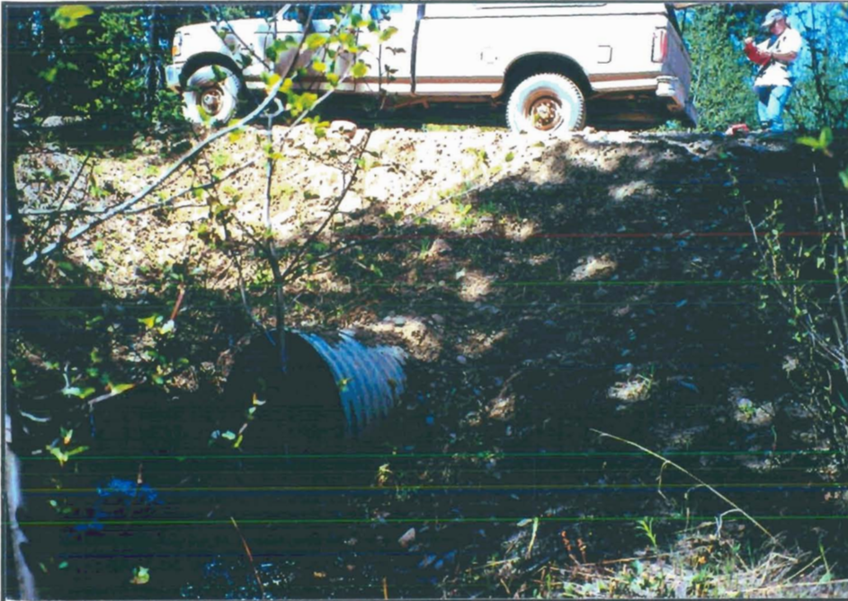
Photo 97. Tagit C. Tributary Ta7, R1, Road culvert.
