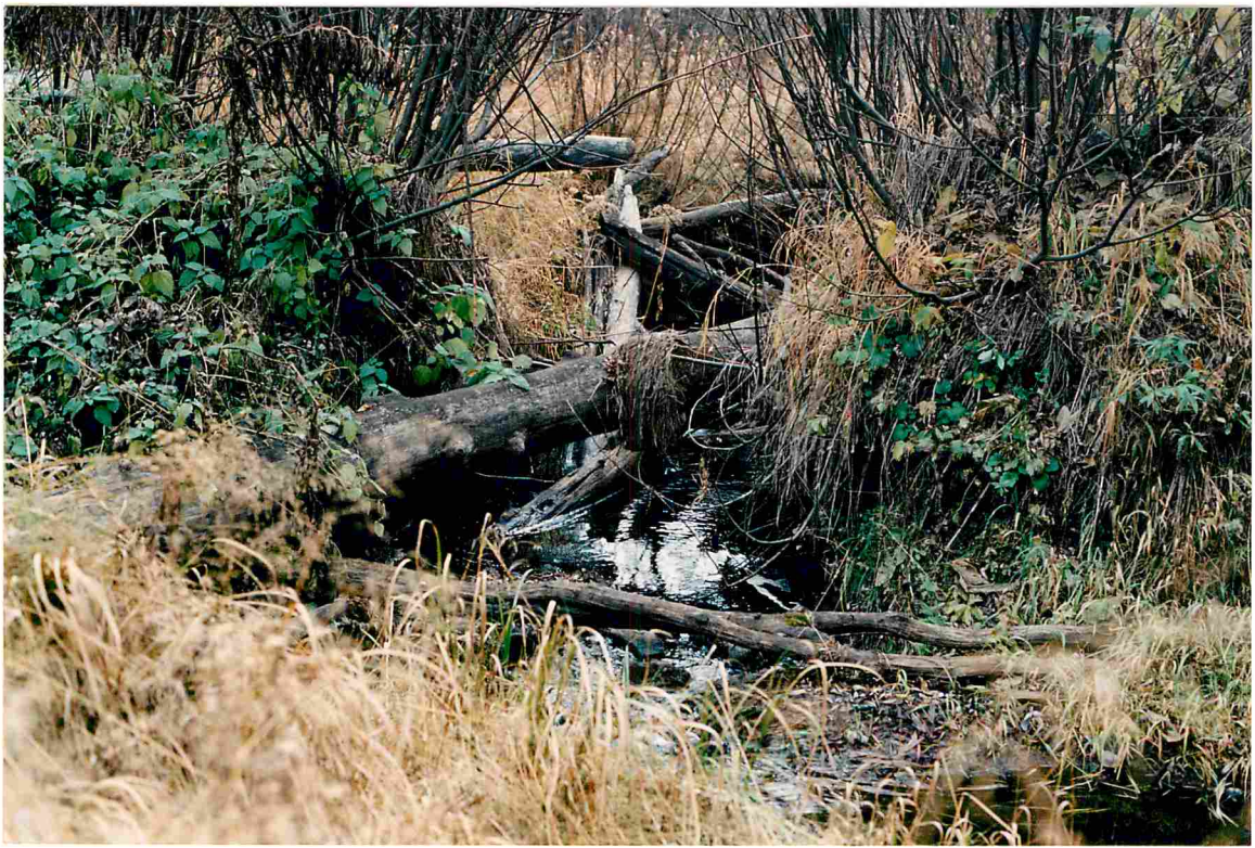
Figure 4. Washout at first beaver dam on outlet stream from Swan Lake.
