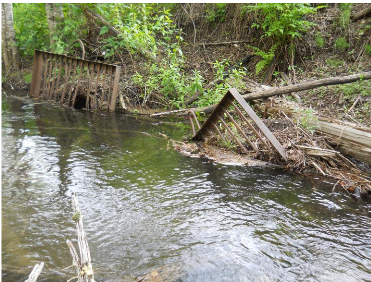
Figure 7.3: Fish and water can no longer pass properly through these streams. (Photo: Marc Porter)
