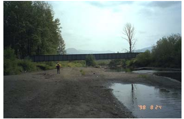
Plate #113: CN railway crossing aggraded section of reach (sediment wedges) approximately 2500 metres upstream of the 1/2 reach break.
