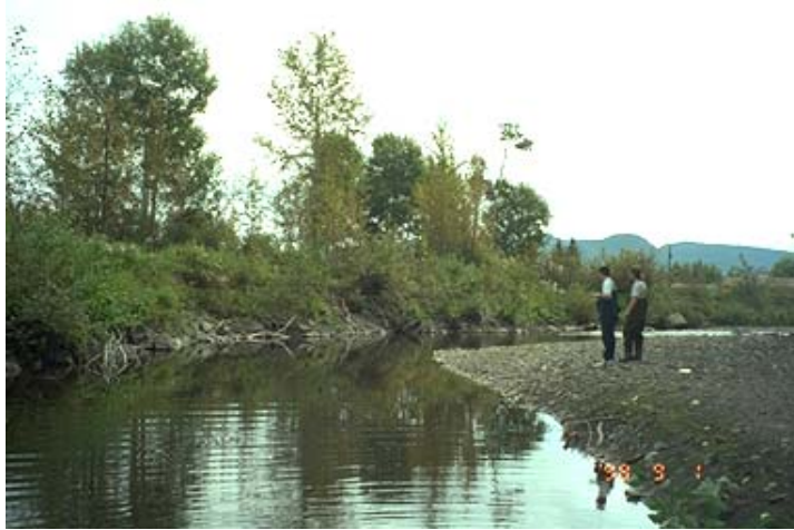
Plate_: Dyking on one side of the channel in the lower half of the reach, resulting in stream channelization.
