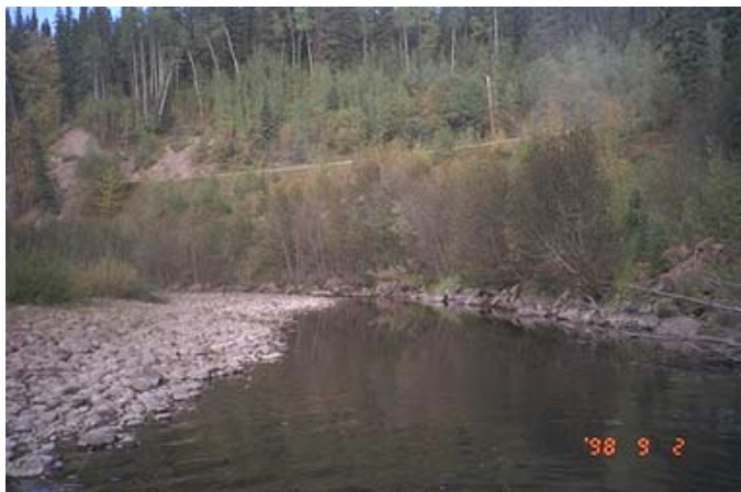
Plate 73: Rip-rap bank channelizing at 4700 metres upstream of the 3/4 reach break, where the Buck Flats Road parallels the creek.
