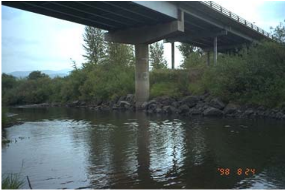
Plate #112: Downstream view of the rip-rapped Highway 16 bridge crossing (east of Houston), channelizing that section of the reach.
