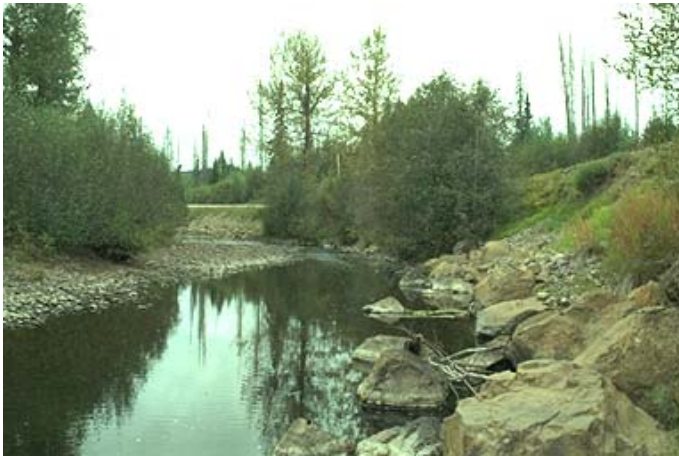
Plate #87: Rip-rapped channelized section of the reach where the Buck Flats Road parallels the creek located 2750 metres upstream of the 5/6 reach break.
