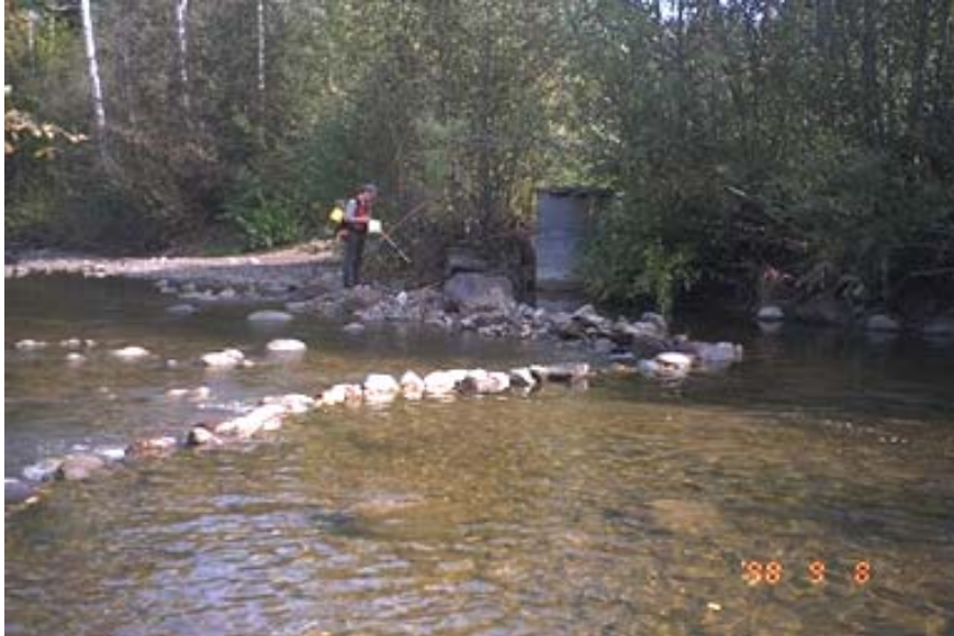
Plate 64: Intersecting powerline corridor crossing the creek between 550-600 metres upstream of the 1/2 reach break. Rocks and boulder have been placed to allow for water at the pump house.
