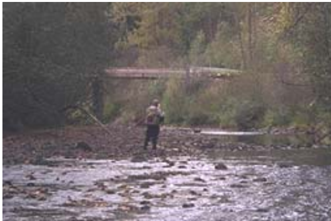
Plate 72: Buck Creek Bridge #1 located at 4100 metres upstream of the 3/4 reachbreak.
