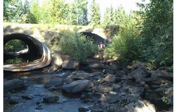
Plate #_ : Double pipe-arch culverts under Highway 16. Flow is consistent through only one culvert during periods of low flow.
