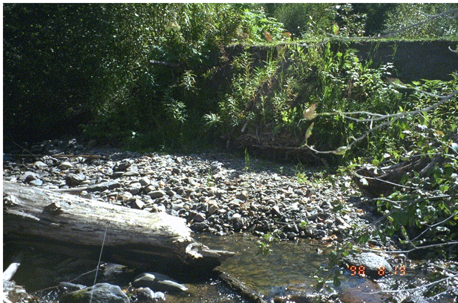
Plate #53: Bank erosion at site of old private bridge site.
