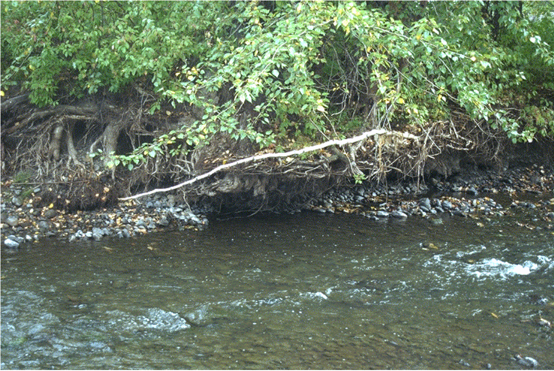
Plate #123: Bank erosion occurring at the head of CN rip-rapped section approximately 440 metres upstream of the 2/3 reach break.
