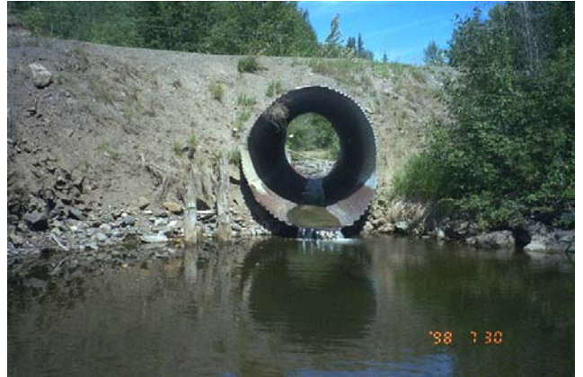
Plate # 9: Highway culvert, with gradient of upto 3%.
