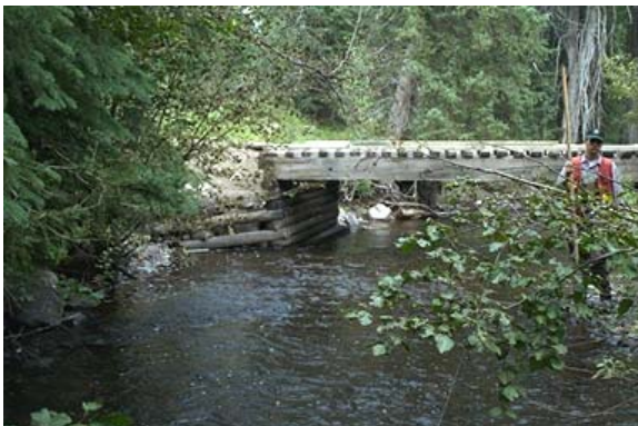
Plate #_: Second upstream bridge crossing, located in the upper reach.
