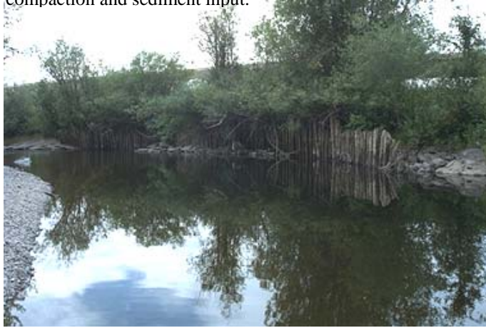
Plate #102: Flood protection dyking occurring mid reach (just upstream of the Highway 16 bridge enforcements) contributing to stream channelization.
