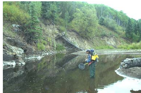
Plate #77: Section of heavy sediment wedge deposits, exposed bedrock, and eroding clay banks 2340 metres upstream of the 4/5 reach break.
