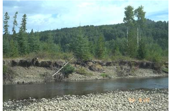
Plate #96: Outside bank erosion seen below area of historically cleared land in the lower end of the reach.
