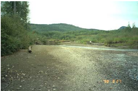
Plate #108: Aggraded channel, extensive bank erosion and minimal riparian forest seen above the Knockholt Bridge.
