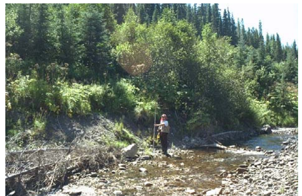
Plate #20: Bank erosion below the North Road, 1000 metres upstream of the 2/3 reach break.
