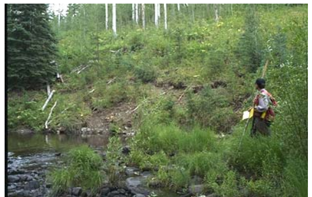
Plate #94: Road related bank slumpage occurring in the upper half of the reach.
