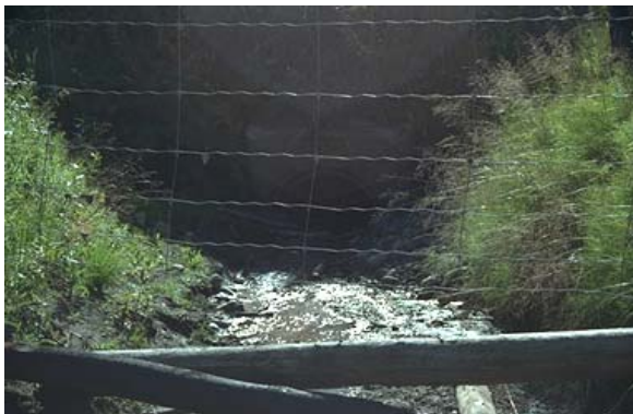
Plate_: Downstream view of railway culvert 28 metres upstream of the Barren/Bulkley confluence. The remainder of the reach runs through private ranch lands.
