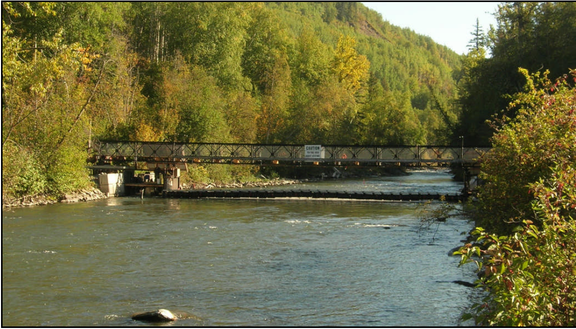
Photograph #2: Upstream view of the KSEF, September 13, 2007.
