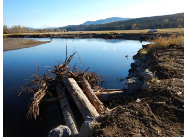
Photo 32. Bulkley River at McKilligan Rd (Lower) – Looking upstream from just below 0+000 m after construction (2 October 2016).
