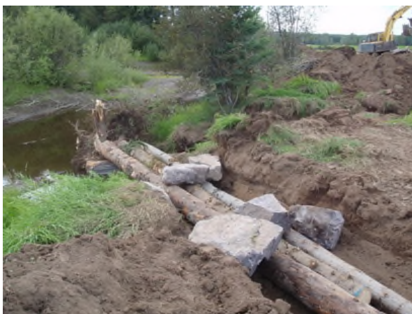
Photo 4. Lower Maxan Creek – Three upstream-facing logs and ballast rocks in a trench at 0+055 m during construction (13 August 2016).
