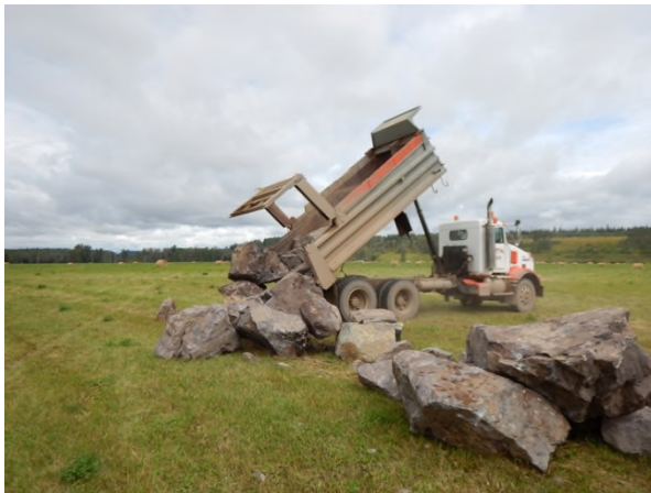
Photo 2. Lower Maxan Creek – High-lift dump truck delivering ballast rocks for LWD structures (9 August 2016).
