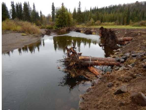
Photo 16. Bulkley River at Groot Farm – Looking downstream from ~0+085 m after construction (25 September 2016).
