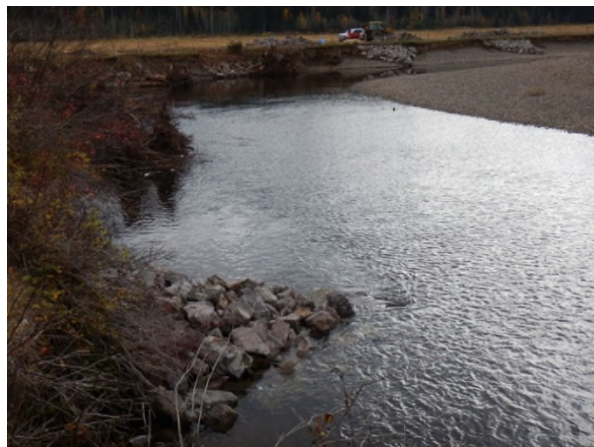
Photo 18. Bulkley River at McKilligan Rd (Upper) – Looking downstream from 0+295 m after construction (5 October 2016).
