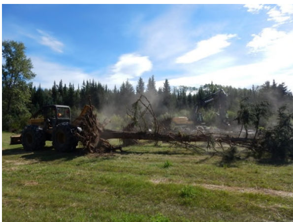
Photo 3. Lower Maxan Creek – John Deere skidder transporting a log with rootwad attached to the site from a nearby area (12 August 2016).
