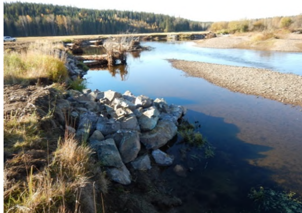
Photo 28. Bulkley River at McKilligan Rd (Lower) – Looking downstream from 0+165 m after construction (2 October 2016).
