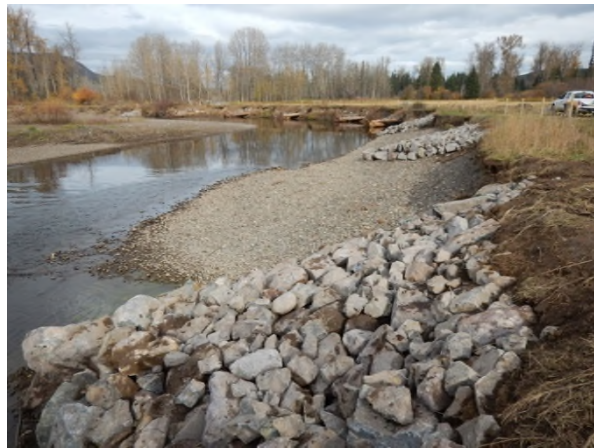
Photo 22. Bulkley River at McKilligan Rd (Upper) – Looking upstream from 0+134 m after construction (5 October 2016).
