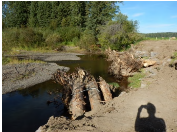
Photo 10. Lower Maxan Creek – Looking upstream from 0+080 m after construction (19 August 2016).
