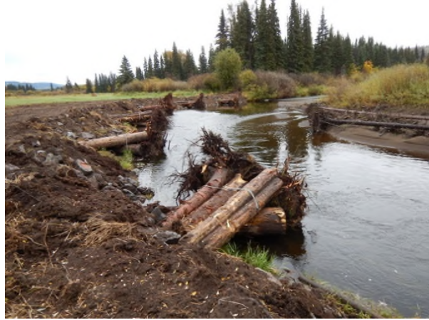
Photo 14. Bulkley River at Groot Farm – Looking upstream from just below 0+000 m after construction (25 September 2016).
