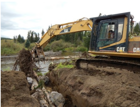
Photo 11. Bulkley River at Groot Farm – An excavator placing a log with rootwad attached in a trench at 0+030 m (8 September 2016).
