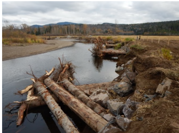
Photo 24. Bulkley River at McKilligan Rd (Upper) – Looking upstream from 0+000 m after construction (5 October 2016).
