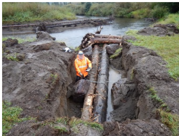
Photo 12. Bulkley River at Groot Farm – Securing ballast rocks to logs using epoxy and 12.7 mm diameter cable at 0+015 m (7 August 2016).
