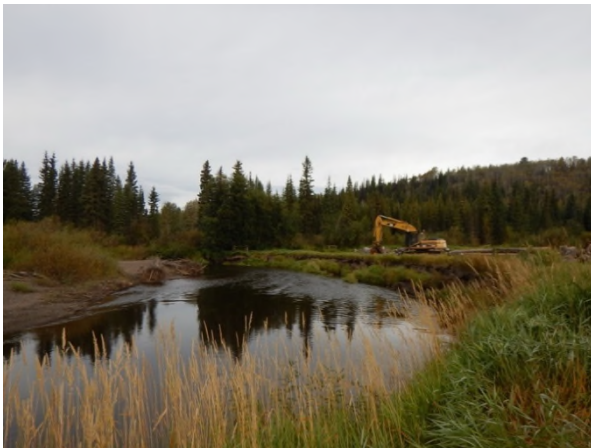
Photo 15. Bulkley River at Groot Farm – Looking downstream from ~0+085 m before construction (7 September 2016).
