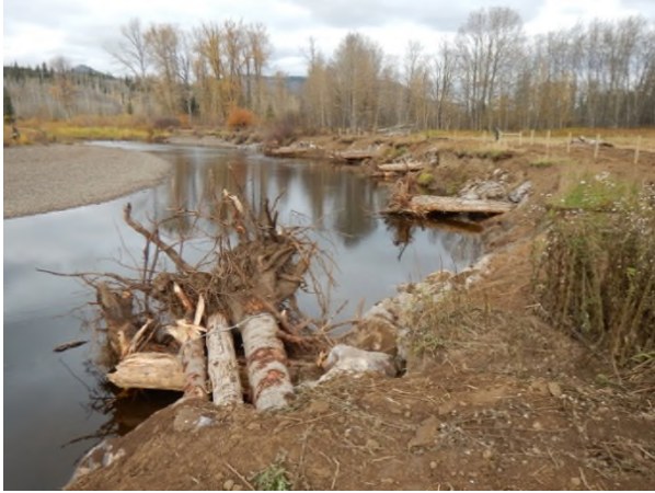
Photo 19. Bulkley River at McKilligan Rd (Upper) – Looking upstream from 0+192 m after construction (5 October 2016).
