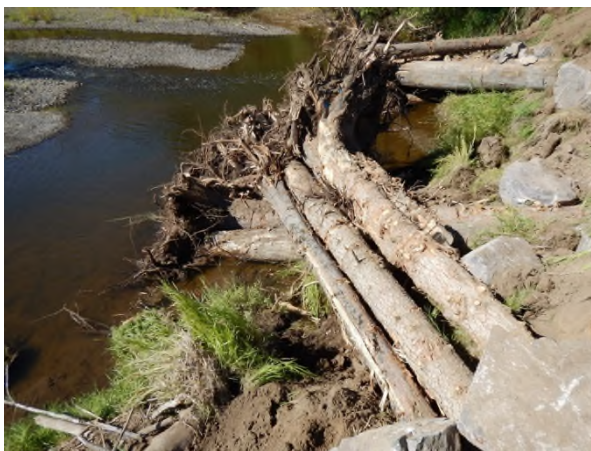
Photo 6. Lower Maxan Creek – Looking upstream at the LWD structure at 0+085 m after construction (14 August 2016).
