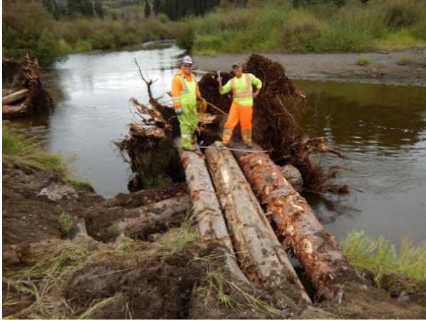
Photo 13. Bulkley River at Groot Farm – Looking upstream at a LWD structure at 0+045 m after construction (9 September 2016).
