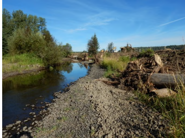
Photo 8. Lower Maxan Creek – Looking upstream from 0+000 m after construction (19 August 2016).
