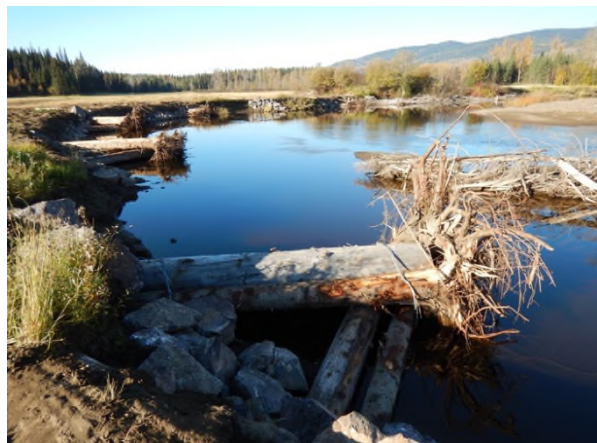
Photo 30. Bulkley River at McKilligan Rd (Lower) – Looking downstream from 0+100 m after construction (2 October 2016).
