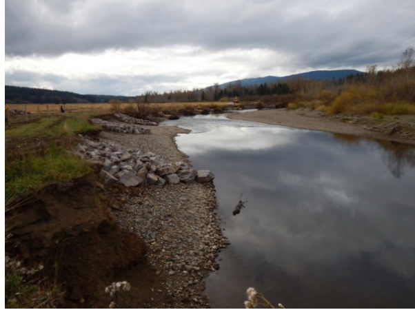
Photo 20. Bulkley River at McKilligan Rd (Upper) – Looking downstream from 0+192 m after construction (5 October 2016).
