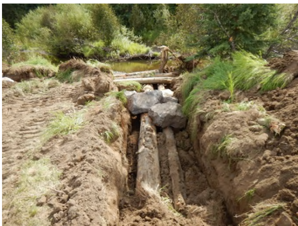
Photo 5. Lower Maxan Creek – Two downstream-facing logs and ballast rocks in a trench at 0+055 m during construction (13 August 2016).
