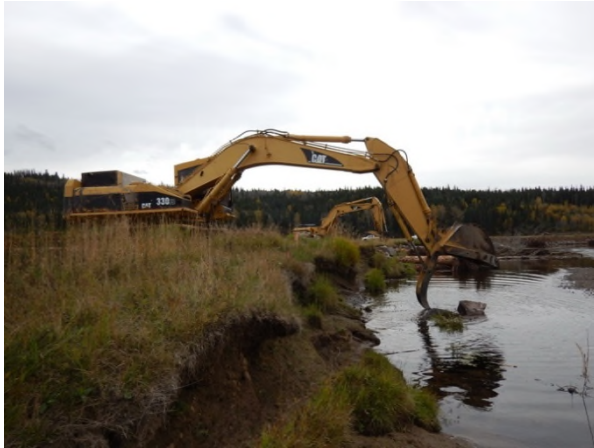
Photo 25. Bulkley River at McKilligan Rd (Lower) – Looking downstream at an excavator constructing a rock groin at 0+287 m (24 September 2016).
