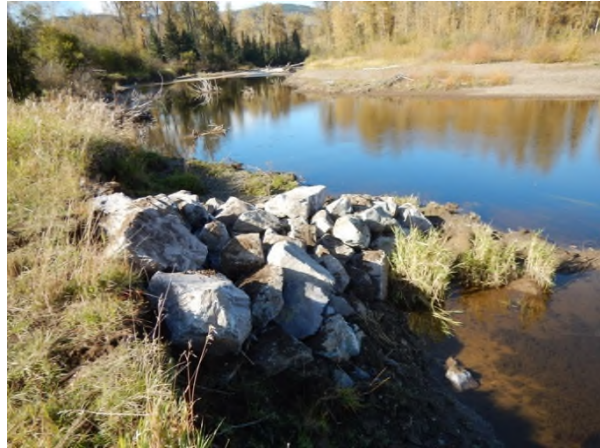
Photo 26. Bulkley River at McKilligan Rd (Lower) – Looking downstream at the rock groin at 0+018 m after construction (23 September 2016).
