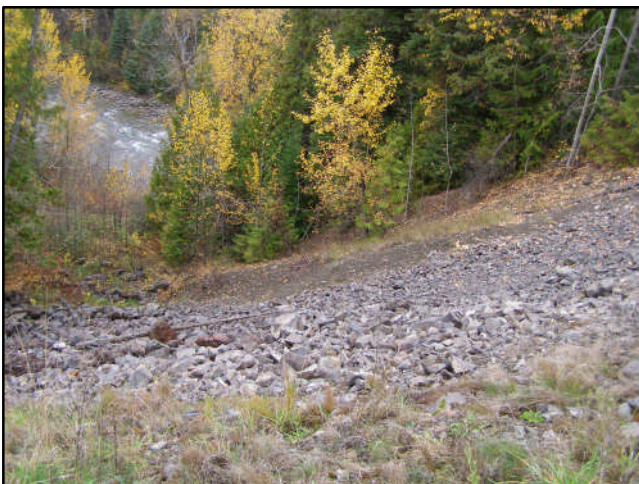
Figure 107. View across the lower portion of Slide 3 that received a rock blanket.
