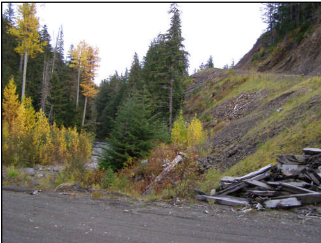
Figure 111. View downstream from bridge on West Kitsuns Creek. Slim Jim Road (aka: W7 Branch, Kitsuns 701) ascends the hill on the right. Much of the right streambank has slid into the creek and was subsequently covered with rock blankets.
