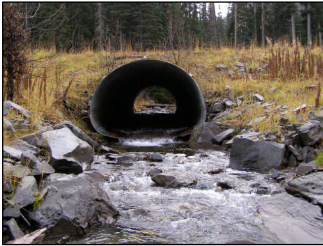
Figure 93. View is upstream to culvert outlet.
