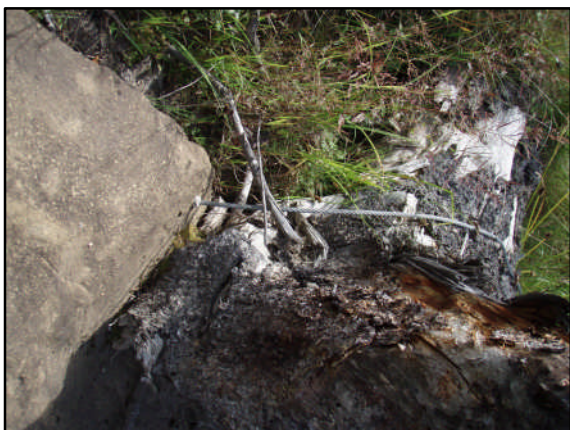
Figure 14. Log-boulder cabling.
