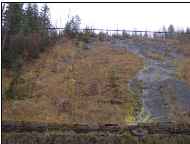
Figure 71. Photo shows the two areas of chronic wasting that need to be drained and rock blanketed.
