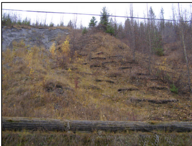
Figure 73. Photo shows drainage berm at the bottom and stabilized brush layer area.
