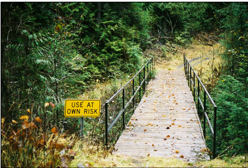
Figure 97. View eastward across Fifteen Mile Creek ATV bridge.
