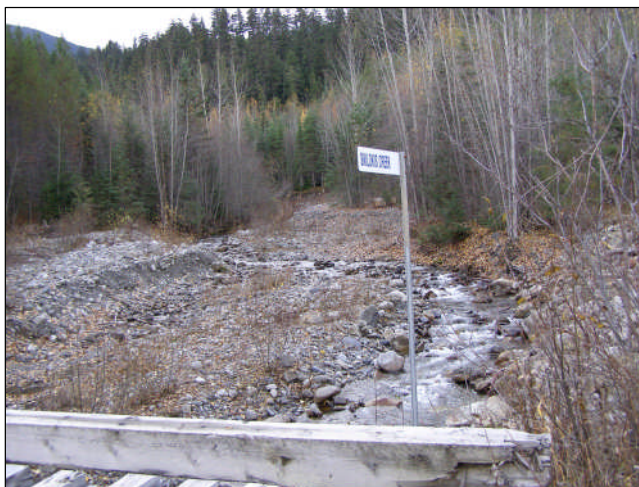
Figure 80. View upstream from bridge.
