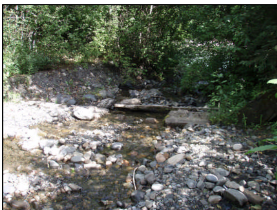
Figure 33. View downstream to 2 nd lock block set.
