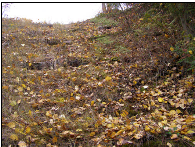
Figure 104. View of the upper, northern portion of Slide 2.
