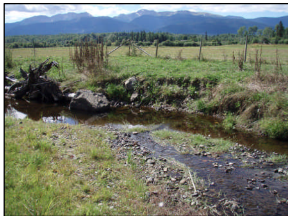
Figure 26. View of bank erosion at upper end.
