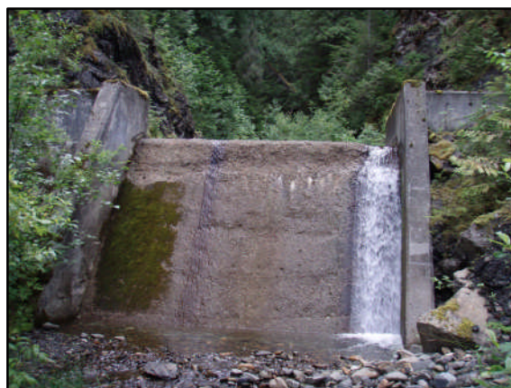
Figure 34. Dam spillway 630 m upstream.
