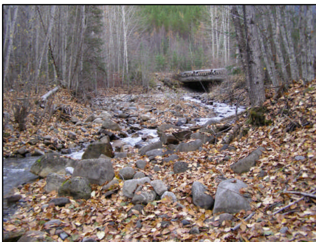
Figure 88. View upstream – 69 m to bridge.
