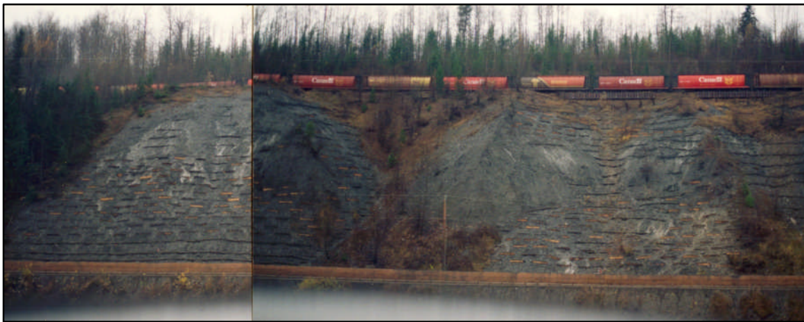
Figure 70. CN Rail tracks at the top, hillslope stabilization structures completed in 1997, and brown drainage berm at the toe of the slope.
