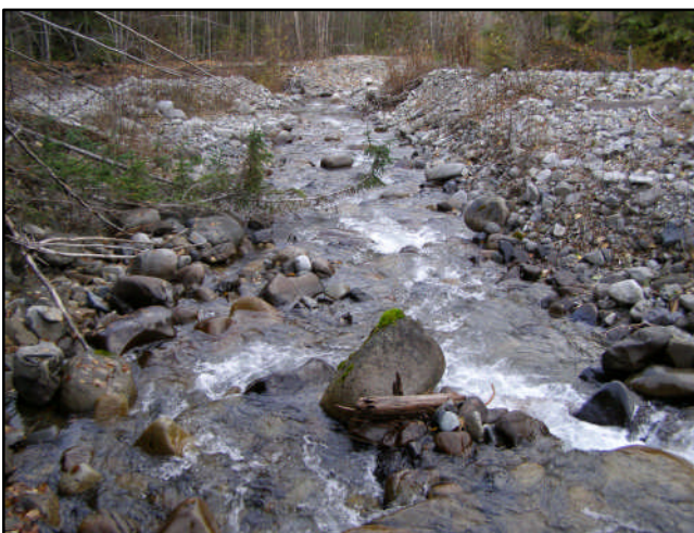
Figure 84. View downstream to bridge-130 m.
