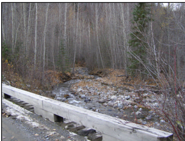
Figure 81. View downstream from bridge.
