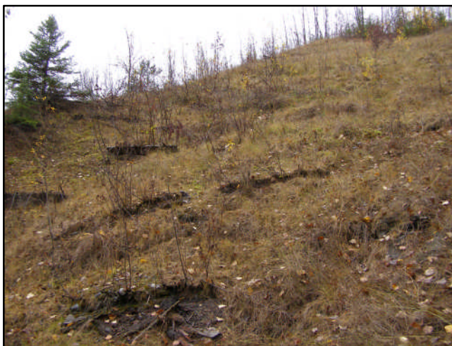
Figure 79. Photo shows modified brush layers with willows established.
