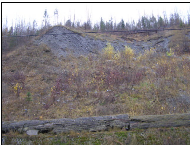
Figure 75. Photo shows drainage berm at the bottom, stabilized brush layer area, and seepage zone above.
