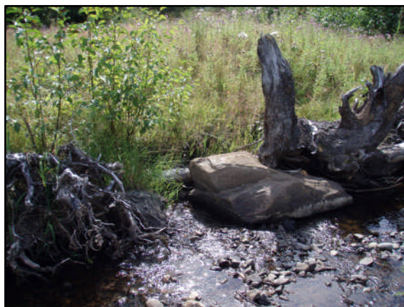
Figure 25. Boulder-rootwad placement.
