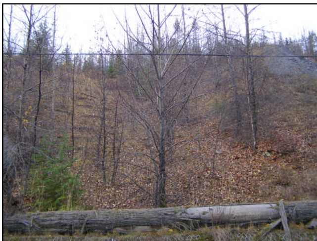
Figure 74. Photo shows stabilized Gully #1.
