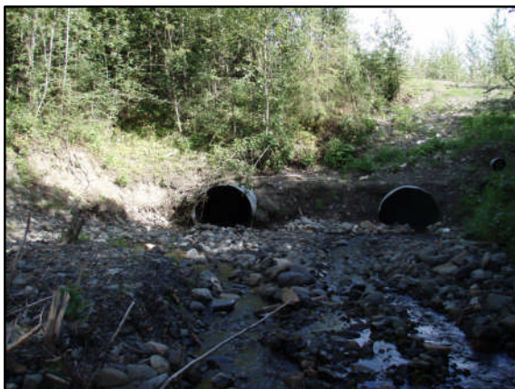
Figure 27. View downstream to culvert inlets.
