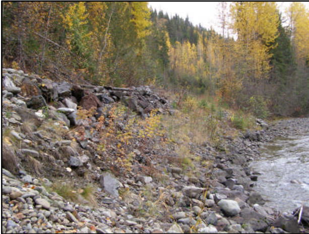
Figure 100. View upstream with Kitsequecla River on the right and berm at base of slides on the left.
