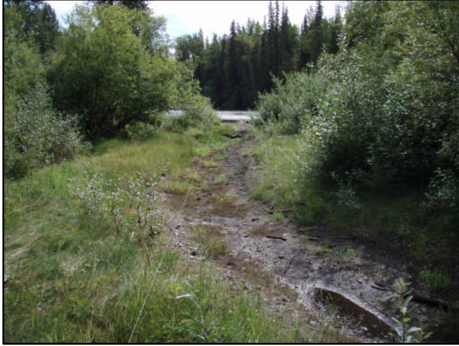
Figure 66. View shows Cullon ground channel close to Kispiox River.
