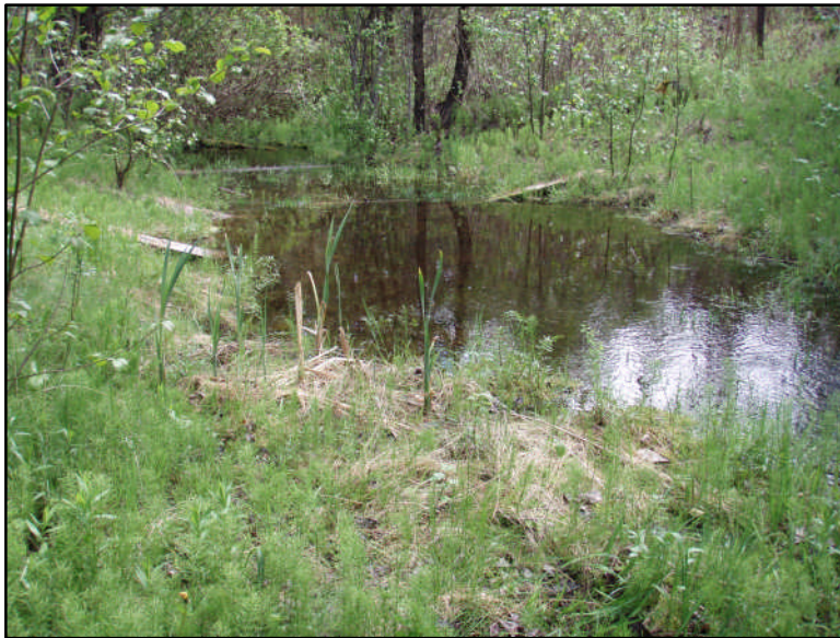
Figure 35. Deactivated wooden box culvert on Corral Creek tributary.
