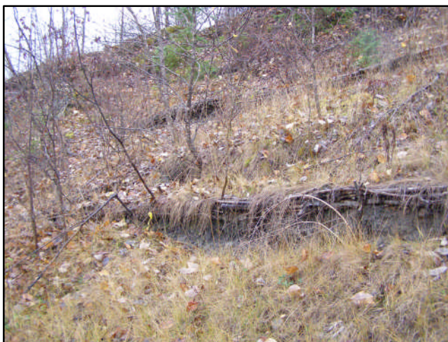
Figure 78. Photo shows functioning wattle fences in Area #4.
