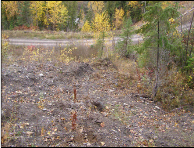
Figure 109. View down northern side of Slide 4 to the road.
