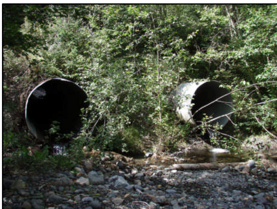
Figure 29. View upstream to culverts outlet.
