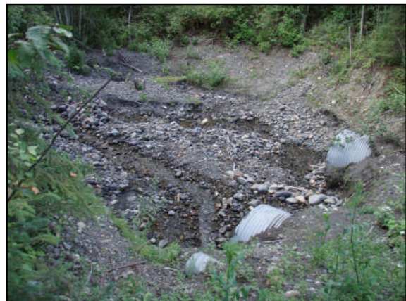
Figure 28. View upstream from culvert inlets.
