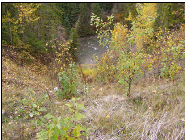
Figure 103. View down Slide 1 from the roadside.
