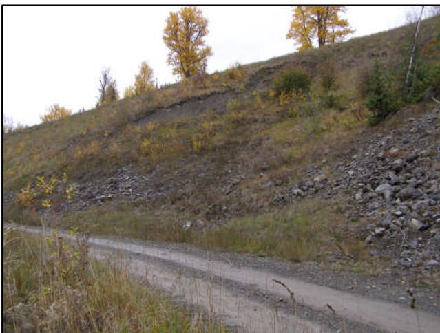
Figure 108. View up Kitseguecla FSR and the upper, northern portion of Slide 3. Note minor slumping above rock blanket.
