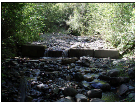
Figure 31. View upstream first lock block step.
