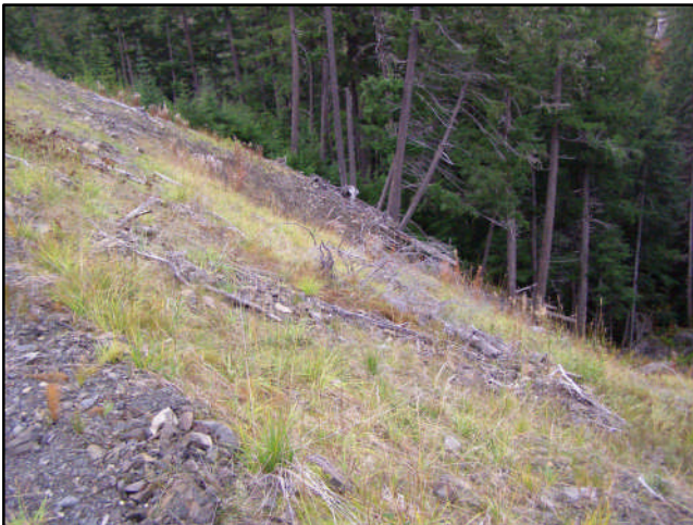
Figure 112. View across slope located at Slim Jim 0+467. The slope has been rock blanketed.
