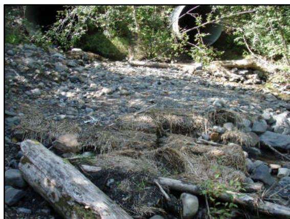
Figure 32. Remnants of hay sediment traps.
