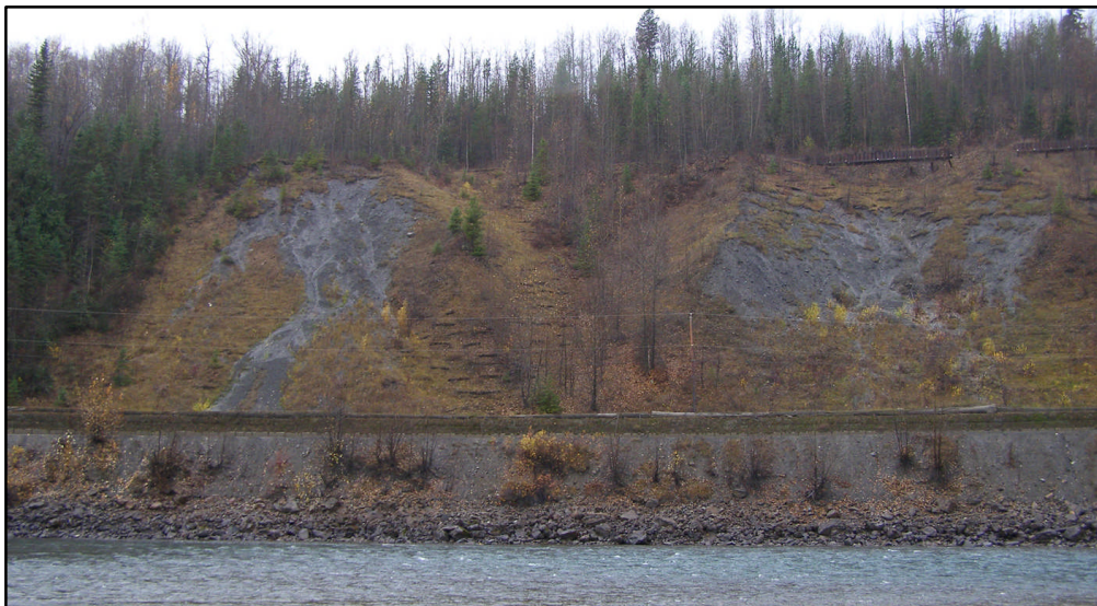
Figure 71. Photo shows the two areas of chronic wasting that need to be drained and rock blanketed.
