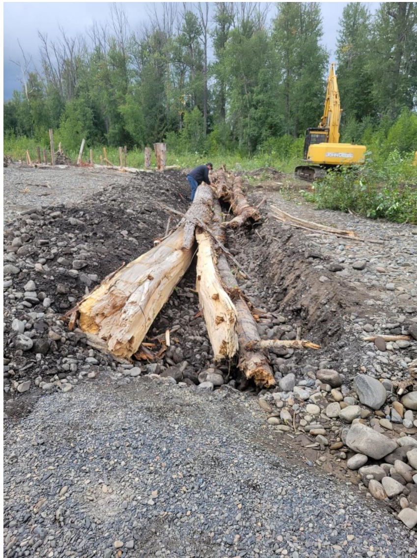
Figure 4. Bank structure put in place to prevent flood waters from channelizing towards MC1. The structure was created by roping 5 cottonwoods together and burying them with rock and gravel approximately 3-4 ft down into the streambed.
