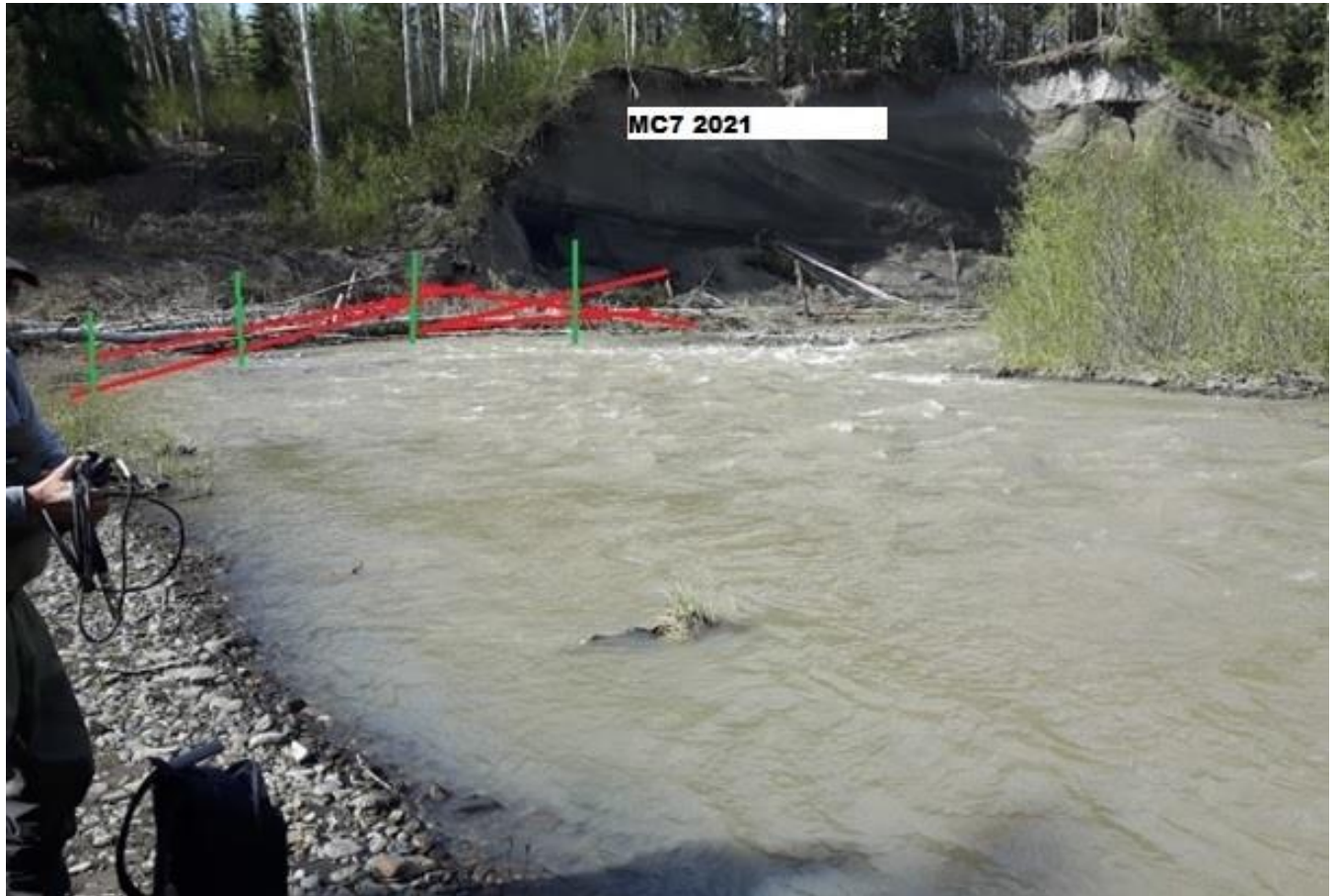
Figure 8. This image was taken at MC7 in 2021, where bank stabilization structures were placed in 2018-2019. The structures have subsided slightly and this site needs to be refurbished as of 2023. The red and green lines represent how the original structure looked when it was first built in 2018-2019. The green lines represent upright logs and the red lines represent horizontal logs.
