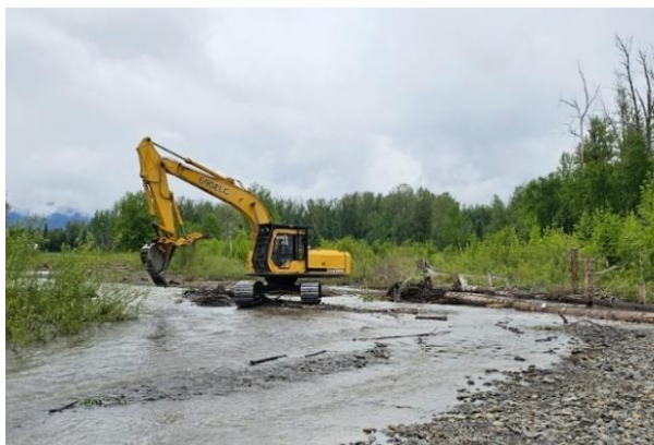
Figure 2. Emergency creek diversion to prevent the main stem of the creek from flowing directly into MC1. June 5, 2023.
