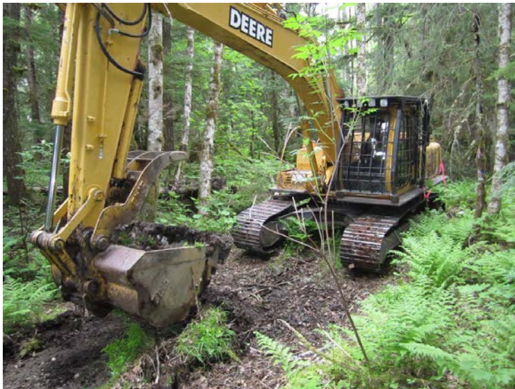
Photo 1. The Beginning of Channel Excavation.
