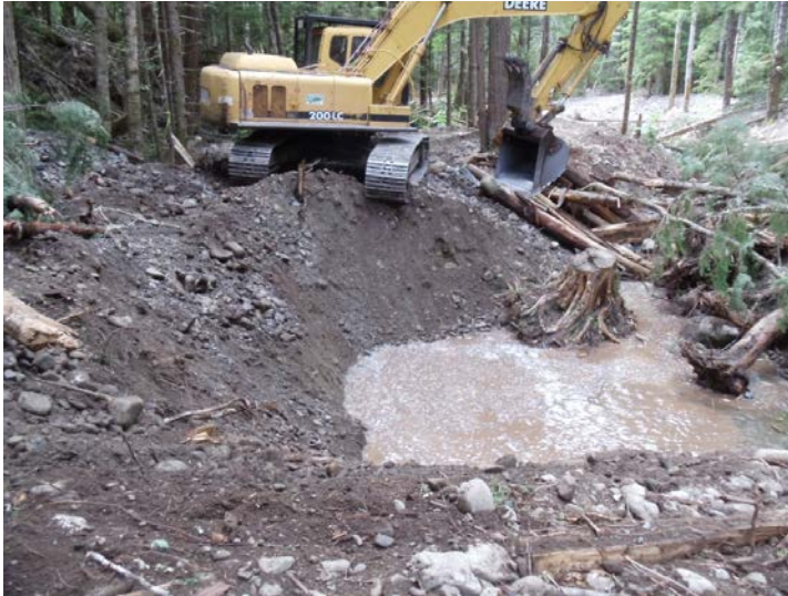
Photo 5. Construction of Undercut Bank @ 0+305m.
