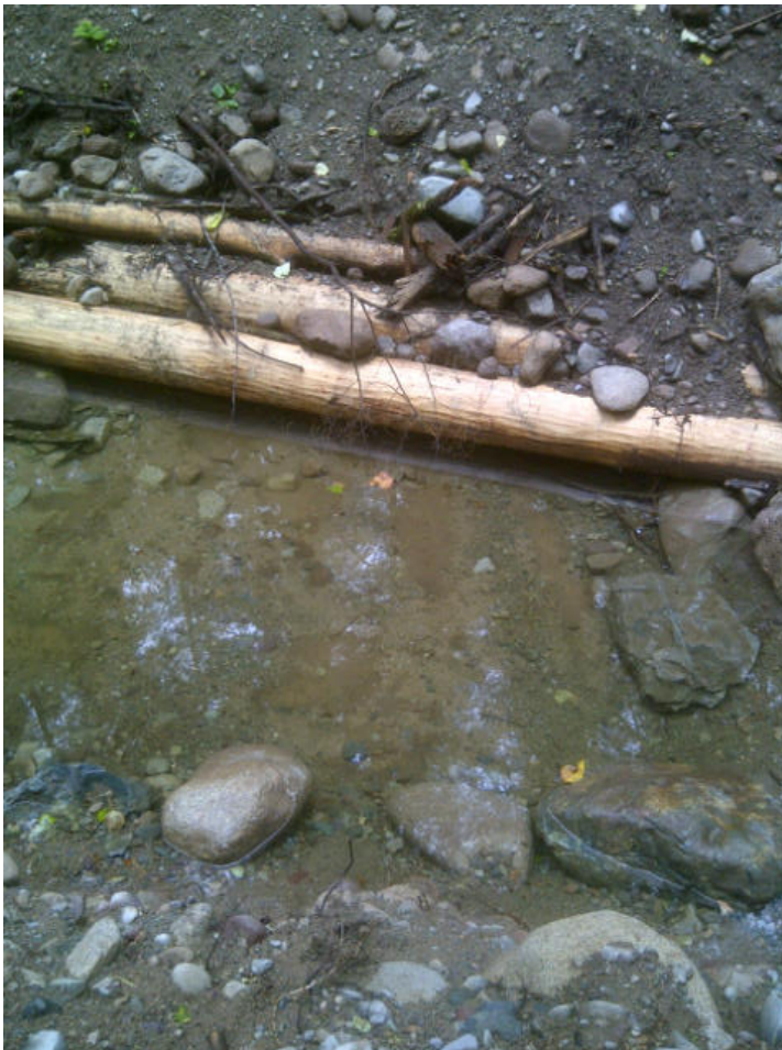
Photo 6. Completed undercut bank
