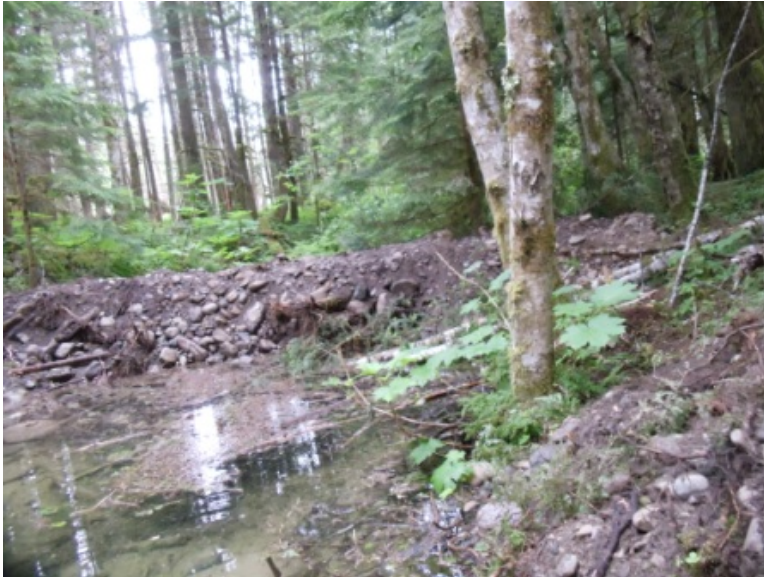
Photo 2. Re-constructed Earthen dam @ 0+0m.
