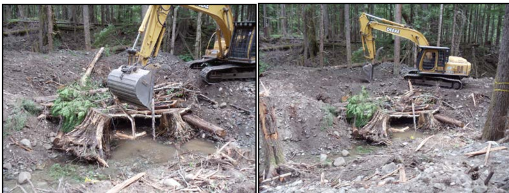
Construction of Undercut Bank @ 0+305m.
