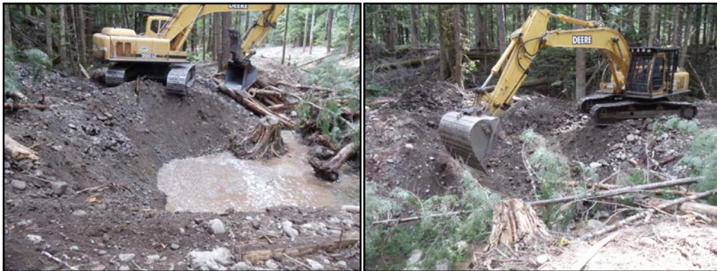
Construction of Undercut Bank @ 0+305m.
