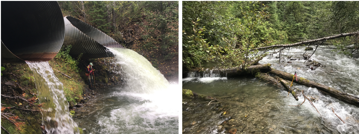
Figure 5.13: Left: Outlets of PSCIS crossing 124487. Right: Typical habitat downstream of crossing 124487 below the railway bridge and adjacent to the Bulkley River mainstem.
