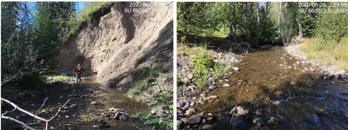
Figure 5.38: Left: Habitat upstream of PSCIS crossing 197664 and location of cutslope. Right: Habitat upstream of PSCIS crossing 197664.
