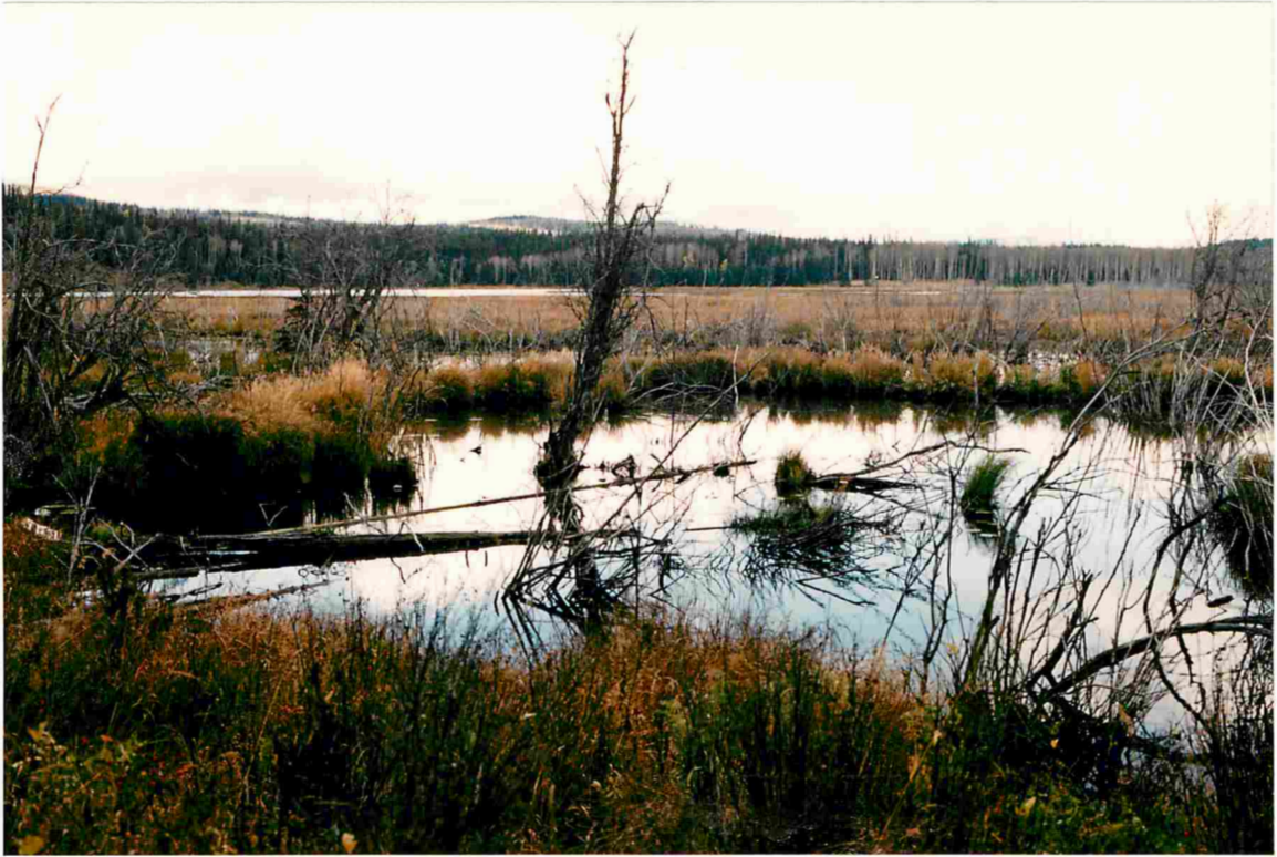
Figure 6. Looking downstream at dam that blocks the inlet stream from McBrierie Lake.
