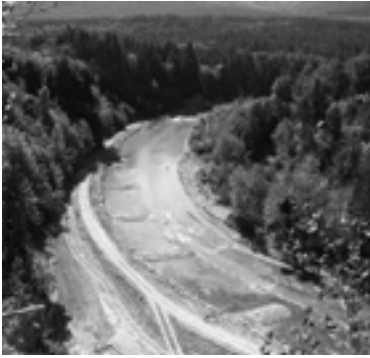
Channel realignment and bank armouring at Stoltz Bluff in the Cowichan River.
