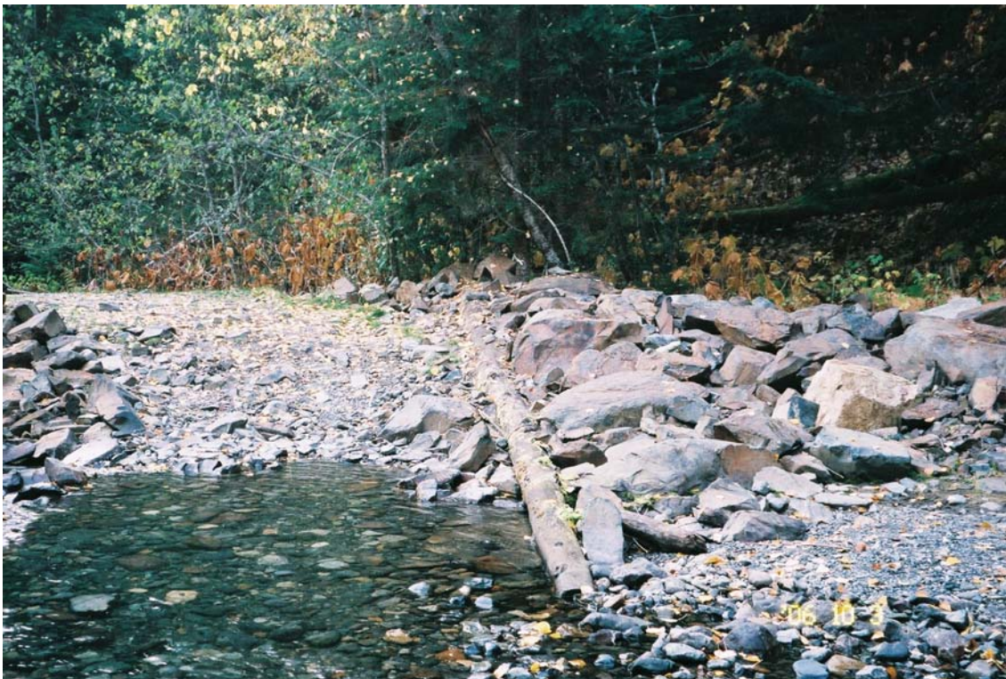
Toboggan Creek Site. Empty side ford approach at Toboggan Creek crossing with log deflector in place.
