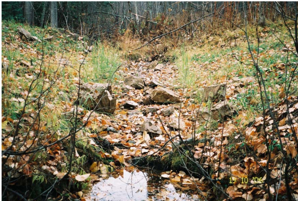
Site 3006-2. Upstream view of completed channel.
