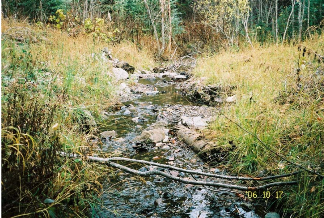
Site 413-123. Downstream view of reconstructed channel.
