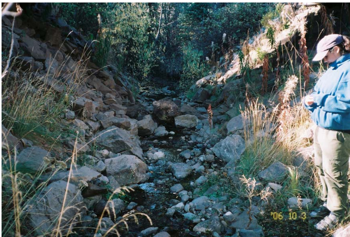
Site 19.3km Telkwa. Downstream view of reconstructed channel under bridge installed in 1999.
