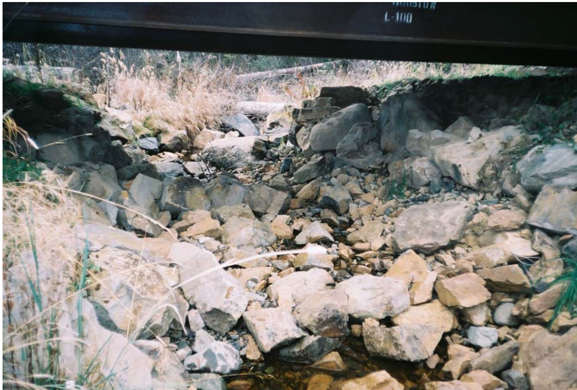
Site 487-34. Upstream view of reconstructed stream channel under new bridge.
