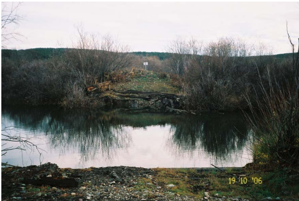
Site 306A. View across Fulton River with bridge removed.
