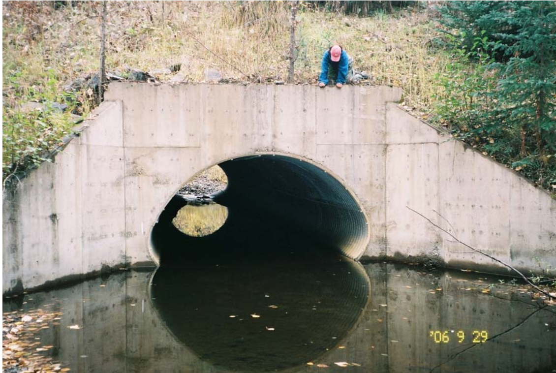
Site 4000-Feature 23/696. Heal Creek. Culvert outlet; apron and culvert backwatered.
