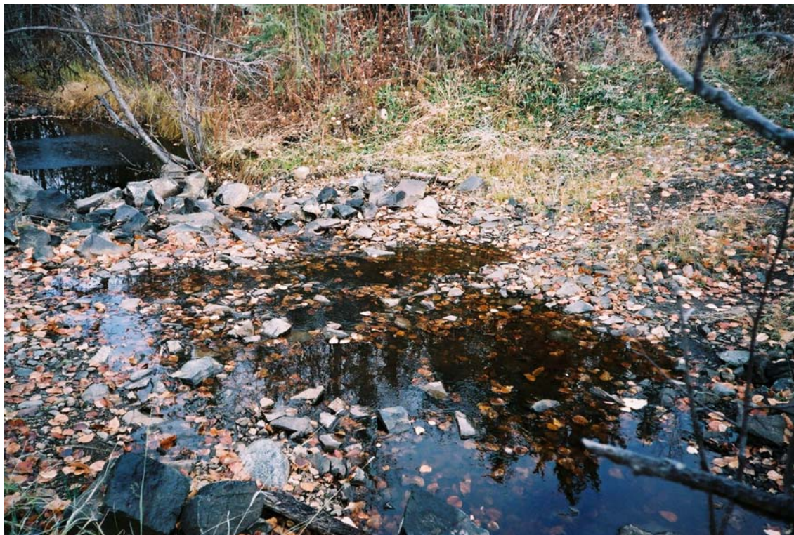
Site 473-1. View across ford from loaded side. No erosion or scour evident.
