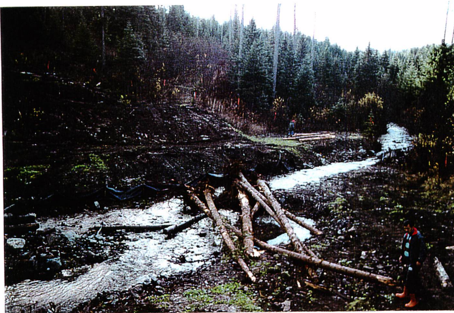
Photo 3 looking upstream after pullback of the collapsed bridge. The foreground shows a thalweg formed around a collapsed bridge structure removed during 1997. The sediment wedge in the upper right of the photo was deposited above the bridge in a 1 in 100 year event and is considered stable.
