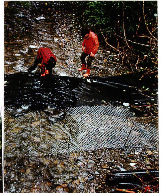
Photo 2 installing silt fence.
