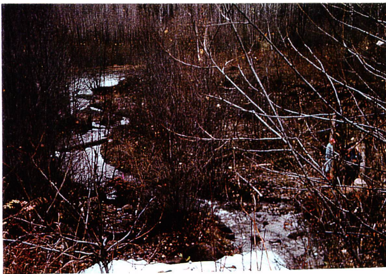
Site 15/Photo 2. Installed works from photo station 1. Workers are tying down the stems placed to control high water erosive forces. The log in the center of the photo is the log in Photo 3. Above
