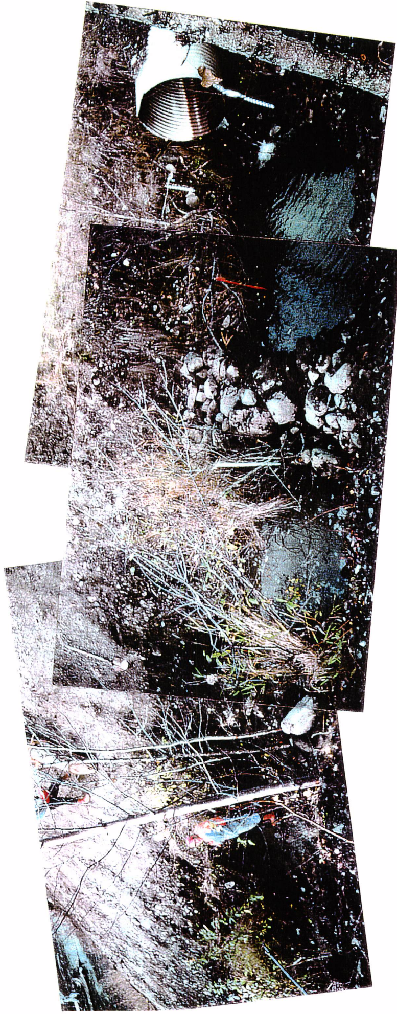
Photo caption of Site 14 shows the two jump pools constructed and the LWD being installed by hand below the pools. The pullback above the site was completed to open the area to light without removing the riparian vegetation or the stream bed. The area was seeded and a silt fence installed.
