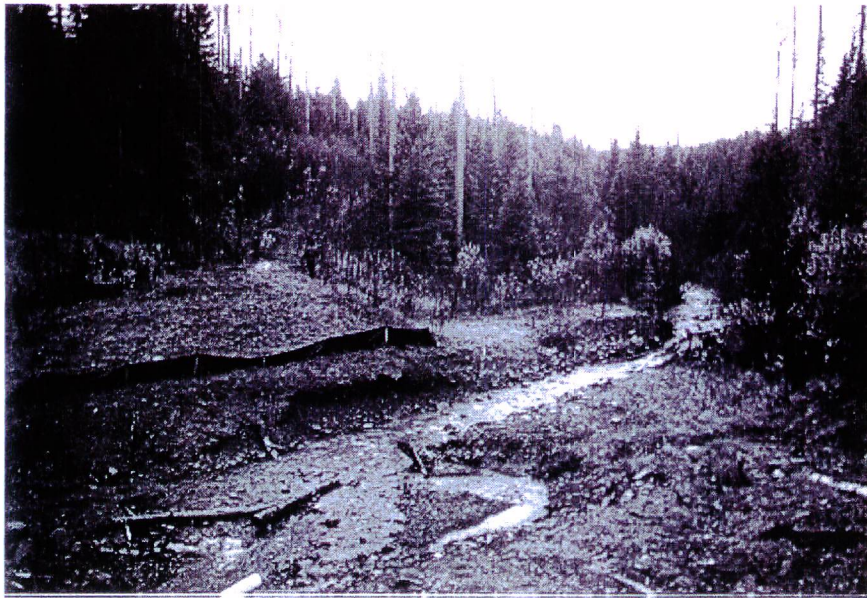
Photo 1. Looking upstream from the former road crossing on Site 3. Note that the road material on the far side was eroding despite earlier pull back of the slope.
