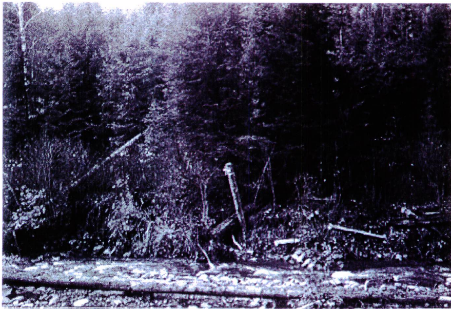
Photo 4. Looking southeast from Photo Point 1. Note the post placed in the bank to stabilize the LWD with root wad.
