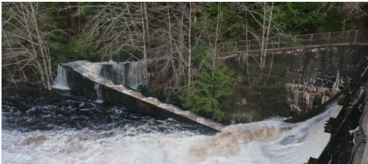
Figure 8. Kloiya fishway during a period of high flow showing cracks in concrete structure.
