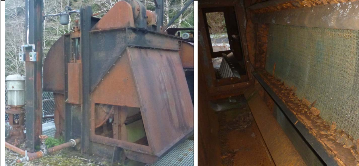
Figure 9. Outside and inside views of the travelling rotating intake screen for the 70" stave pipe at the Kloiya River dam.
