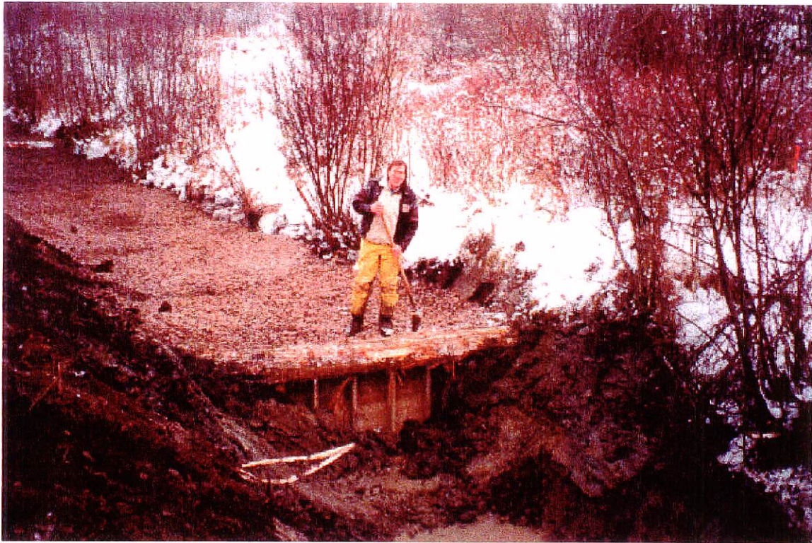
Figure #8 – Site 3B – Abutment placement in spawning channel
