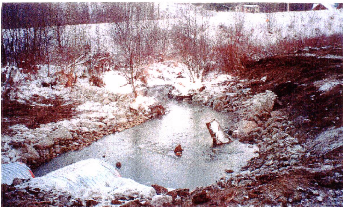
Figure #2 – Upstream view of Site 2 – Installation of culverts & pool development
