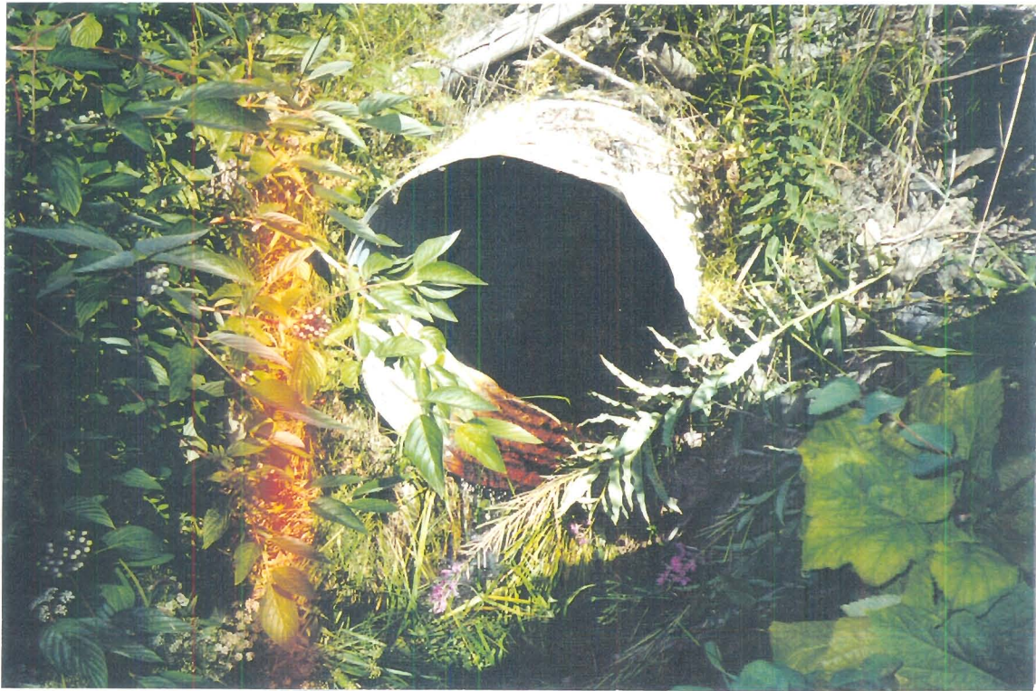
Site #647, Upstream photo of a 900 mm culvert Roll #15, Frame #1, Date: 2000/08/07
