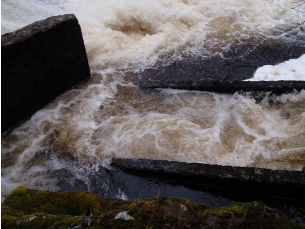
Picture 2. Entrance to Kloiya River fishway.
