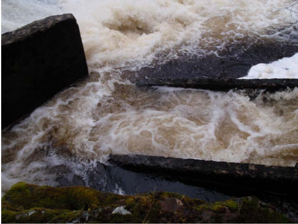
Picture 2. Entrance to Kloiya River fishway.
