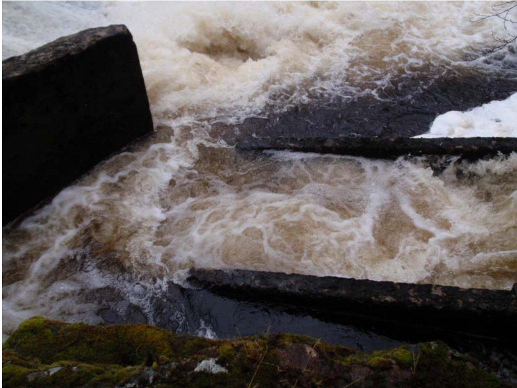
Picture 2. Entrance to Kloiya River fishway.
