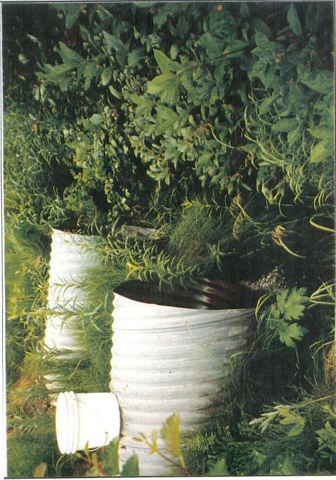
Photo 25. Owen C. Tributary OW3, R1, Site 8 - Road Culverts
