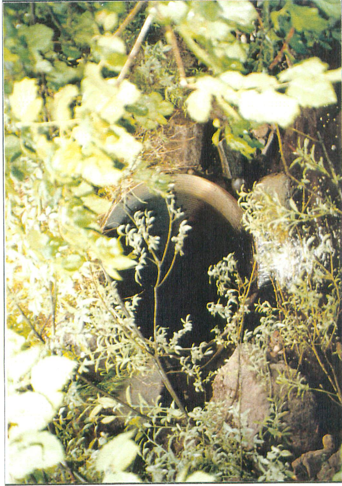
Photo 9. Owen C. Tributary OW2, R1, Site 2 - Upstream at Culvert
