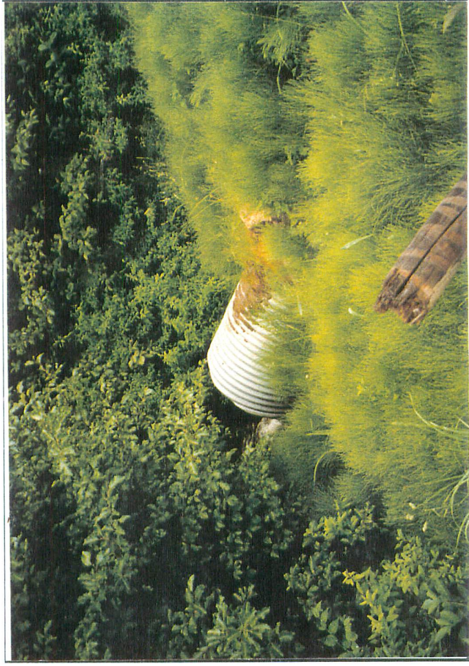
Photo 92. Owen C. Tributary OW14, R1, Site 38 - Road Culvert
