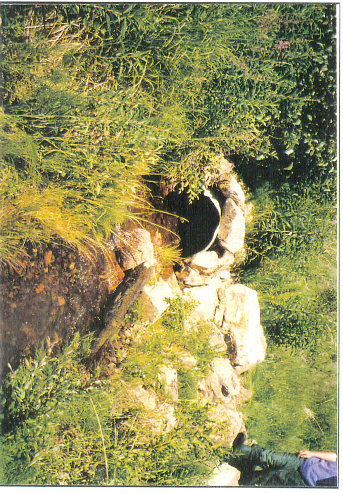
Photo 64. Puport C. Tributary PU1, R1, Site 25 - Road Culvert
