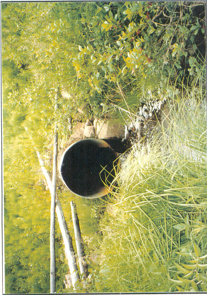
Photo 57. Puport C. Tributary PU1, R2, Site 22 - Road Culvert
