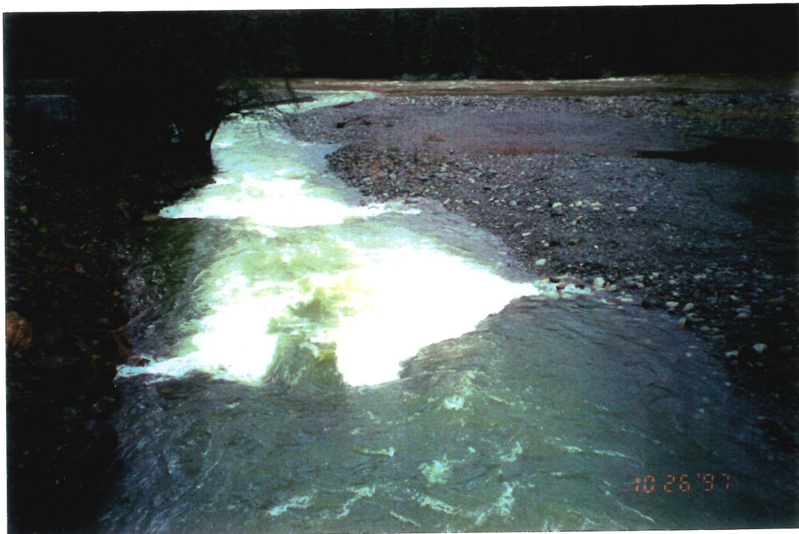
Photo 2. Downstream Simpson Creek after rock vee installation (10-26-97)
