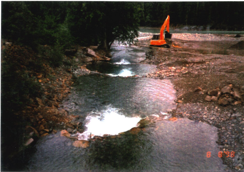
Photo 3. Excavation of lower rock vee (8-8-98).
