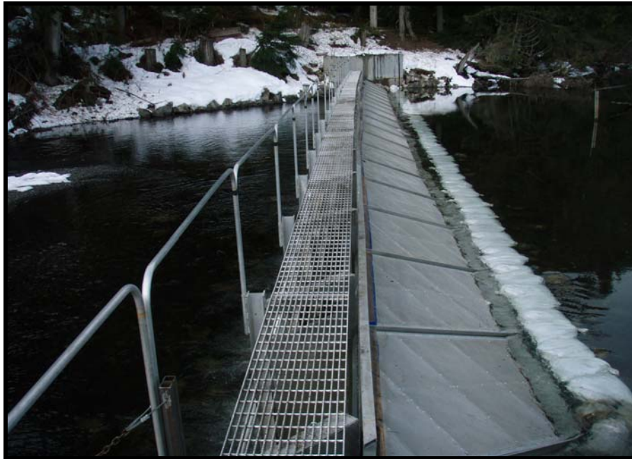
Figure 8: Completed weir installation with new non-skid walkway and safety railings.
