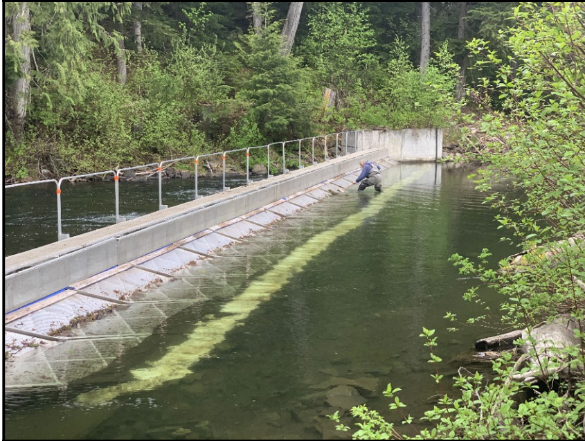
Figure 6: Photo showing GFA technician cleaning debris off panels
