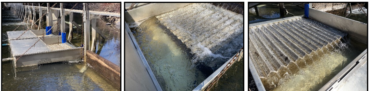
Figure 7: Photo series showing v-trough and stop-logs (left), high flow situation (middle) which needed adjustment and photo on right showing adjusted v-trough
