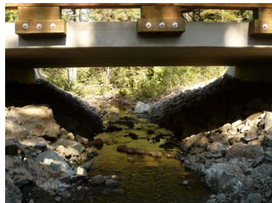
Photo 3. View of new bridge across restored stream channel.
