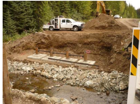
Photo 2. View of bridge footing beyond newly restored stream channel
