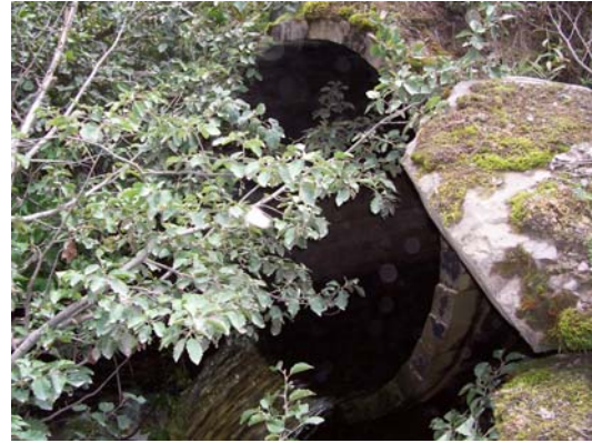
Photo 1. Original stream culvert.
