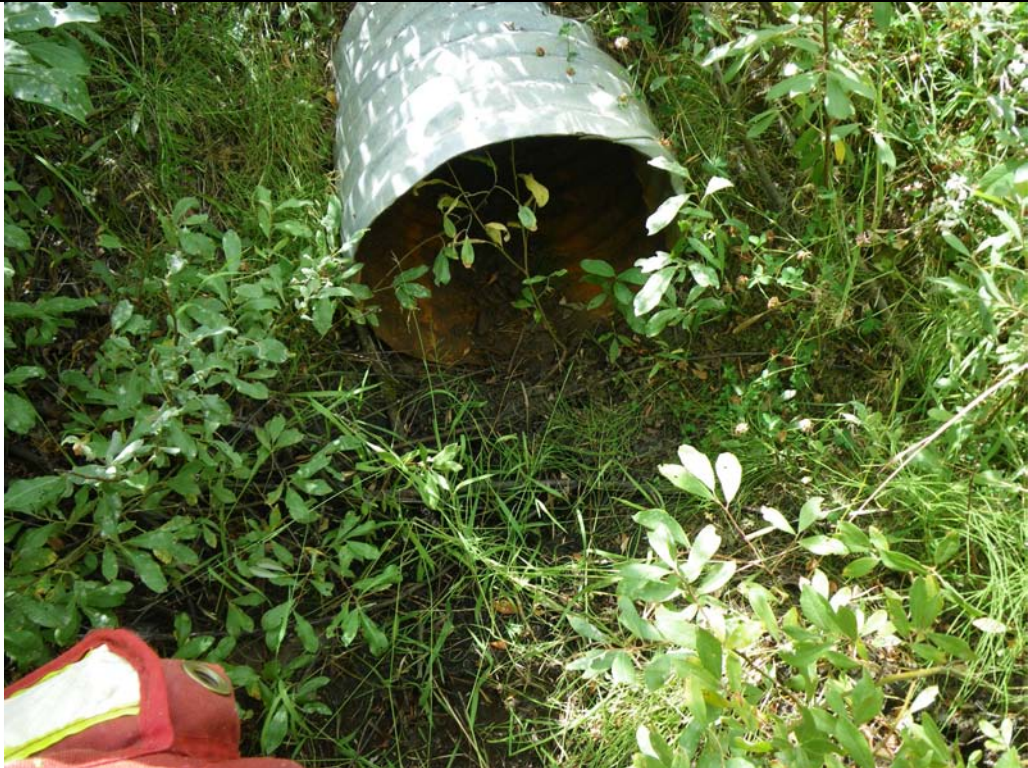
Stream/ILP: 9002 Image: 383 Comment: Downstream, Culvert inlet. 8/20/2010.
