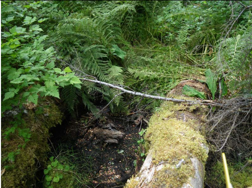
Stream/ILP: 9004 Image: 389 Comment: Downstream, Down Ditch. 8/20/2010.
