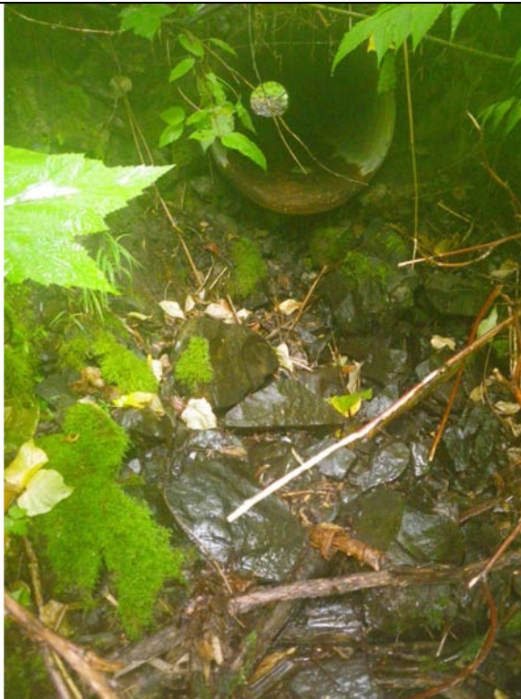
Stream/ILP: 7017 Image: 0358 Comment: Upstream, Culvert. 8/23/2010.
