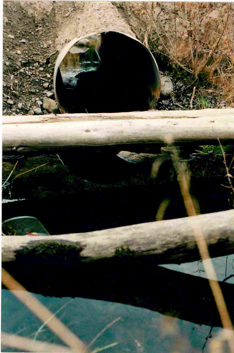
Figure 12. Culvert under the logging road at the Day Lake outlet stream.
