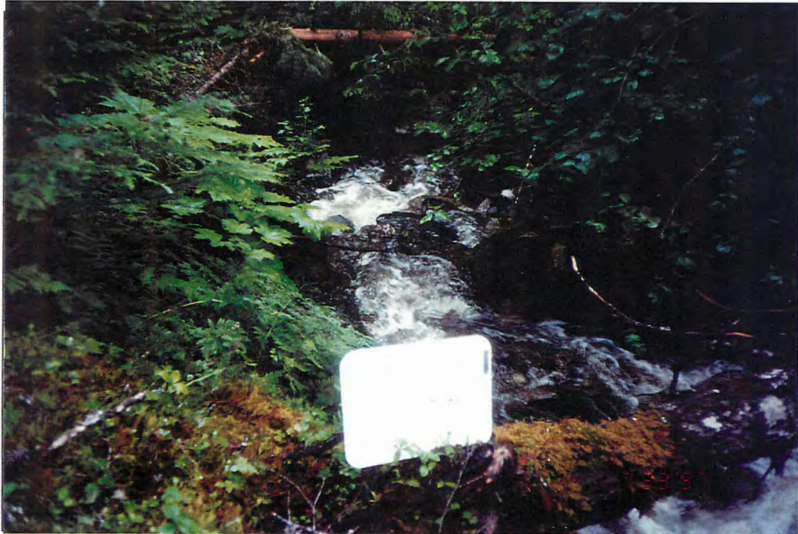
Photo #: W-11-16, 23-Jul-97 Site #: W100, Looking downstream at the channel
