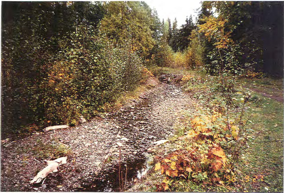
Photo #: A-5-23, 27-Sep-96 Site #: A53, Looking upstream, channel beside road.
