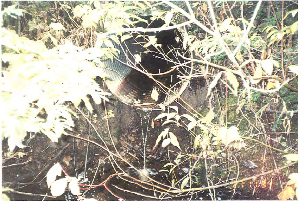
Photo #: R-8-17, 1996/09/27 Site #: R132, Looking upstream toward culvert.
