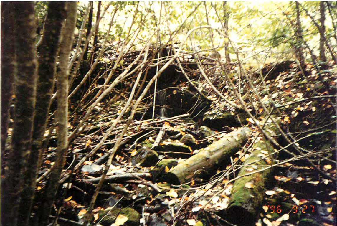
Photo #: A-5-12, 27-Sep-96 Site #: A48, Looking upstream toward culvert, old logging debris.
