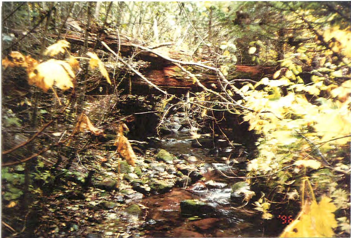
Photo #: A-5-13, 27-Sep-96 Site #: A49, Looking upstream.
