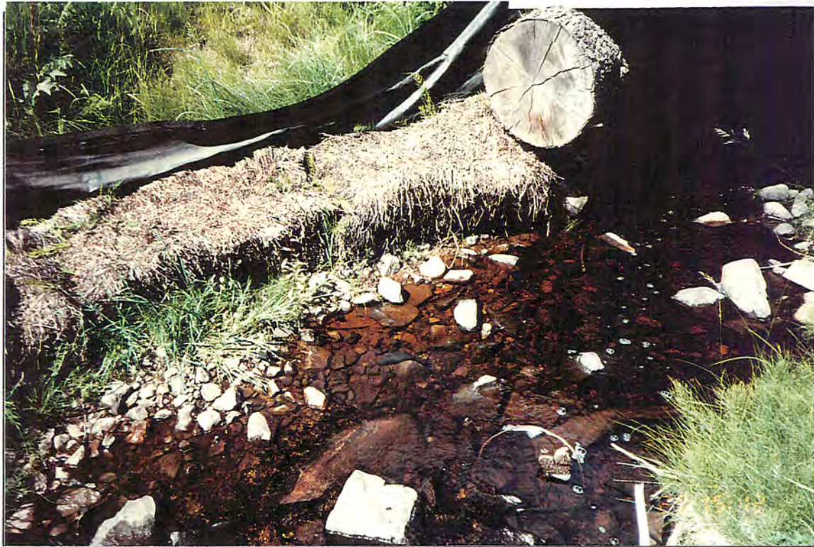
Photo #: T-2-11, 1996/07/29 Site #: T31, Upstream view, stabilization.
