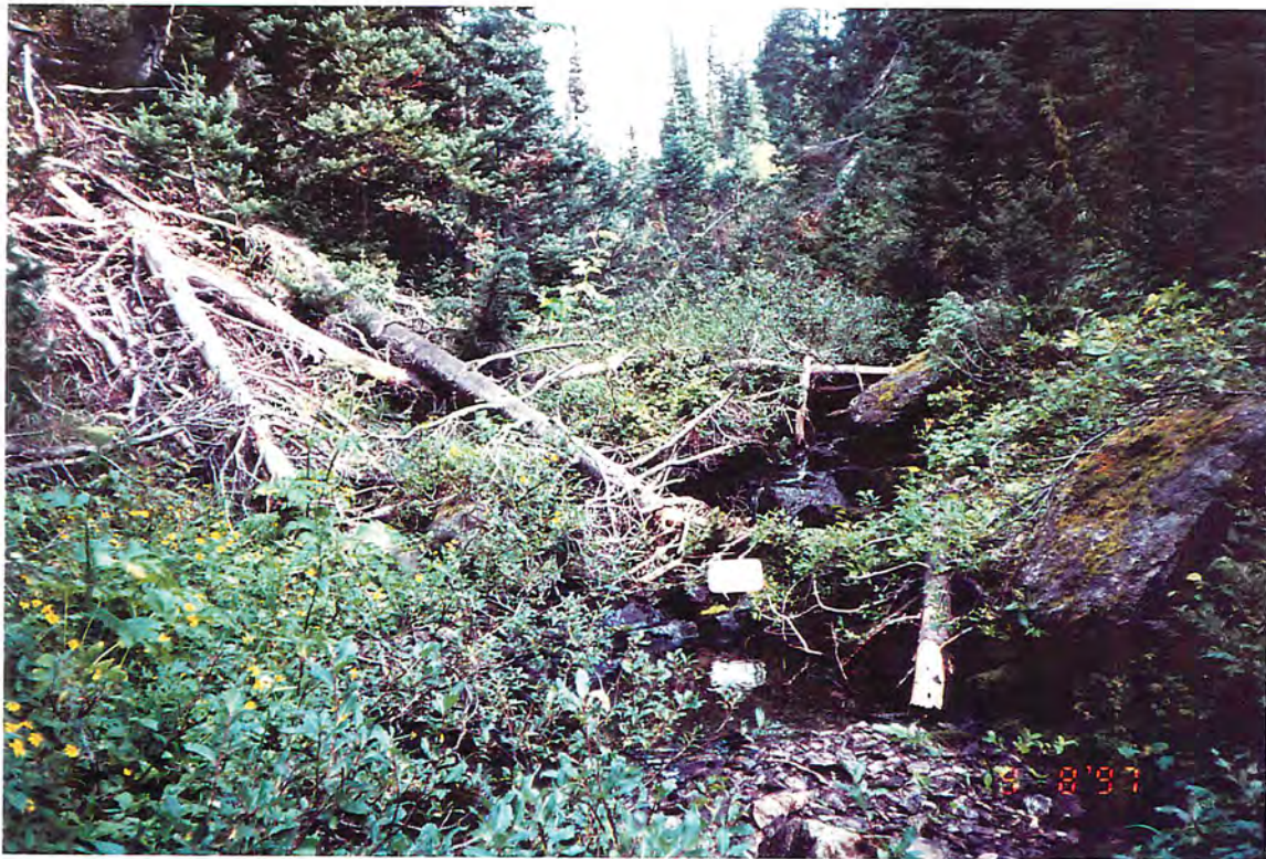
Photo #: Y-27-23, 08/09/97 Site #: Y229, Looking upstream at the channel
