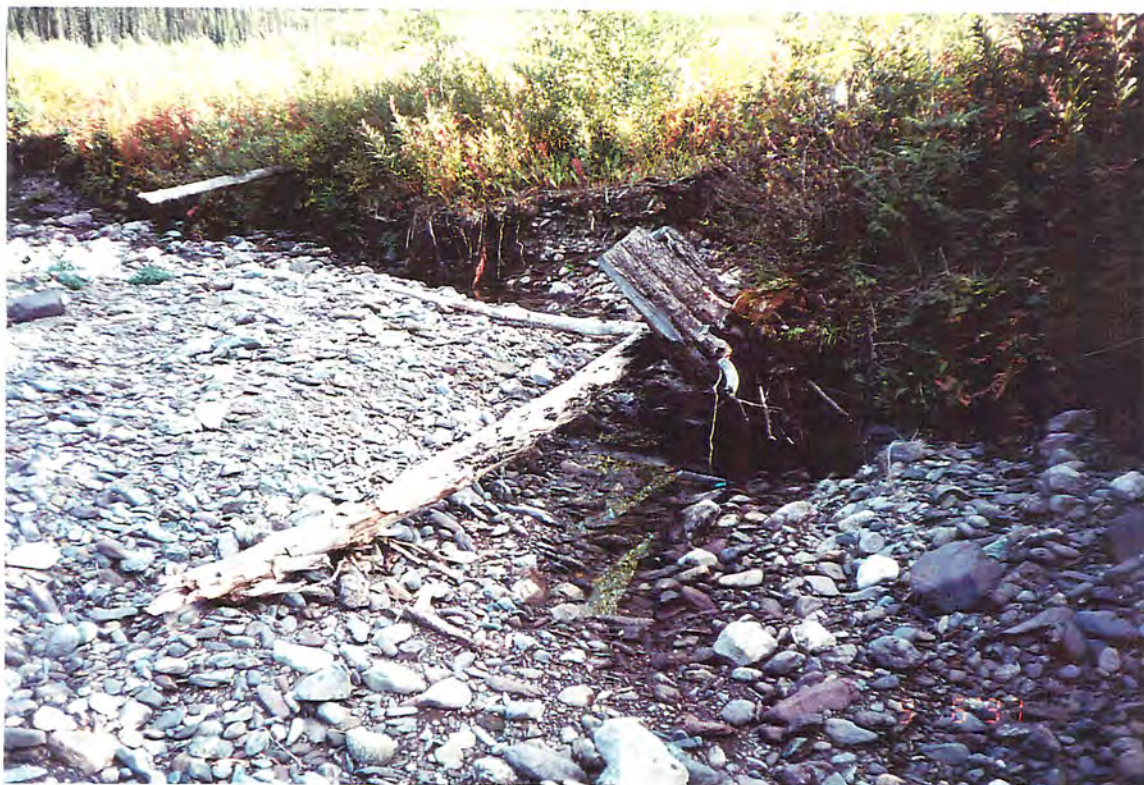
Photo #: Y-26-13, 06/09/97 Site #: Y221, Looking upstream at the channel
