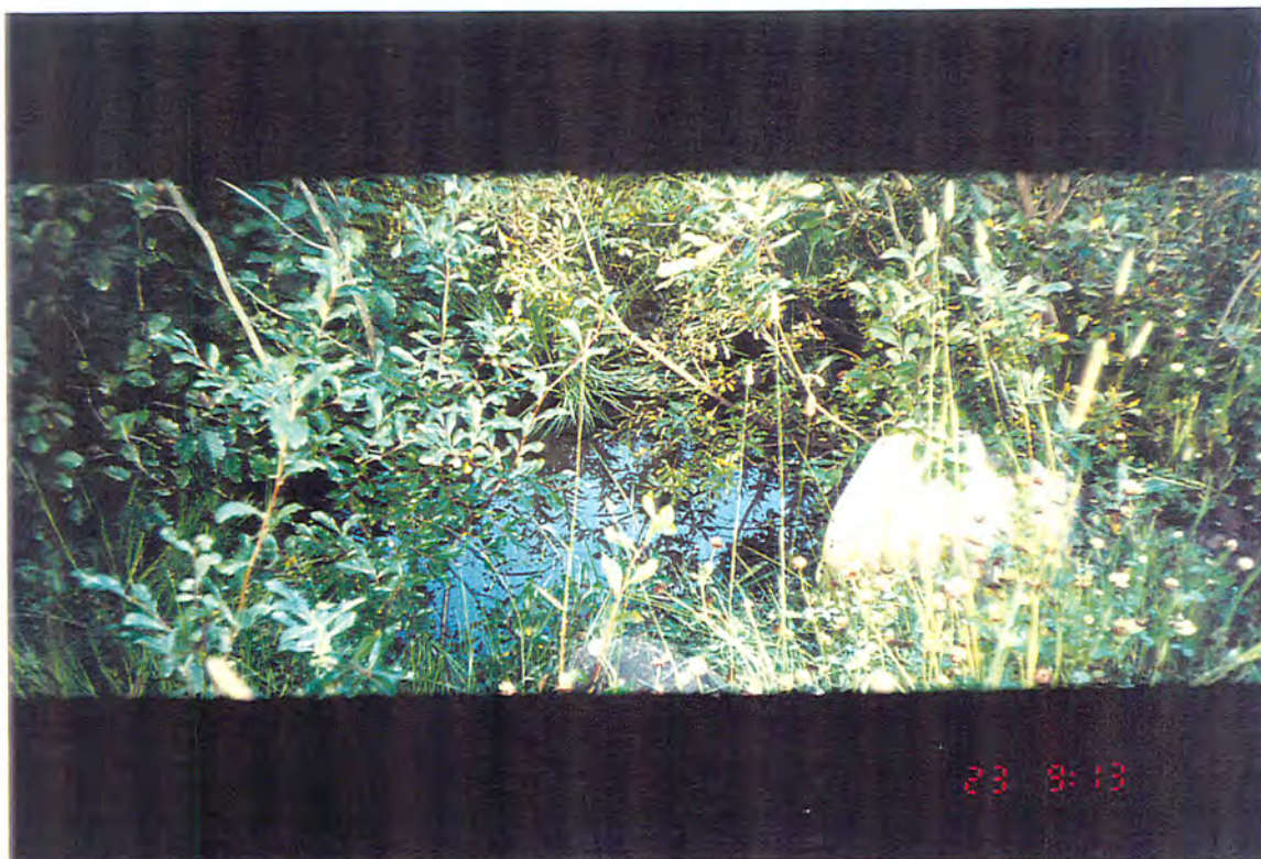
Photo #: T-8b-14, 1996/08/23 Site #: T150, Not a creek, culvert at road.
