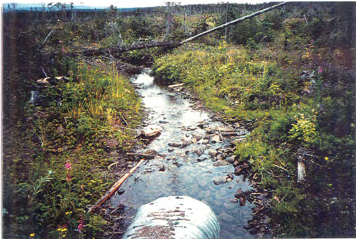
Photo #: J-6-16, 1996/08/18 Site #: J107, Looking downstream from culvert.
