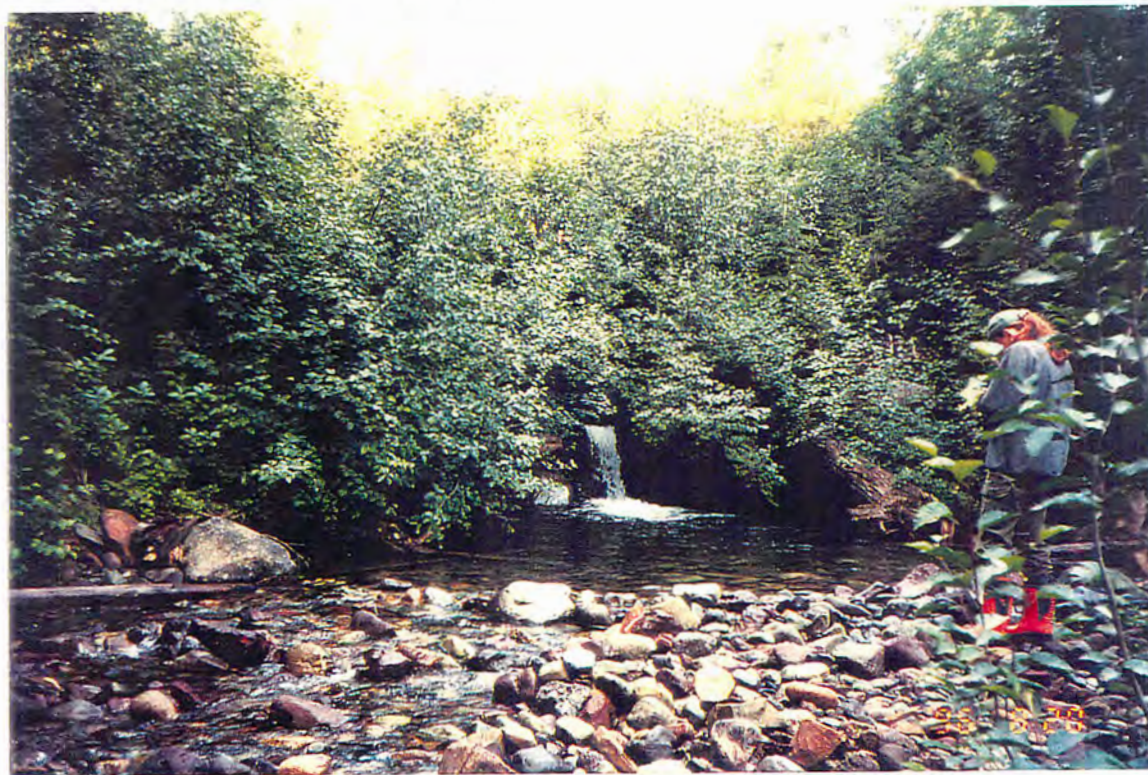
Photo #: H-6-14b, 1996/08/20 Site #: H97, Looking upstream toward culvert.
