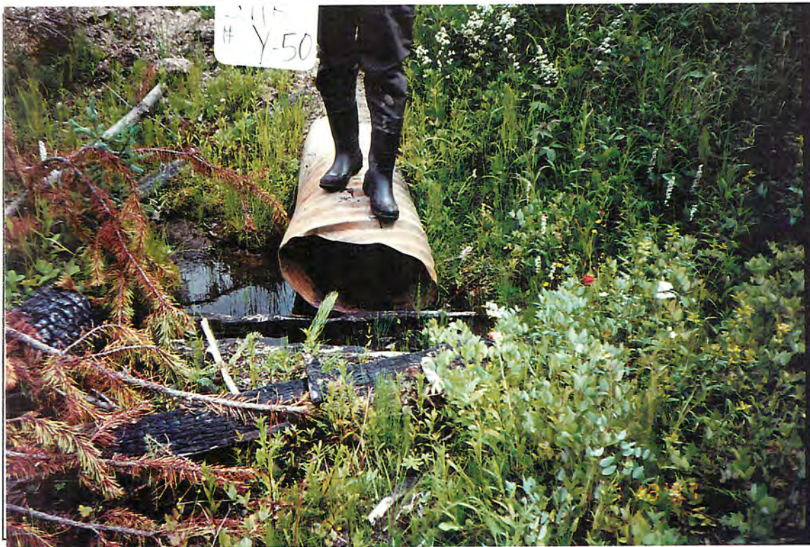
Photo #: Y-7-9, 18/07/97 Site #: Y50, Looking downslope at the channel, note the condition of the culvert.
