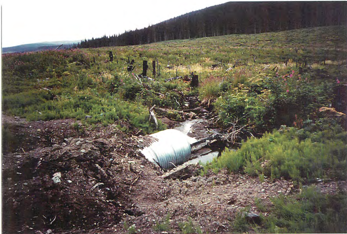
Photo #: J-6-17, 1996/08/18 Site #: J108, Looking upstream past culvert.
