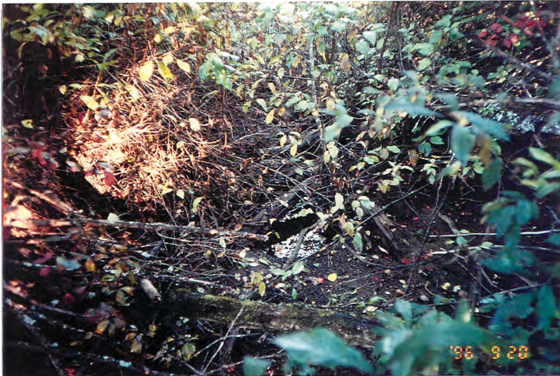
Photo #: A-1-14, 19-Sep-96 Site #: A6, Looking upstream.
