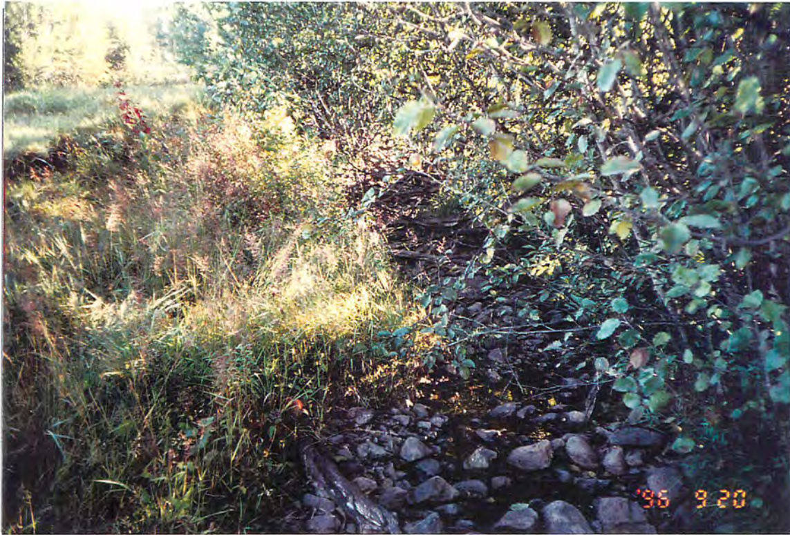
Photo #: A-1-7, 19-Sep-96 Site #: A3, Looking upstream.
