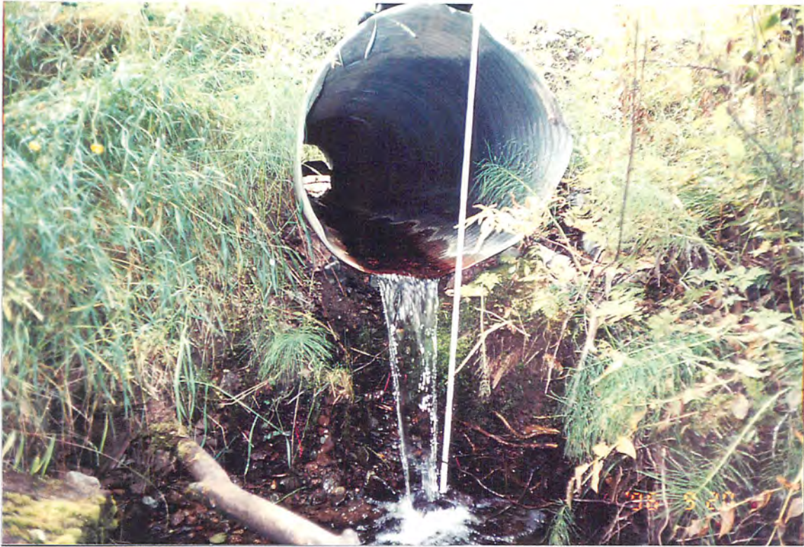
Photo #: R-5-7, 1996/09/20 Site #: R78, Looking upstream toward culvert.
