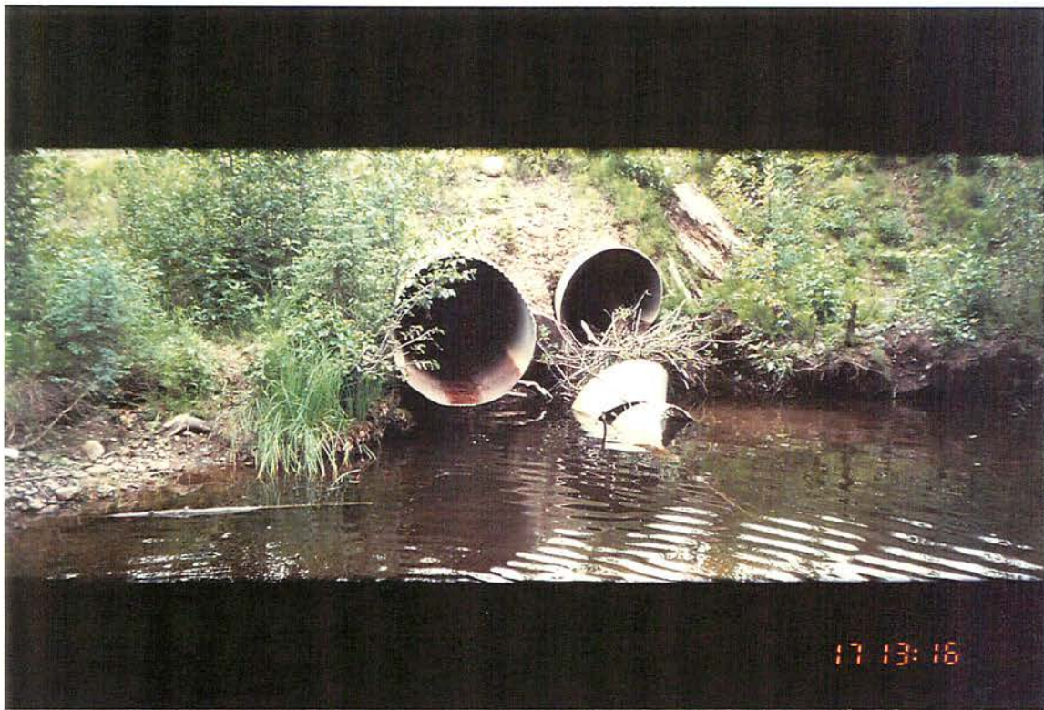
Photo #: T-6-17, 1996/08/17 Site #: T114, Upstream view, two culverts.
