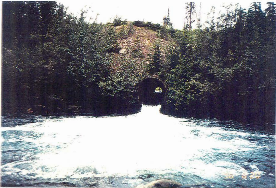
Photo #: H-6-21, 1996/08/20 Site #: H99, Looking upstream toward culvert.
