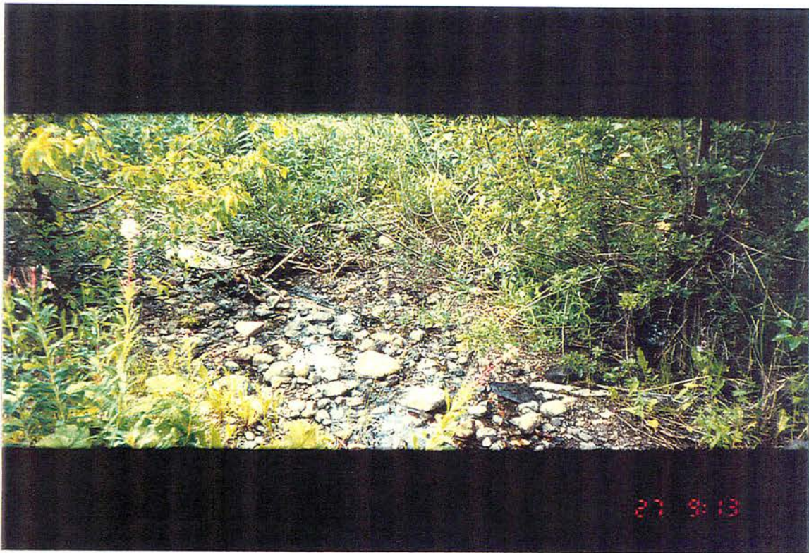
Photo #: T-10-20, 1996/08/27 Site #: T179, Downstream view taken from road.
