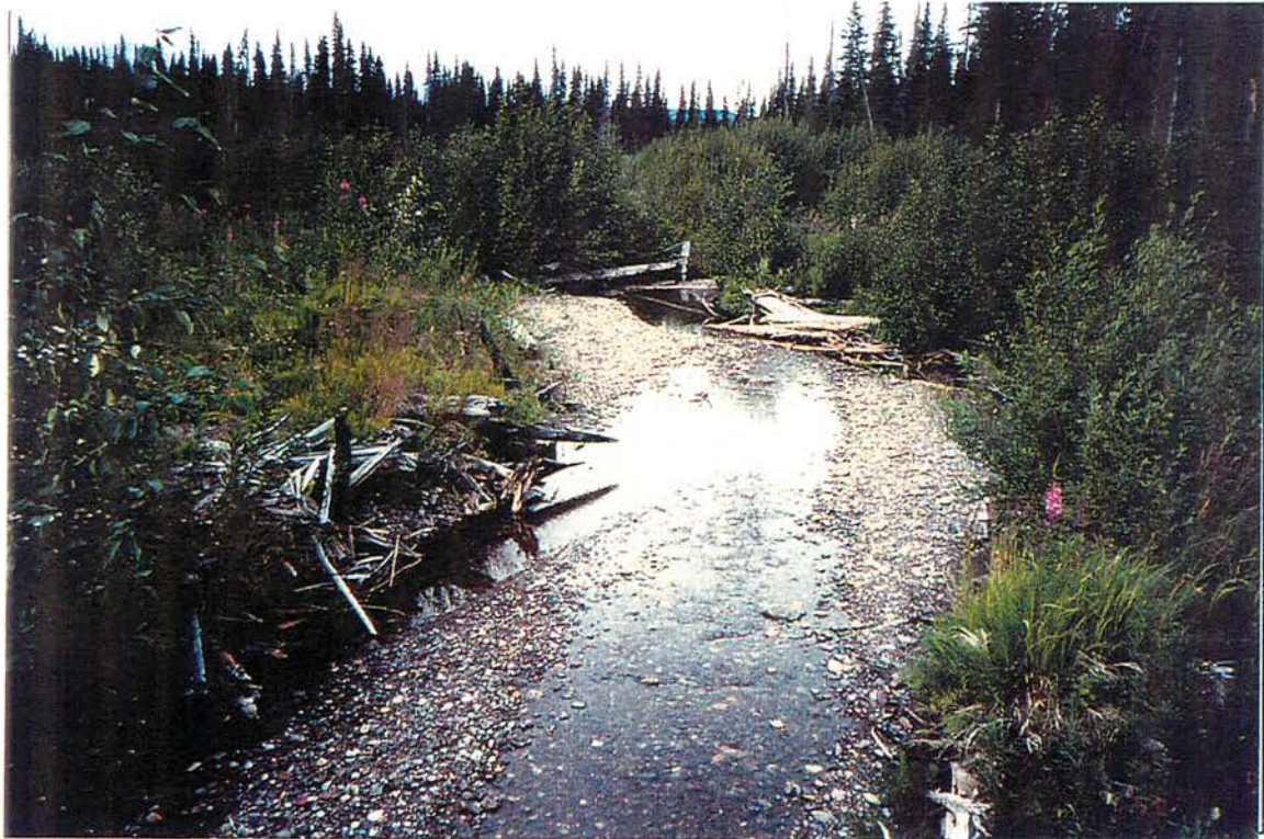
Photo #: J-6-7, 1996/08/16 Site #: J103, Looking downstream from bridge.
