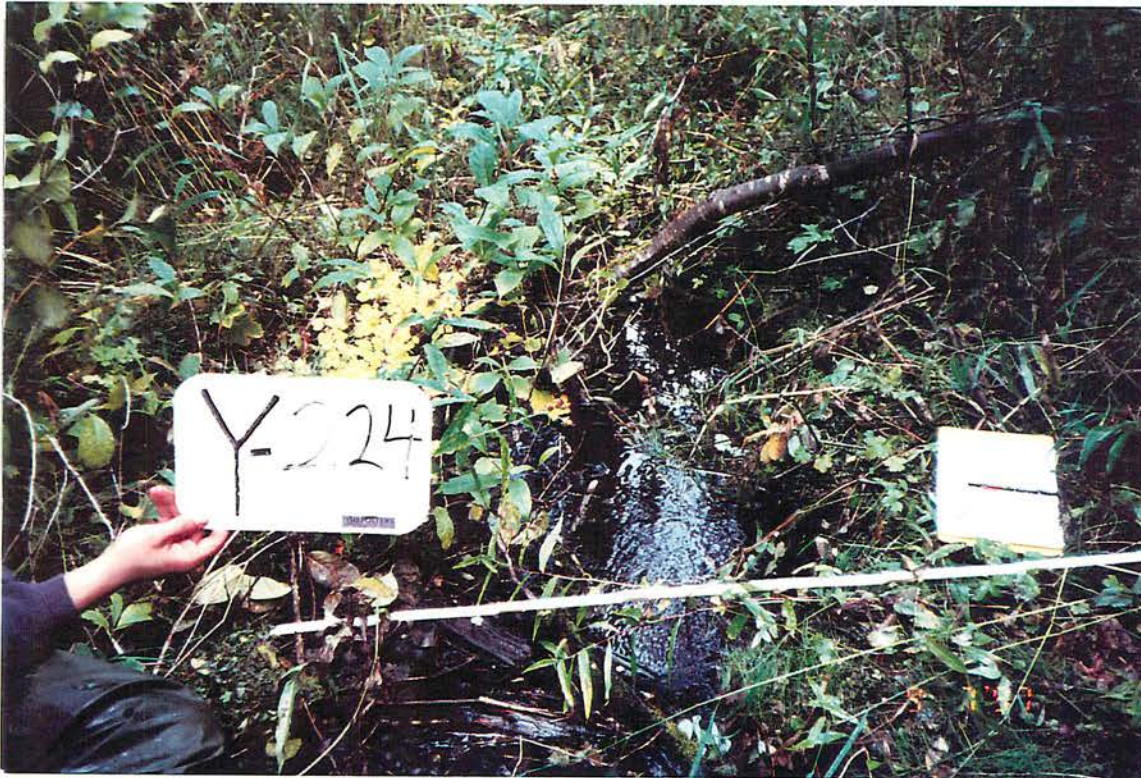
Photo #: Y-27-4, 07/09/97 Site #: Y224, Looking downstream at the channel
