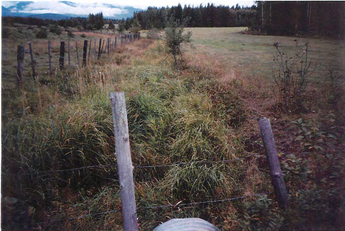
Photo #: W-N-1, 05-Sep-97 Site #: W232, Looking upstream at the channel, overgrown with grasses
