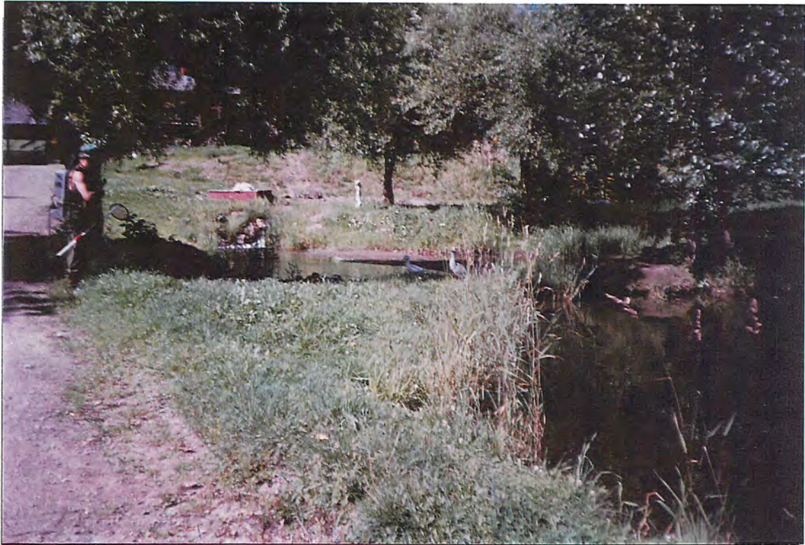
Photo #: W-G-9, 13-Aug-97 Site #: W175, Looking at a pond diversion
