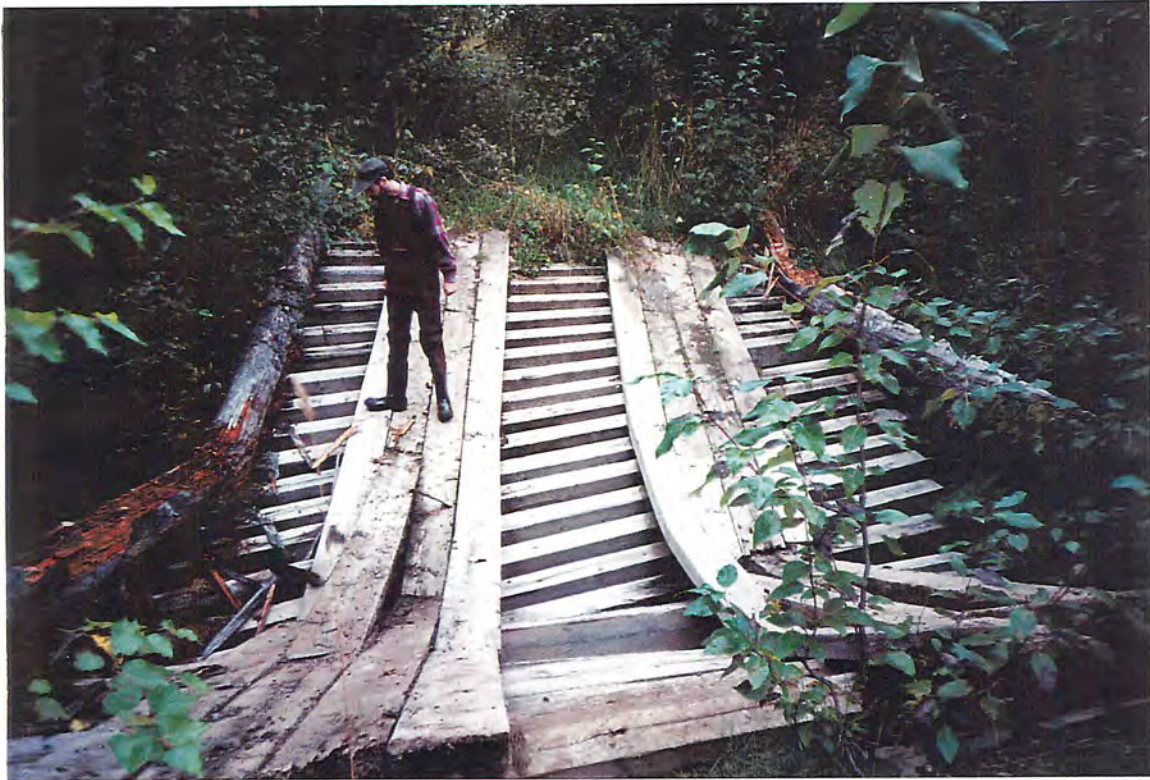
Photo #: W-M-20, 05-Sep-97 Site #: W230, Looking across stream at a collapsed bridge
