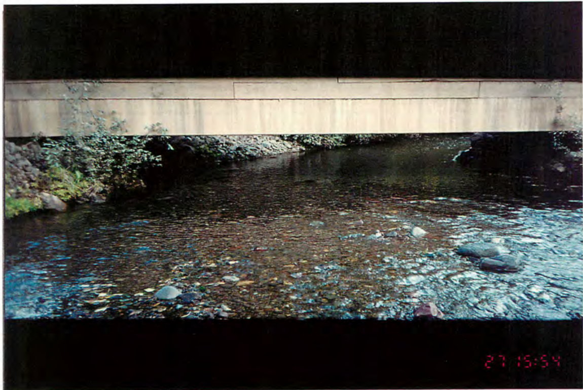
Photo #: K-6-10, 1996/09/27 Site #: K62, Looking upstream toward bridge.
