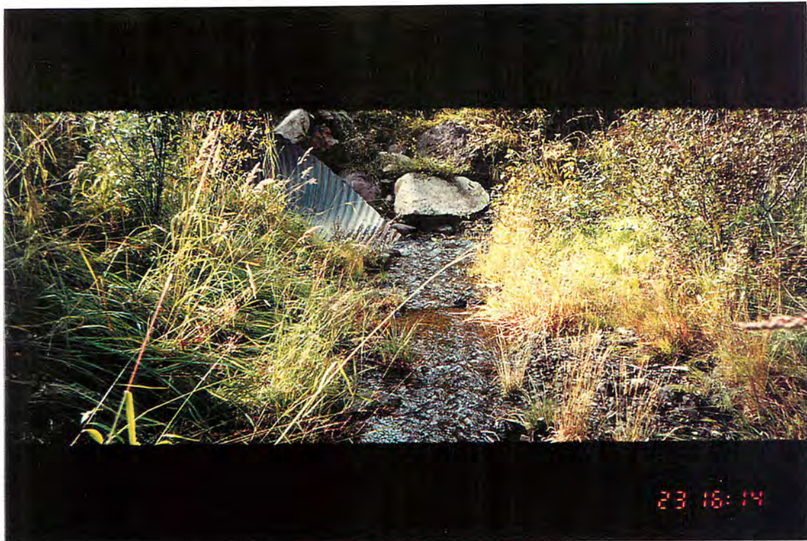
Photo #: K-3-13, 1996/09/23 Site #: K30, Looking downstream toward culvert.
