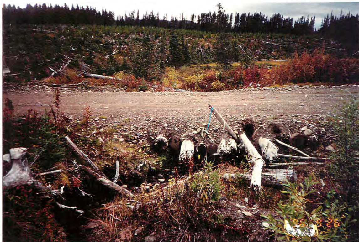
Photo #: A-5-5, 26-Sep-96 Site #: A45, Looking downstream at road crossing.
