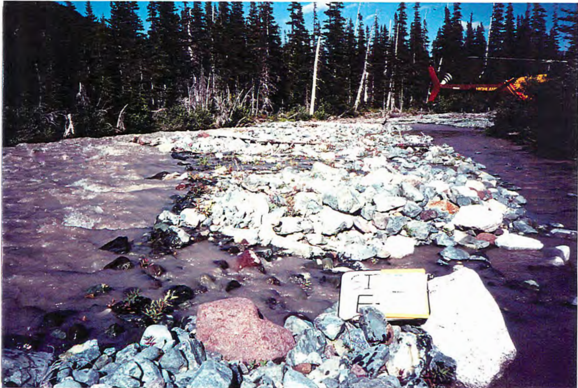
Photo #: E-18-25, 13-Aug-97 Site #: E191, Looking downstream at the channel
