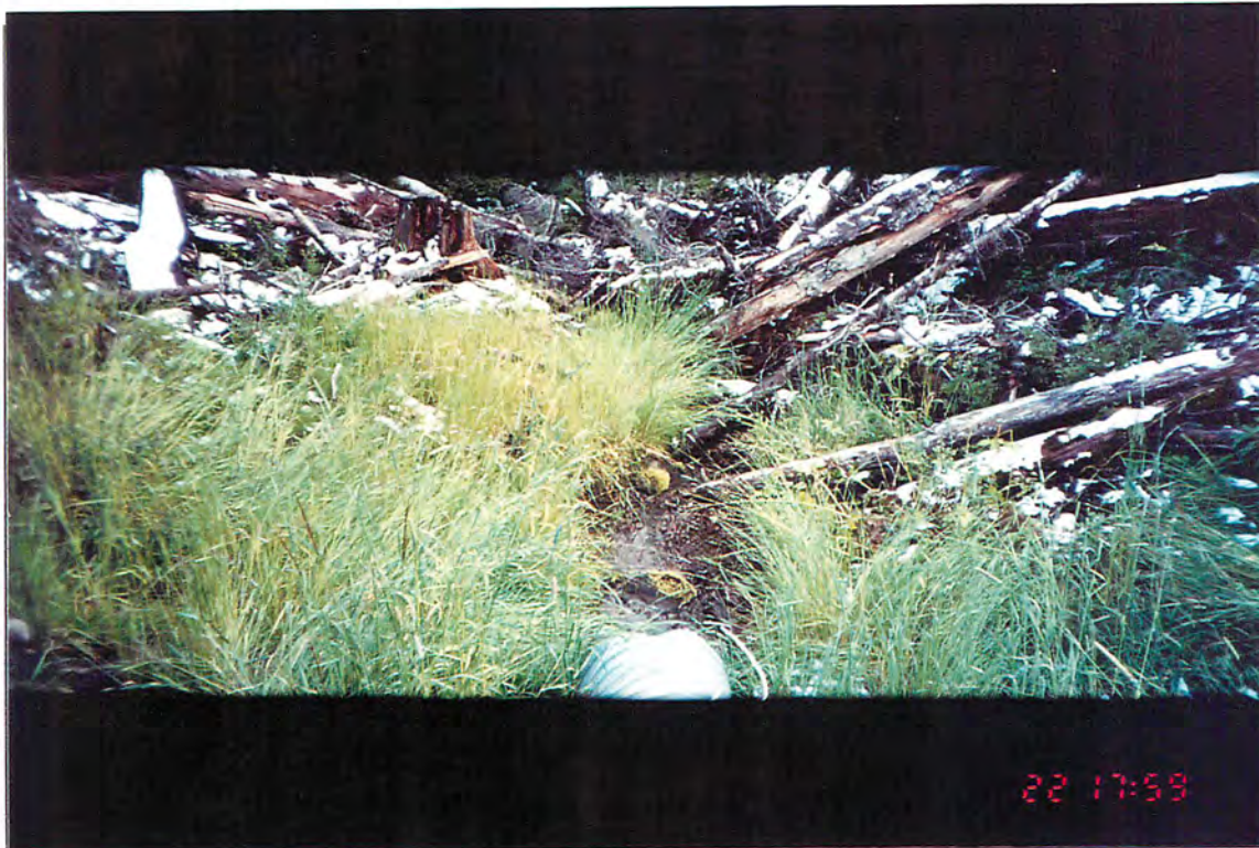
Photo #: K-3-1, 1996/09/22 Site #: K25, Looking downstream from culvert.
