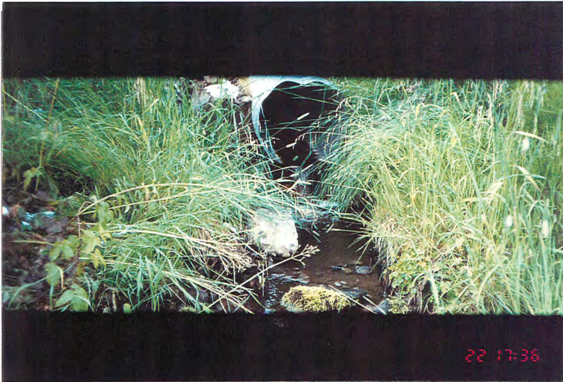
Photo #: K-2-25, 1996/09/22 Site #: K25, Looking upstream toward culvert.
