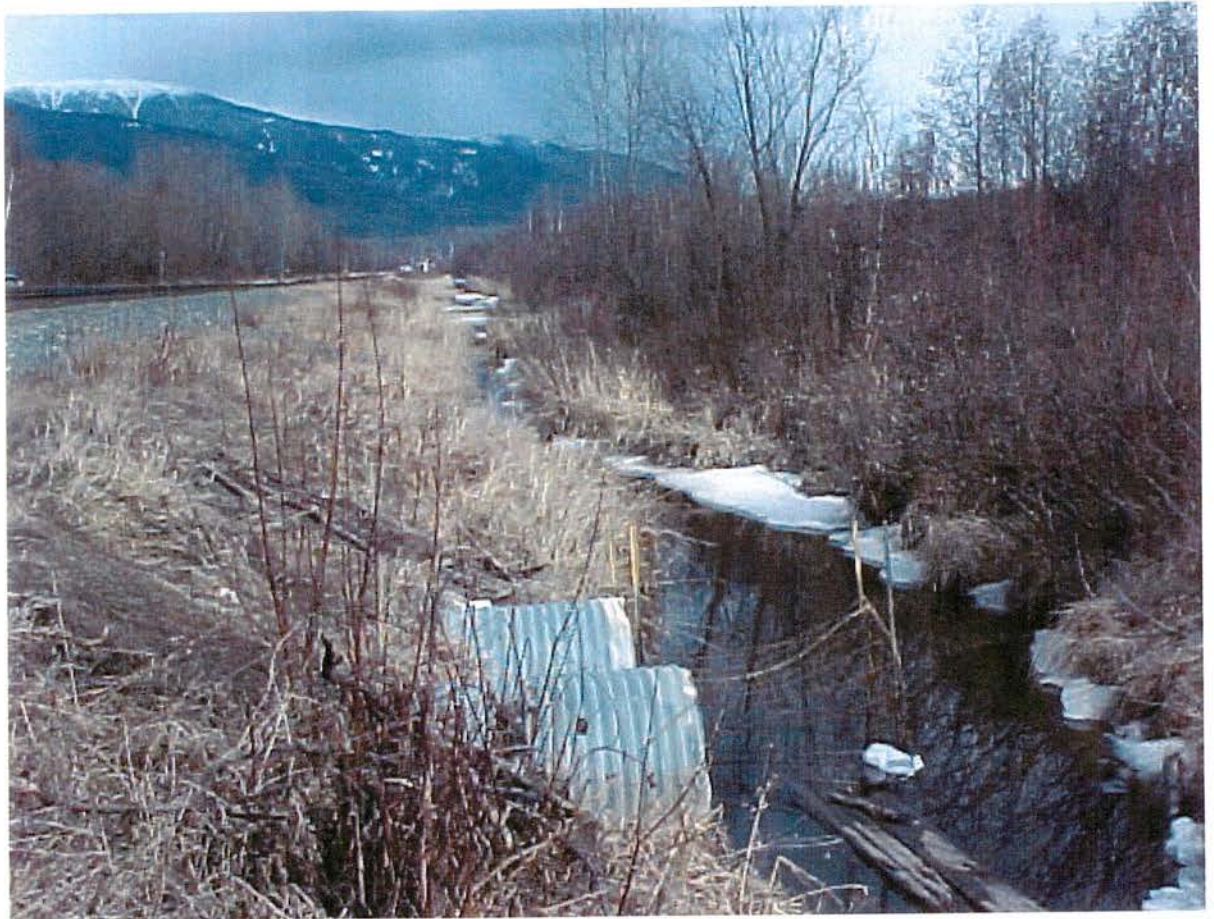
Above: Site 4 View from culverts under CN tracks, looking upstream.
