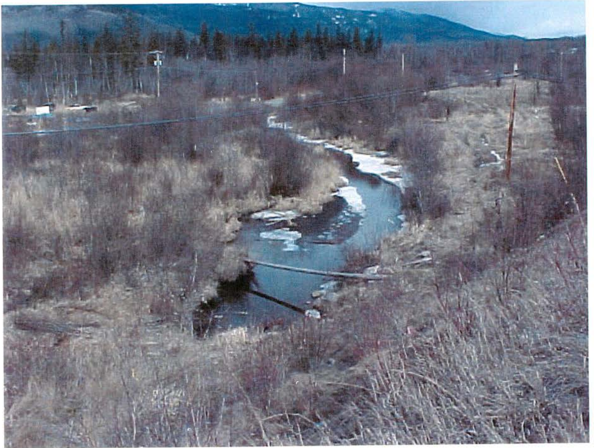
Above: Site 3 Viewed from Highway 16, looking upstream.
