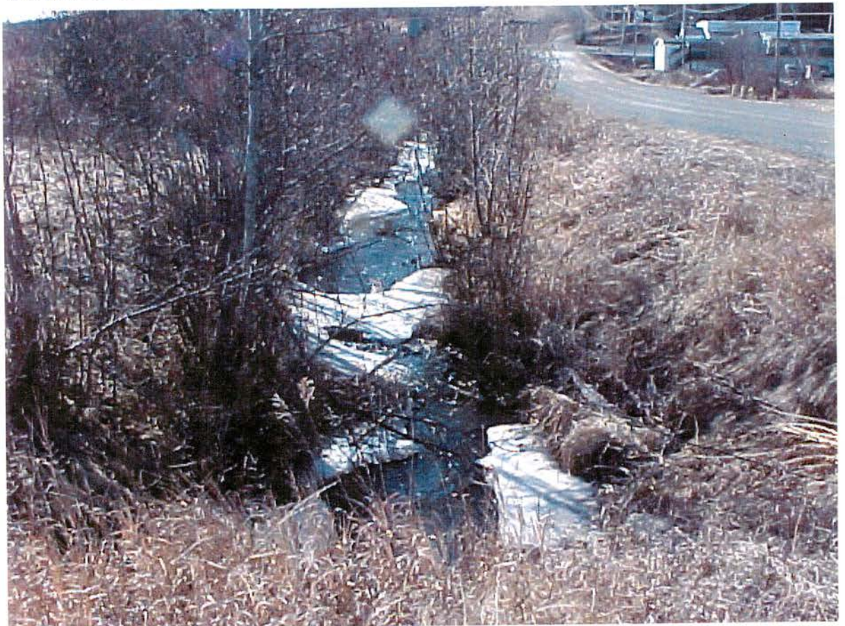
Below: Site 3 Viewed from culverts to be retained, looking downstream.
