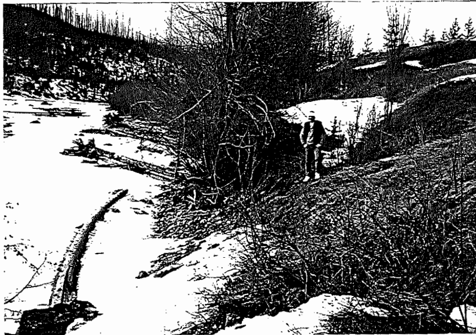
Photo 2. This small rotational failure is located at Km 23 of the Morice River. Rip rap is proposed for approximately 60 m along this section. The adjacent channel is dry during the low flow March period.
