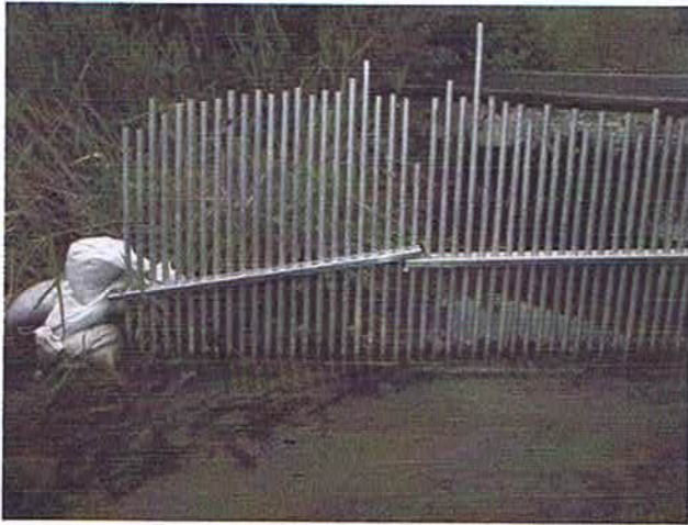
Photograph 3. Downstream fence segment to bank join blocked with sand bags.
