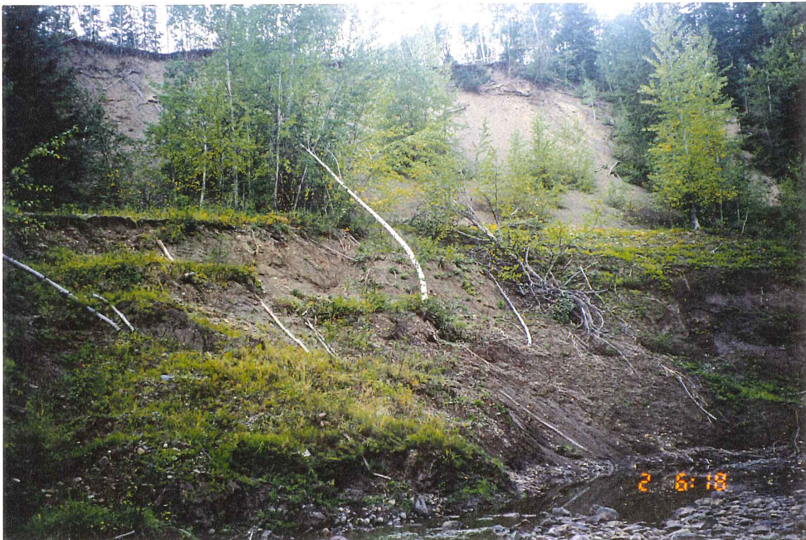
Plate 40: Large slump at the Reach \frac{1}{2} break of Richfield Creek. Note the numerous active blocks below the bottom slide scarp. Cattle use the benches of this slide for passage across and down to the waterline.
