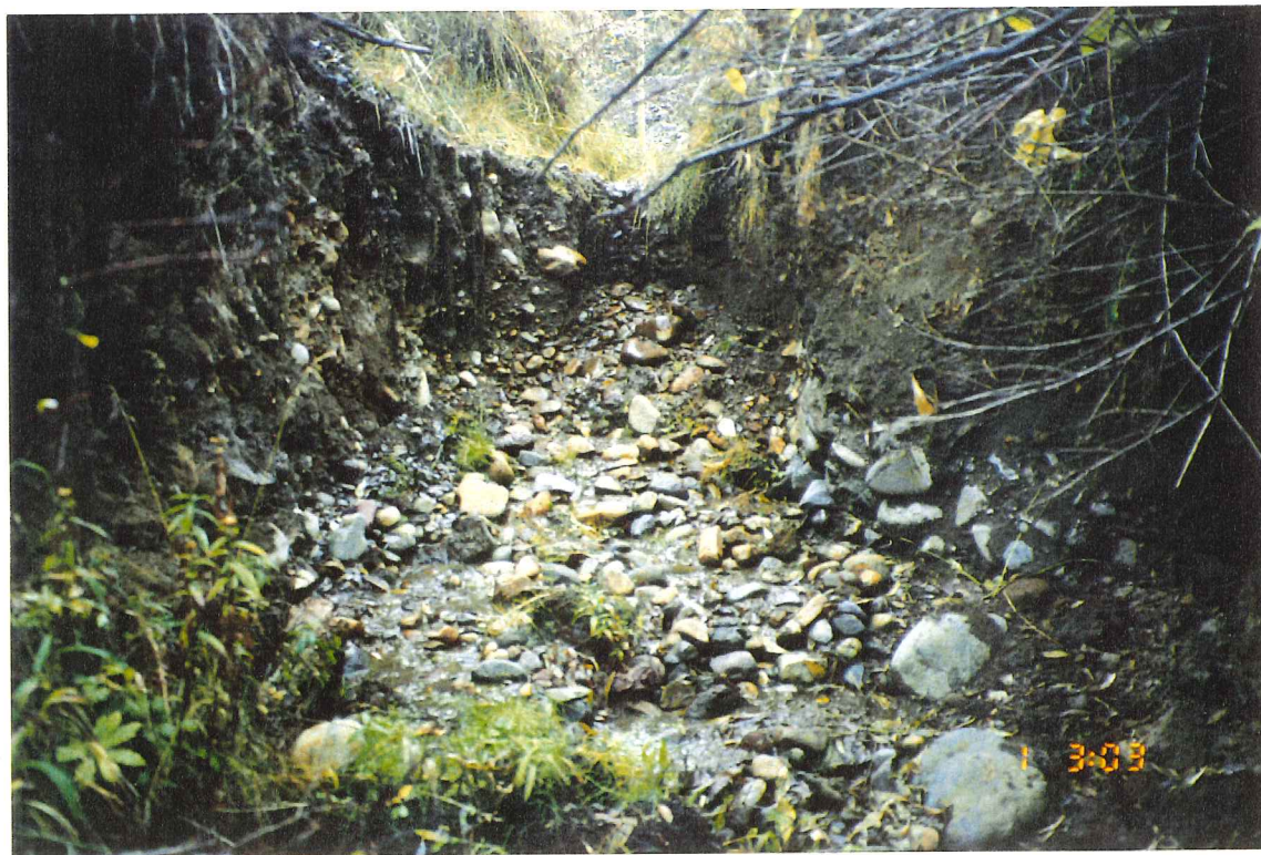
Plate 32: Failing crossditch line on FSR delivering sediment to Upper Buck Creek, Reach 11B.
