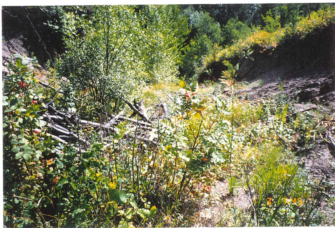
Plate 34: Large mass movement from the farm road upslope of Dungate Creek, Reach 1 (to the North) into the floodplain.
