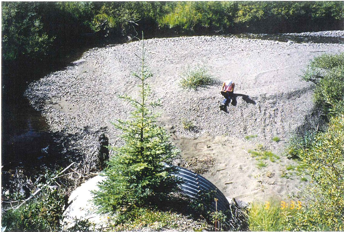
Plate 57: Aggradation above North Road FSR culvert on McQuarrie Creek. There is good fish habitat and minimal land-use from here to McQuarrie Lake provided that no barriers exist in the upstream canyon.
