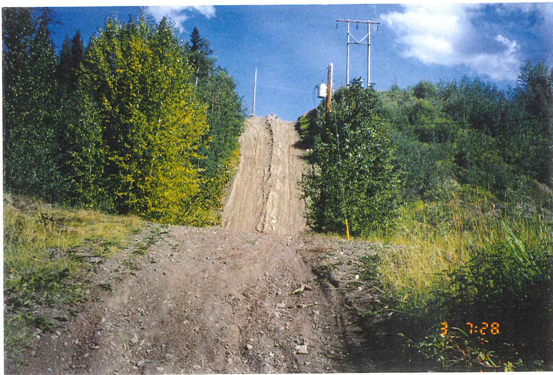
Plate 22: Powerline access road in Reach 2, Buck Creek, eroding due to concentration of runoff. An external source of fine sediment.
