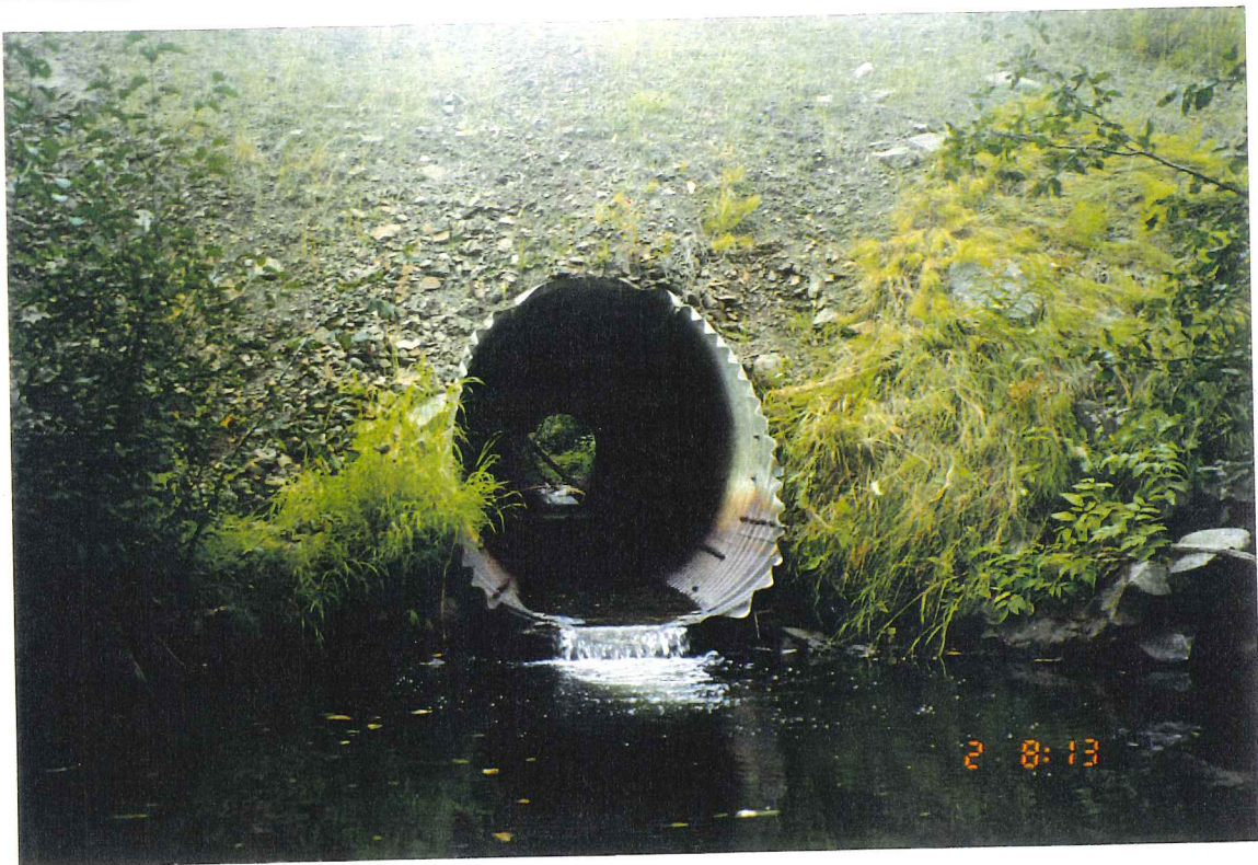
Plate 47: Highway culvert on Johnny David Creek. This culvert does not appear to be a barrier due to gradient and height of inlet/outlet above the channel surface. It may be impassable due to water velocities at higher flows and water levels at low flows. Photo taken at low flows.
