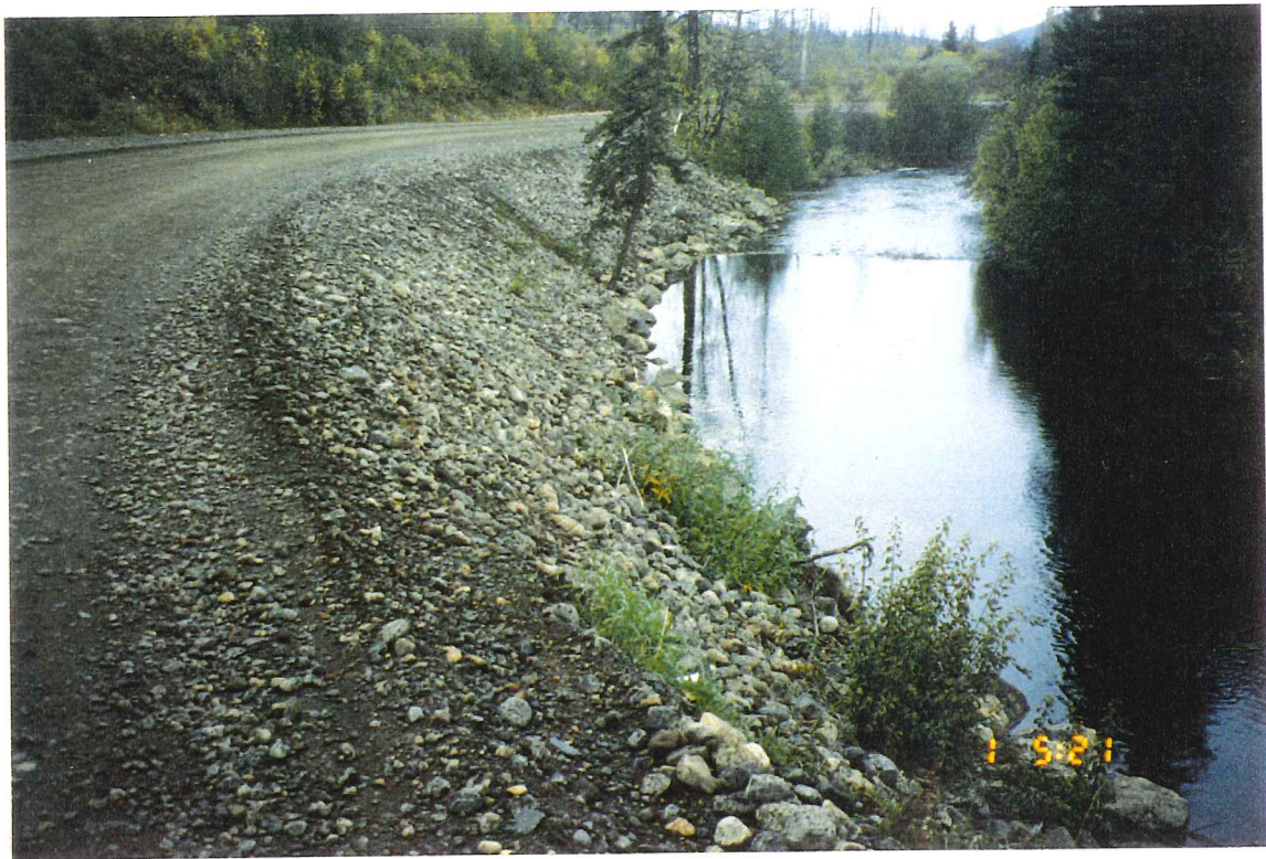
Plate 27: Extensive rip-rapped section of Reach 6, Buck Creek along the Buck Flats road.
