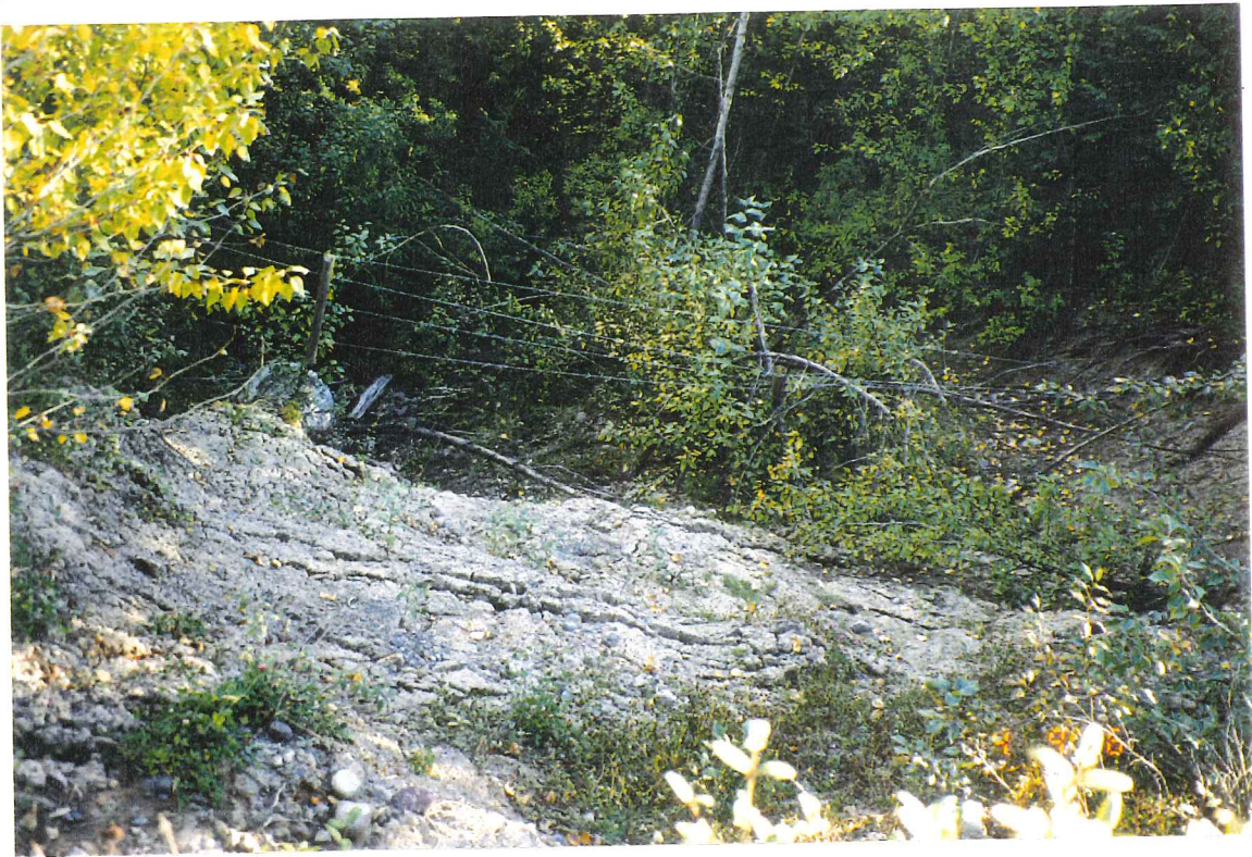
Plate 3: Large rotational clay slump at the Michelle Bay FSR. Occurred at a culvert for a small intermittent unnamed creek and was likely caused by the geotechnical and/or hydraulic failure of the fine-textured fill.
