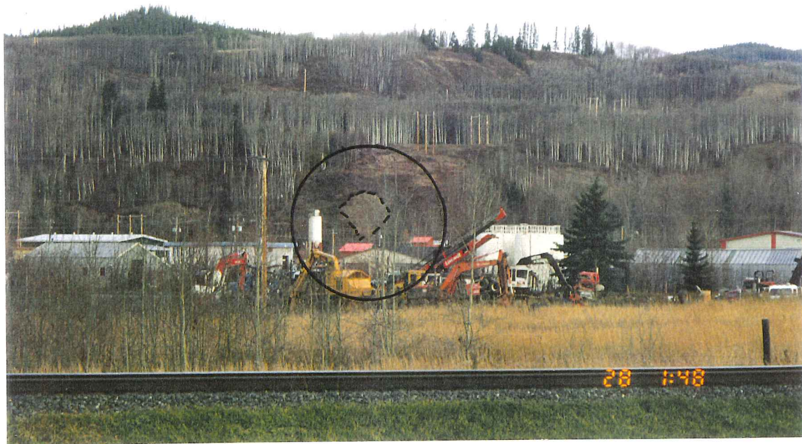
Plate 6: Powerline crossing of Bulkley River at Houston showing an actively eroding section on the cleared slope.
