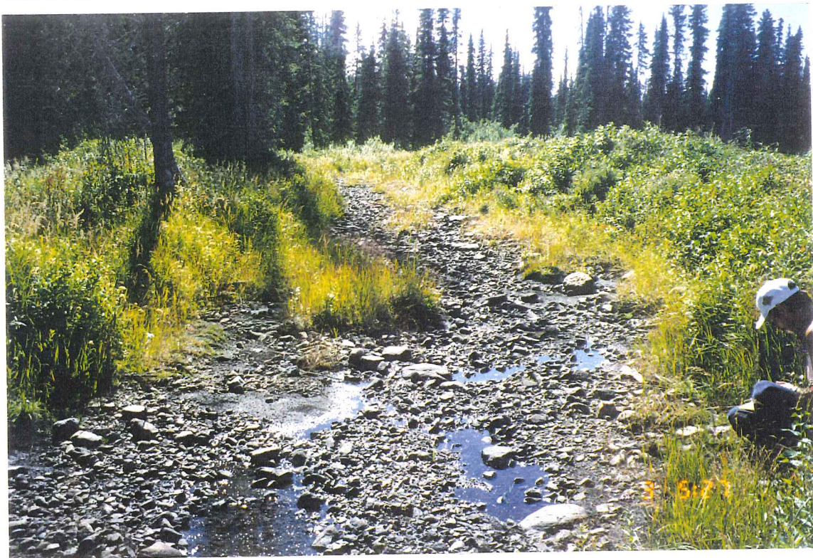
Plate 45: Eroding fire break at clearcut in the headwaters of Robert Hatch Creek which delivers sediment into a wetland area behind a beaver dam. The water running over this fire break is Robert Hatch Creek.
