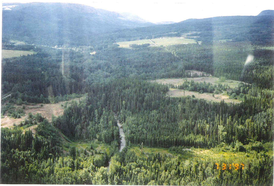
Plate 20: Reach 2 of Buck Creek, showing powerline crossing and gravel quarries. The right-of-way is eroding from runoff being concentrated down the road to the creek crossing (to the left of the photo).
