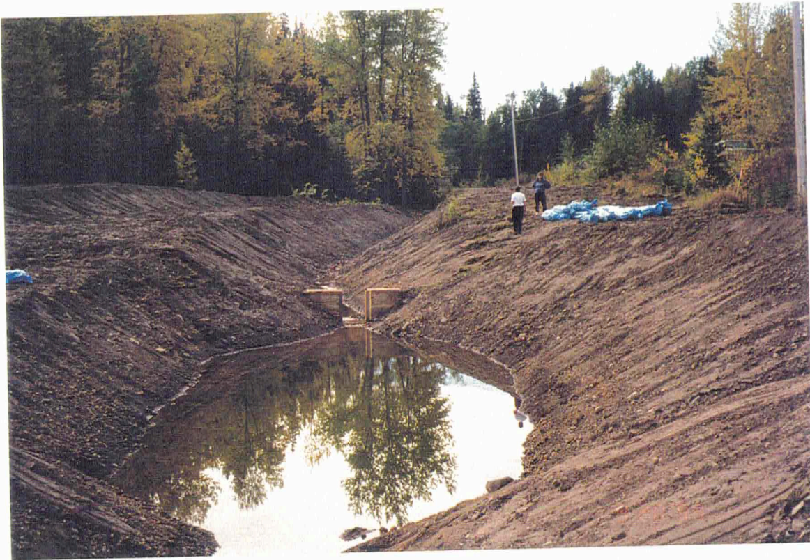
Seeding and Installation of Biomats
