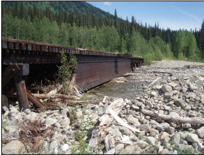
Figure 1. Downstream side view across Azuklotz Creek Bridge showing 10 cm clearance between the bridge span and the stream surface.
