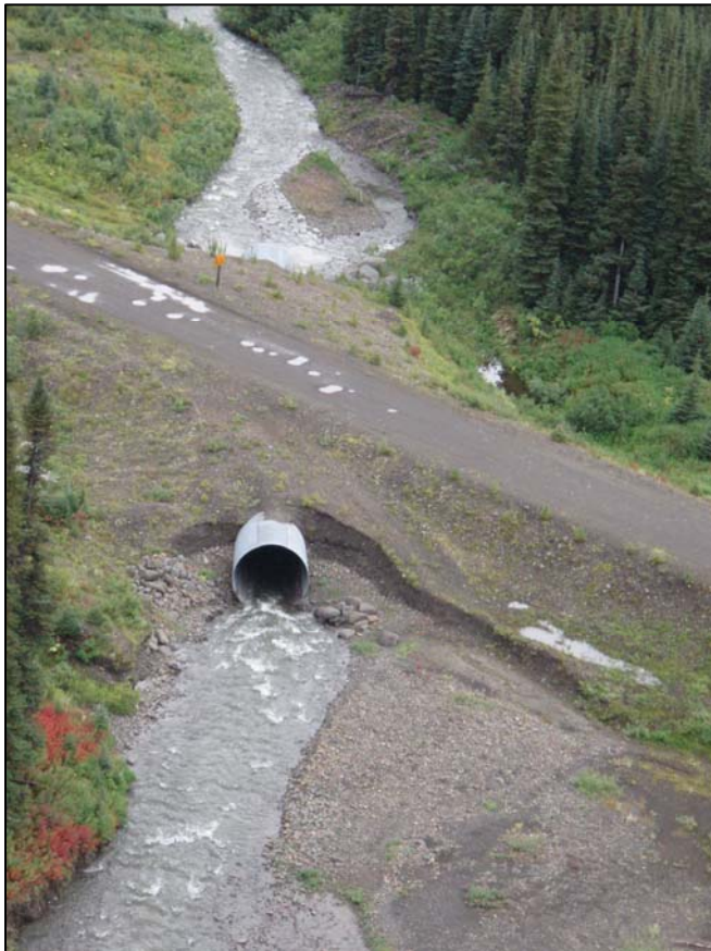
Figure 57. View downstream to Garner Creek crossing.
