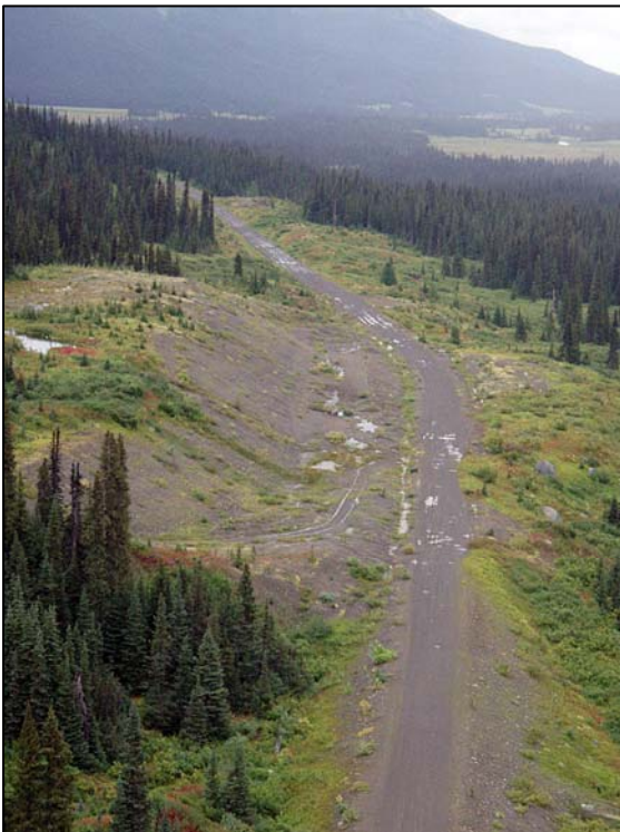
Figure 37. Cutslope showing limited vegetation after three decades of recovery.
