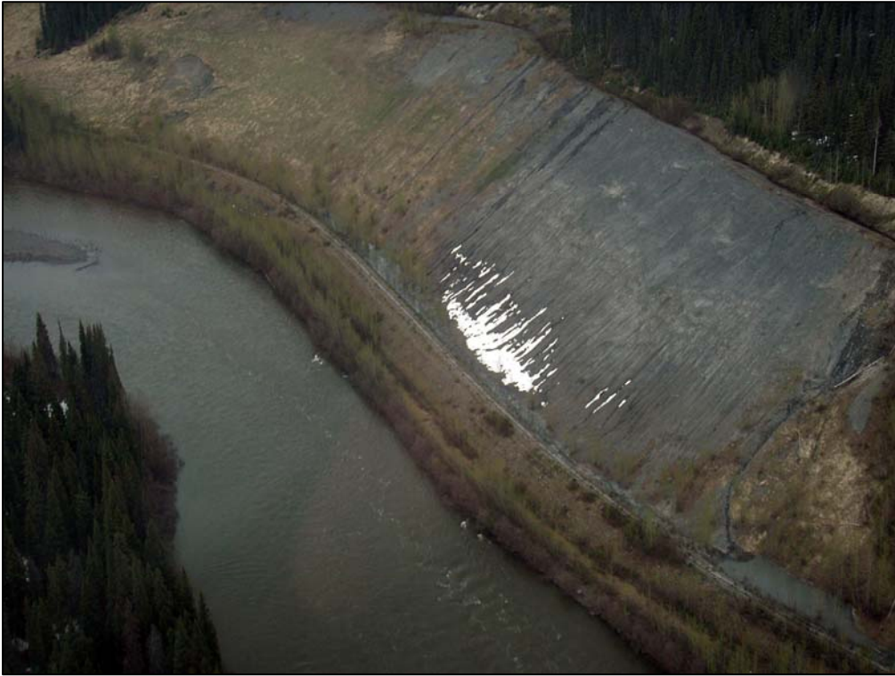
Figure 34. Cutslope upstream of Mosque River, 2007.
