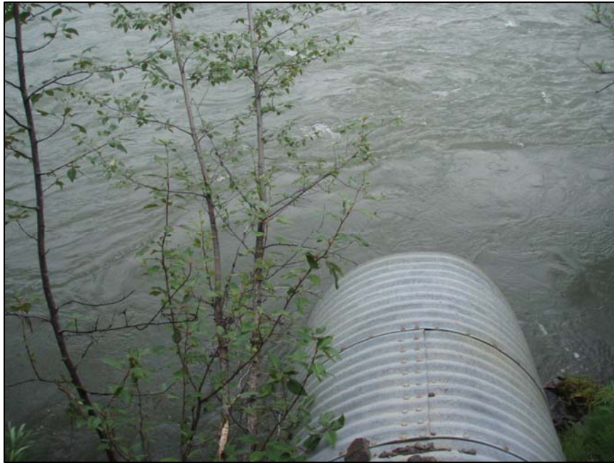
Figure 47. Site 21, view downstream from culvert outlet.
