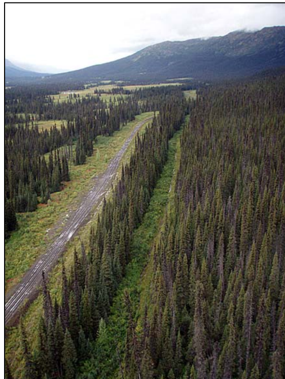
Figure 38. Drainage ditch intercepts surface and concentrates stream flows.
