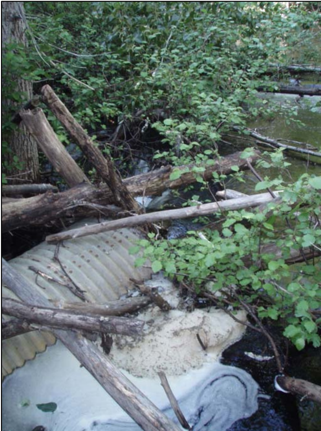
Figure 56. View upstream of partially blocked south culvert inlet.
