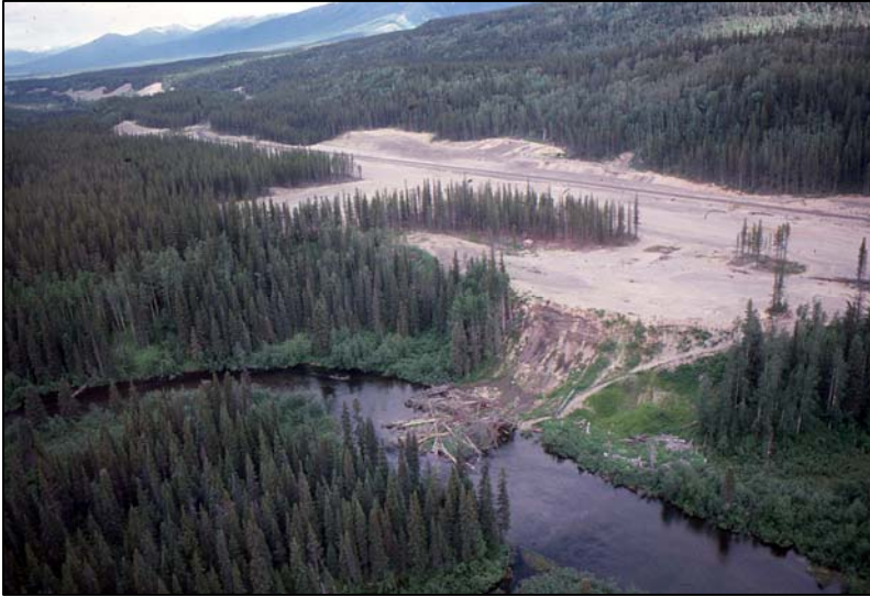
Figure 30. Slide into the Bear River, July 1977.
