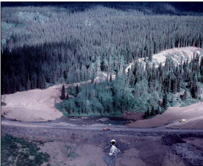
Figure 29. View to Bear River tributary culvert installation, August 1974.
