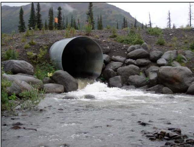
Figure 60. View upstream to culvert outlet.
