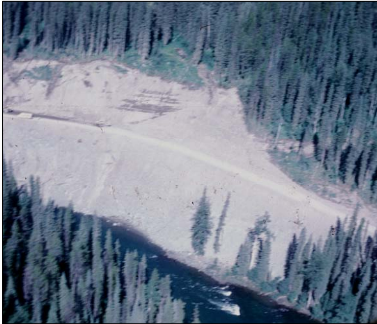
Figure 26. Chronic fill slope slide into Bear River, August 1974.
