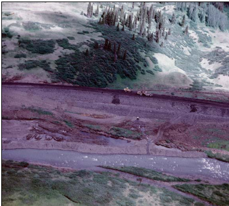
Figure 27. Sediment and waste earth into Bear River, August 1974.
