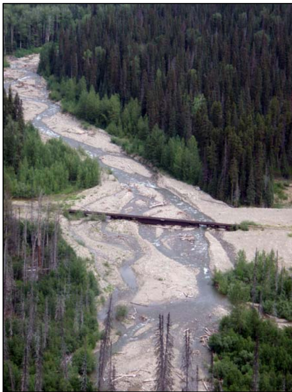
Figure 40. Azuklotz Creek and the rail bridge.
