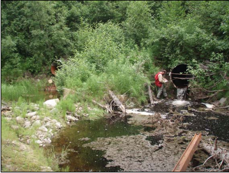
Figure 43. Site 3, view upstream to culvert outlet.
