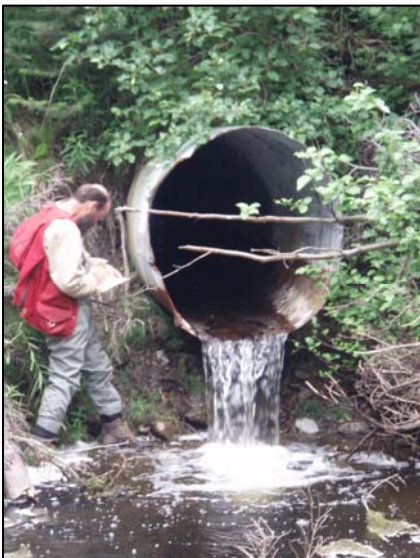
Figure 45. Site 3, view upstream to culvert inlet.
