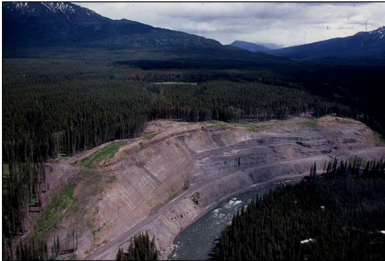
Figure 32. Extensive rockcut ~3 km upstream from Birdflat Creek, July 1977.
