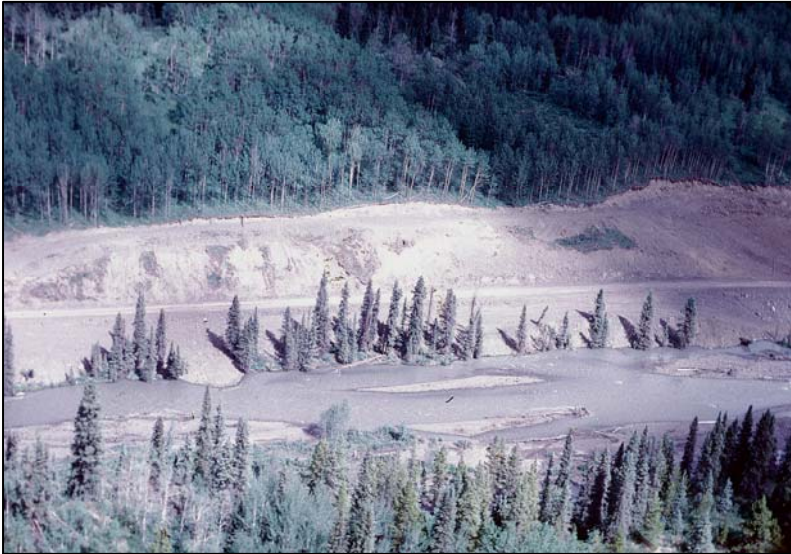
Figure 28. Photo shows Bear River with fill and waste soil encroaching on the channel, 1974.
