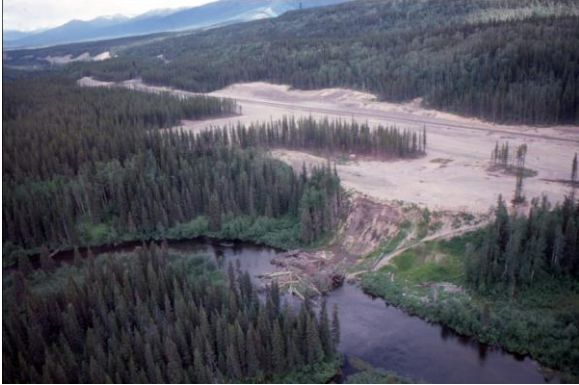
Slide into Bear River chinook spawning habitat from BC Rail construction
