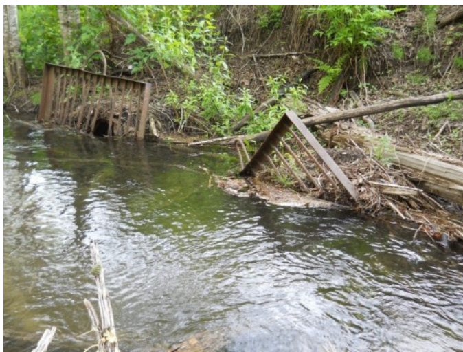
Figure 8b. This site, located along a public road (Old Lakelse Lake Road) and ~ 100 meters from site W-0437, is also a 3rd order stream with beaver/debris guards. Although not assessed, it is another example of problematic beaver guarding impeding or blocking fish access.
