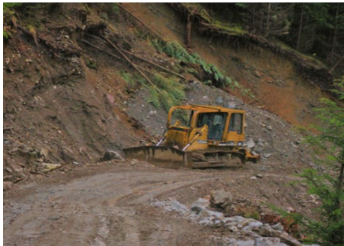
Figure 10. Recently constructed spur with active hauling. Site had poor water management and high road-related sediment generation, which was compounded by over-steepened cutslopes.
