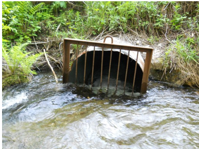
Figure 8a. Site W-0437, located along a public road (Old Lakelse Lake Road), and a 3rd order stream with beaver/debris guard was assessed to be a significant fish barrier. Issues included: undersized culvert restricting channel, velocity barrier, and outlet and inlet drops.
