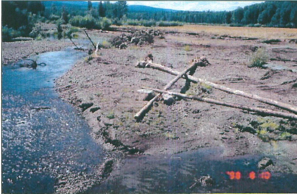
Figure 4: Site 6 - Bar Stabilization Structure
