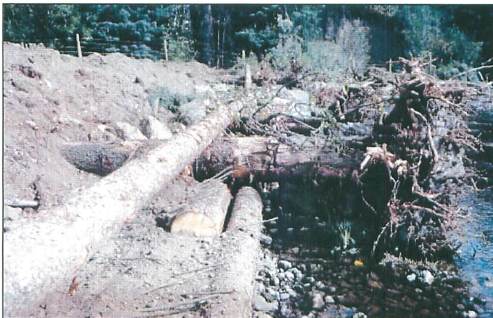
Figure 2: Site 1 - LWD Revetment
