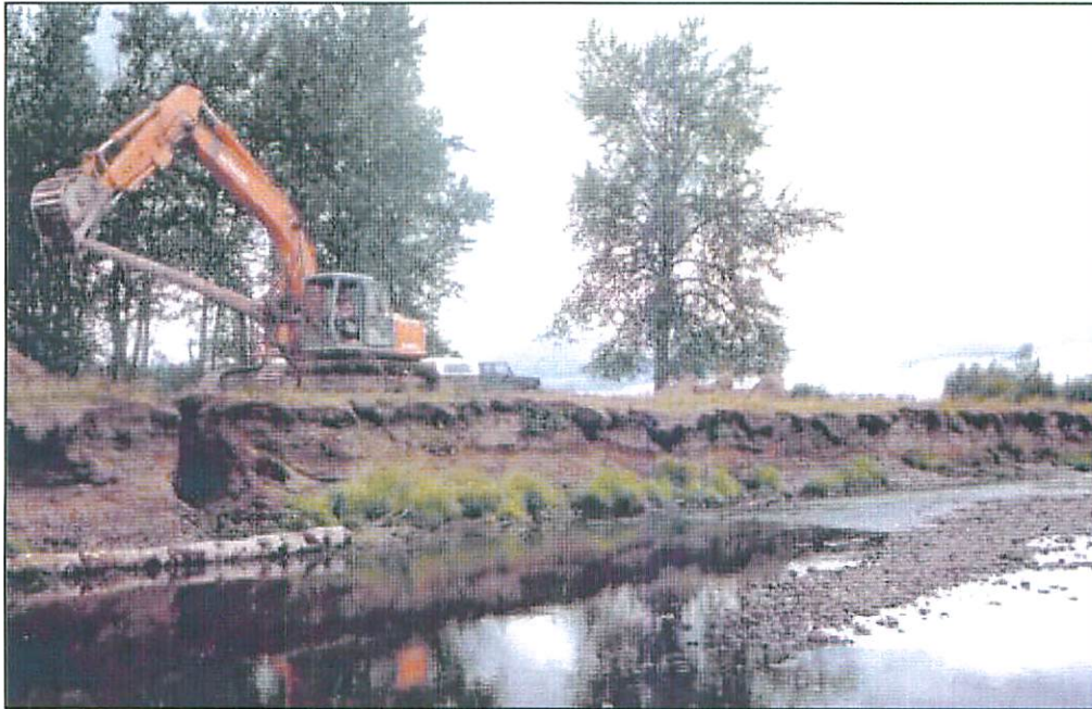
Figure 1: Site 1 - Placing LWD
