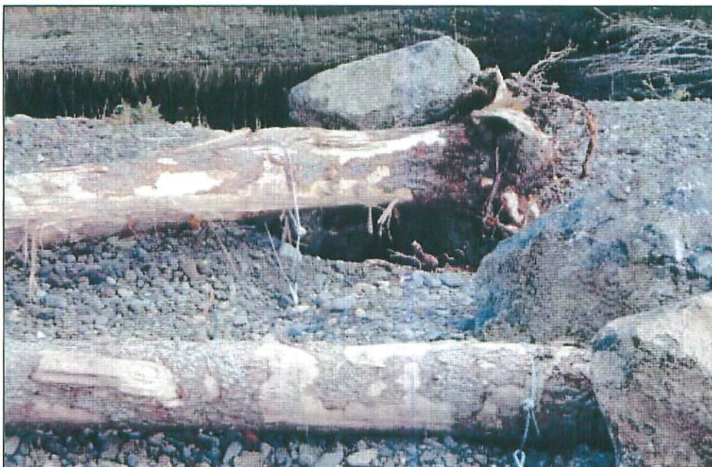
Figure 5: Site 6 - Anchoring for Bar Stabilization Structures
